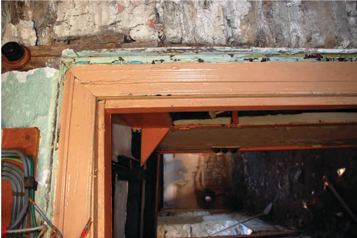
Plate 22 Doorcase of kitchen doorway, assembled from two or more Phase 3 doorcases, looking SE.
