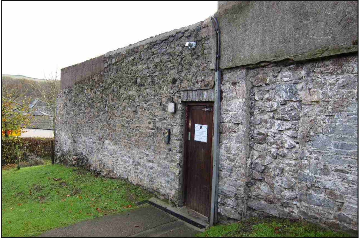
Photo. 5 The north boundary wall of the school and convent grounds, showing the blocked doorway and area of protecting stone build (site 3). Looking east.
