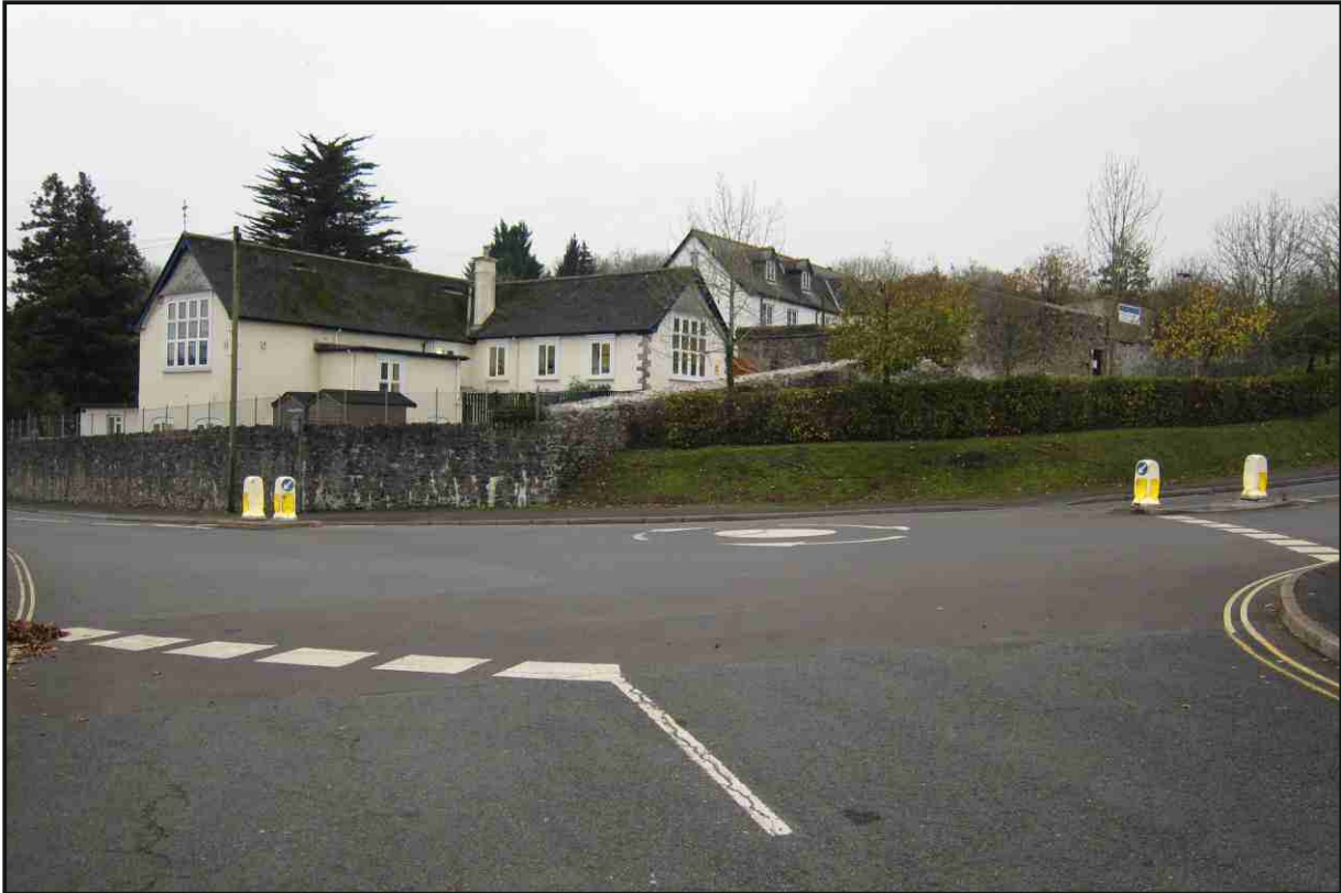
Photo. 1 The assessment site, looking south-west, with the convent on higher ground to the rear of the school.
