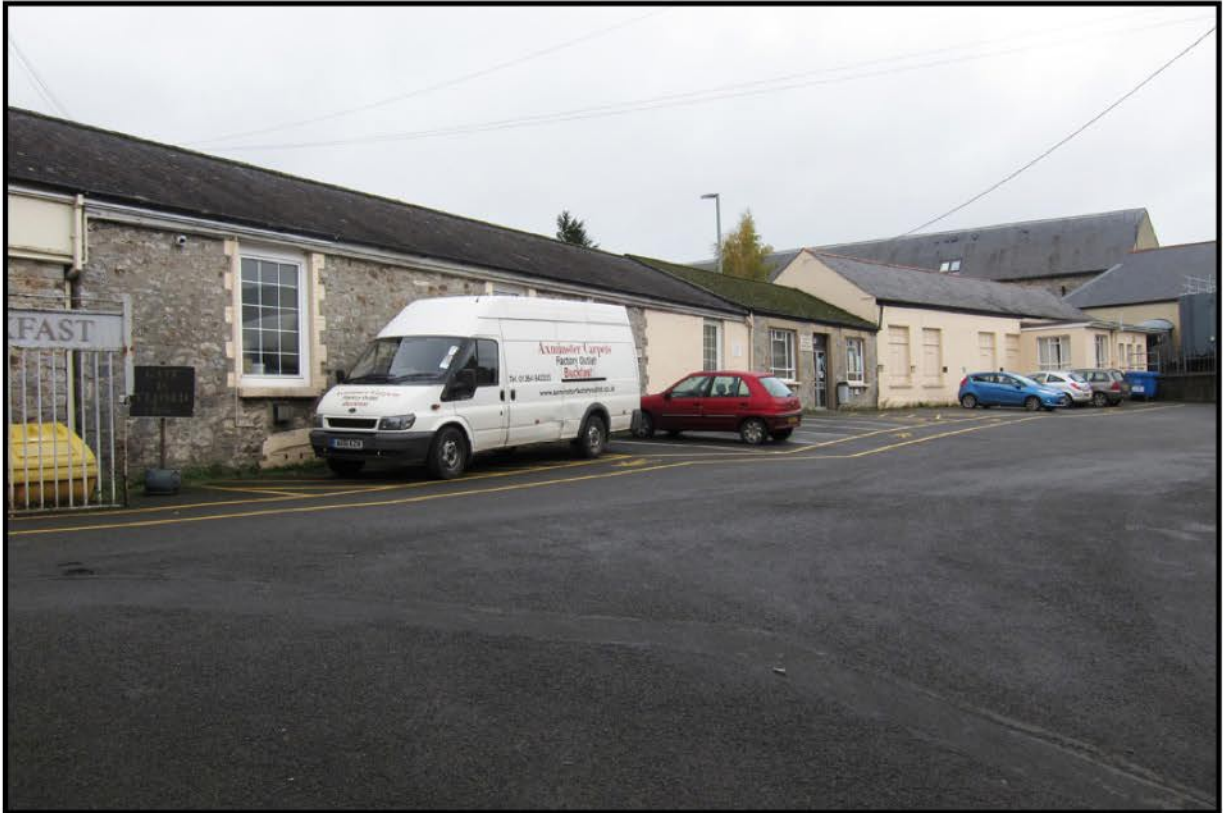
Photo. 7 The western range (Building D), looking north-west. The roof to Building B is visible at the far right. Later elements include the southern tip (to the left, and behind the gate) and a section of infilling (abutting the cream painted northern section).
