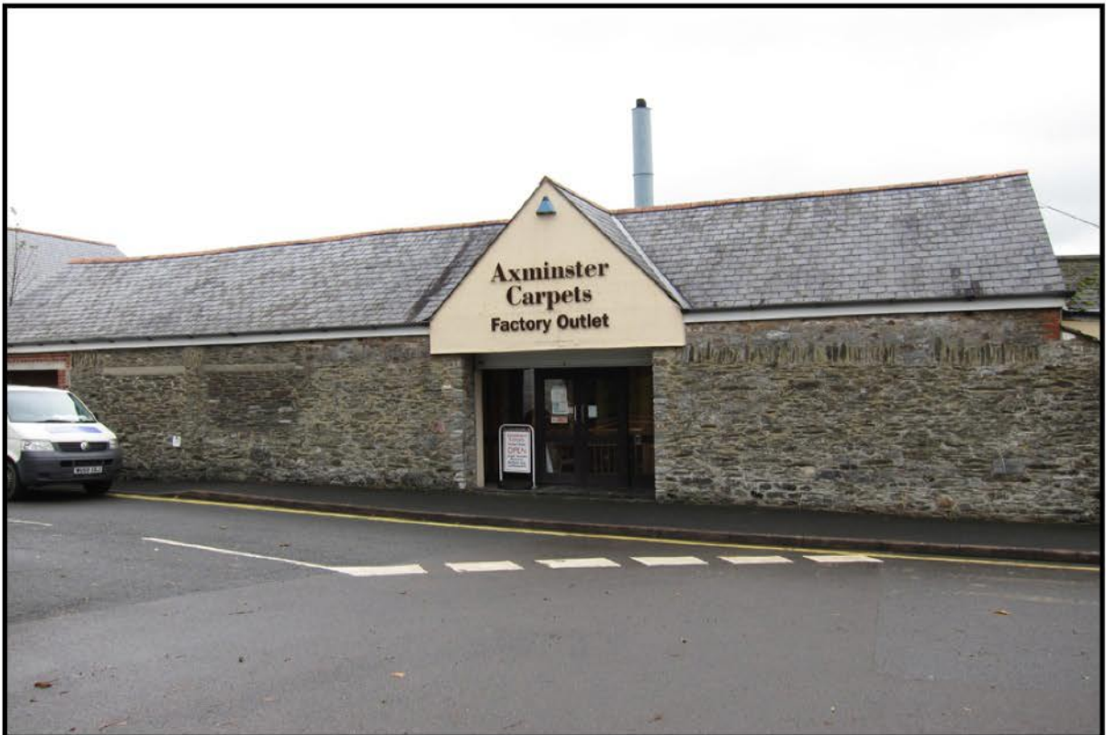
Photo. 8 The west elevation to the northern part of Building D, seen from the road. The capping to an incorporated boundary wall, and blocked openings, are visible.
