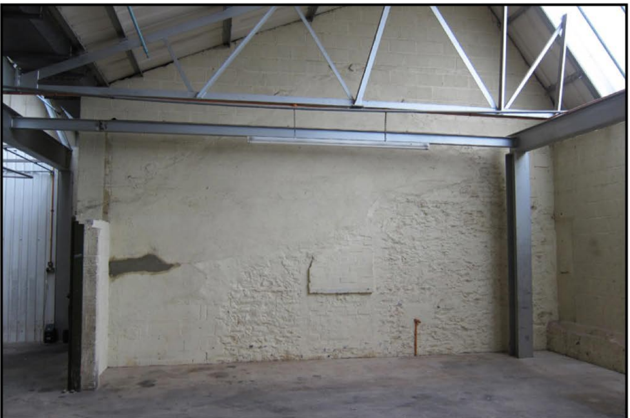
Photo. 14 What was once the eastern external elevation to the partial nineteenth-century range, now enclosed within the modern southern half of Building J.
