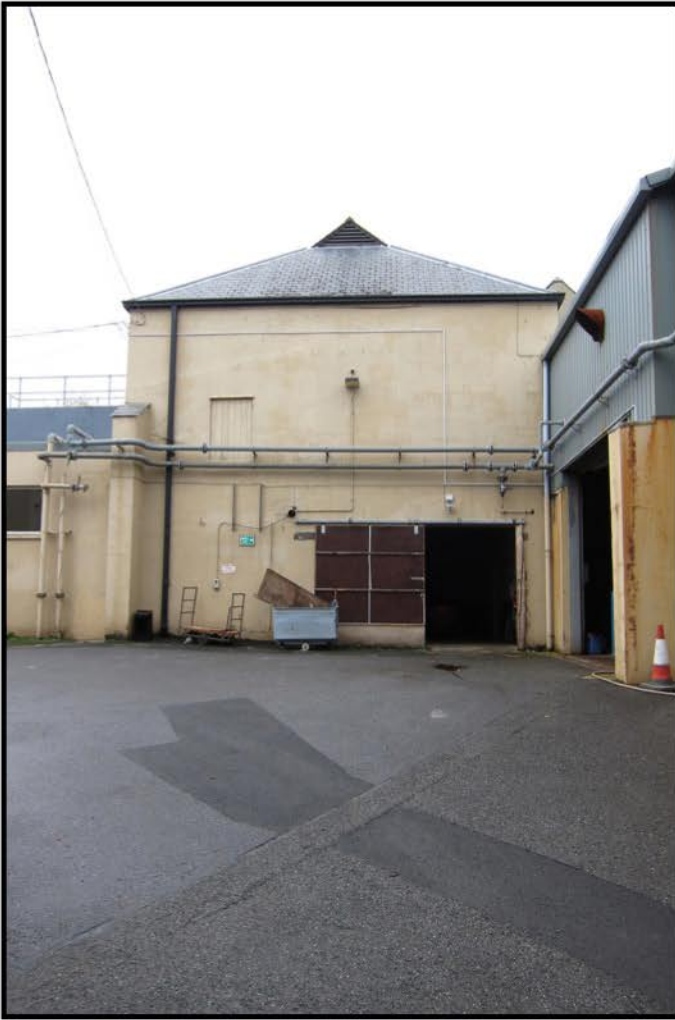
Photo. 3 The east elevation of Building B, looking west. Parts of Buildings A (to the right) and C (to the left) are also shown.
