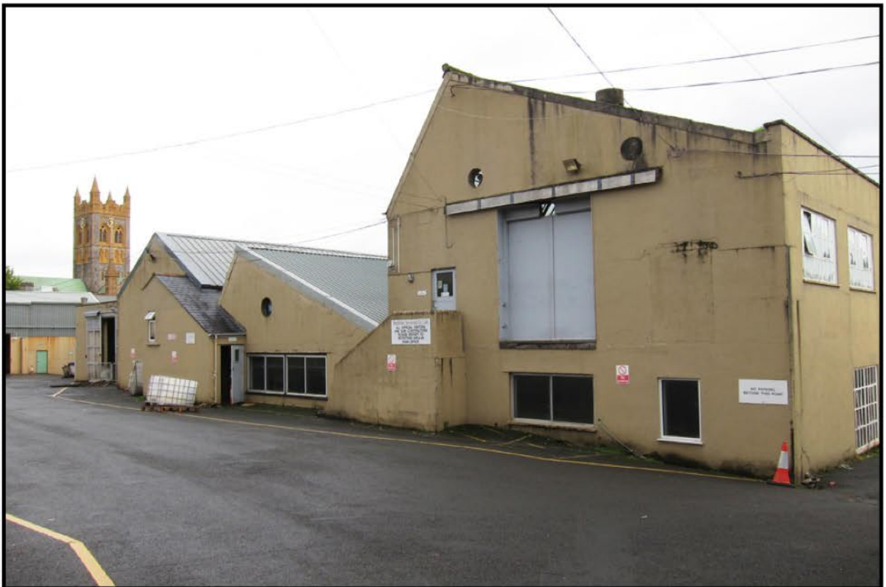
Photo. 10 The west elevation of Building J, looking north-east. The gabled roofline directly to the right of the church tower represents the only early roof structure. The flat roof below the tower covers the only range with all four surviving walls.
