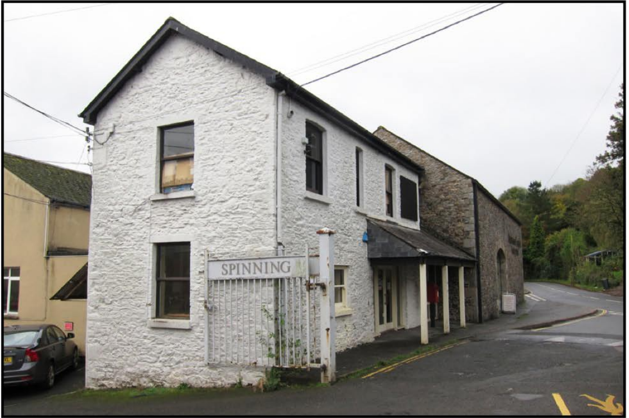
Photo. 1 Buildings E and F, looking south.
