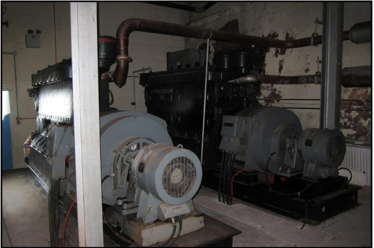
Photo. 15 Two Lister engines within the engine room in Building J. The east wall (beyond the farthest engine) may date to the early twentieth century.
