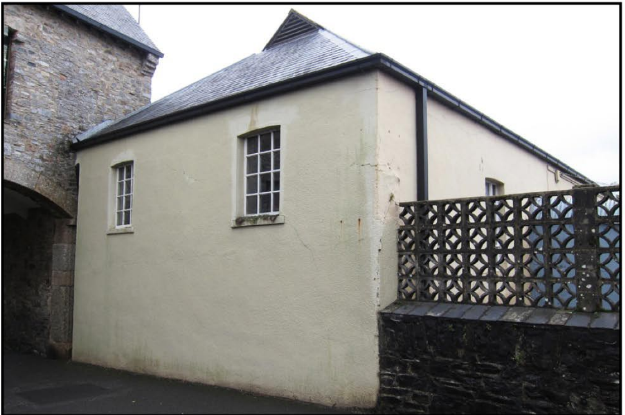
Photo. 2 The west elevation to Building 2, looking north-east.
