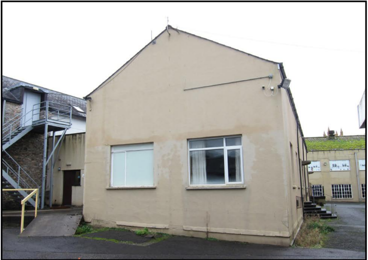
Photo. 9 The south elevation of Building G, looking north.
