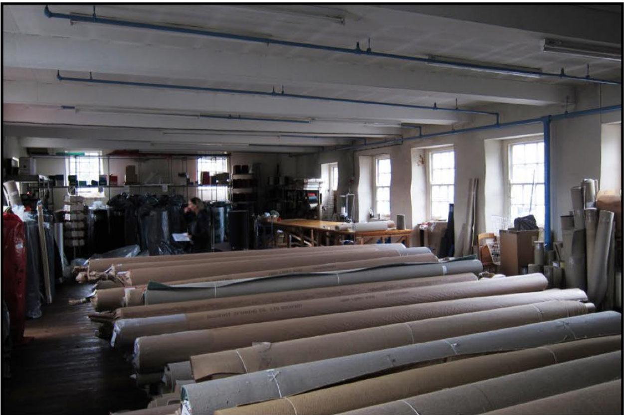
Photo. 4 The first floor of Building B, looking west.
