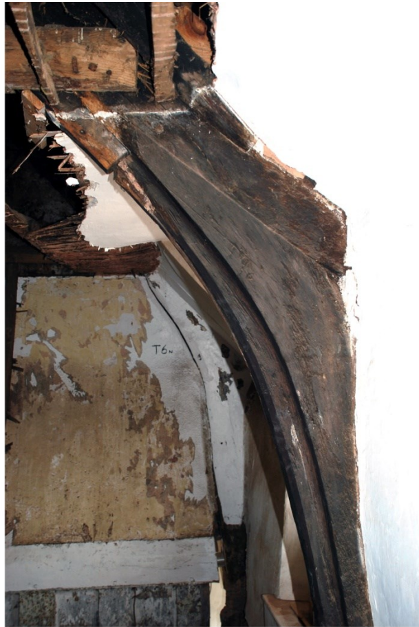
Plate 3 Elbow joint of jointed cruck truss over former kitchen, looking west.
