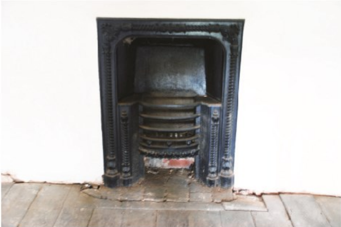
Plate 27 The first-floor 19th-century cast iron fireplace in the north wall of the lower end, looking north.
