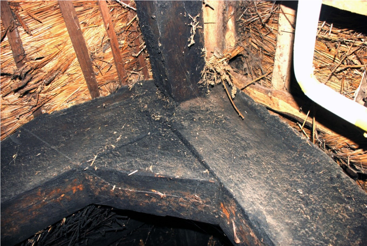
Plate 5 Triangular yoke and diagonal ridge of the medieval roof, looking west.
