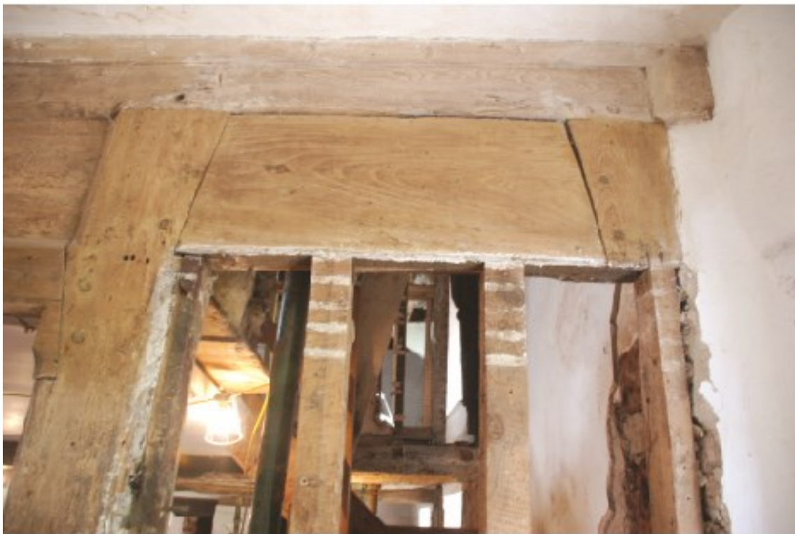
Plate 22 The door head of the stair doorway, looking east.
