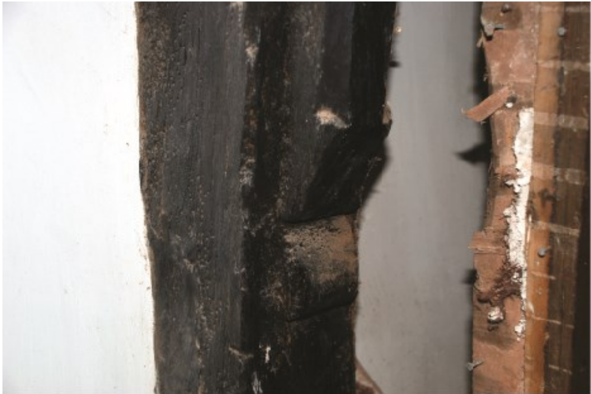
Plate 7 Decorative corbel stop at the base of the arch braces, looking northeast.
