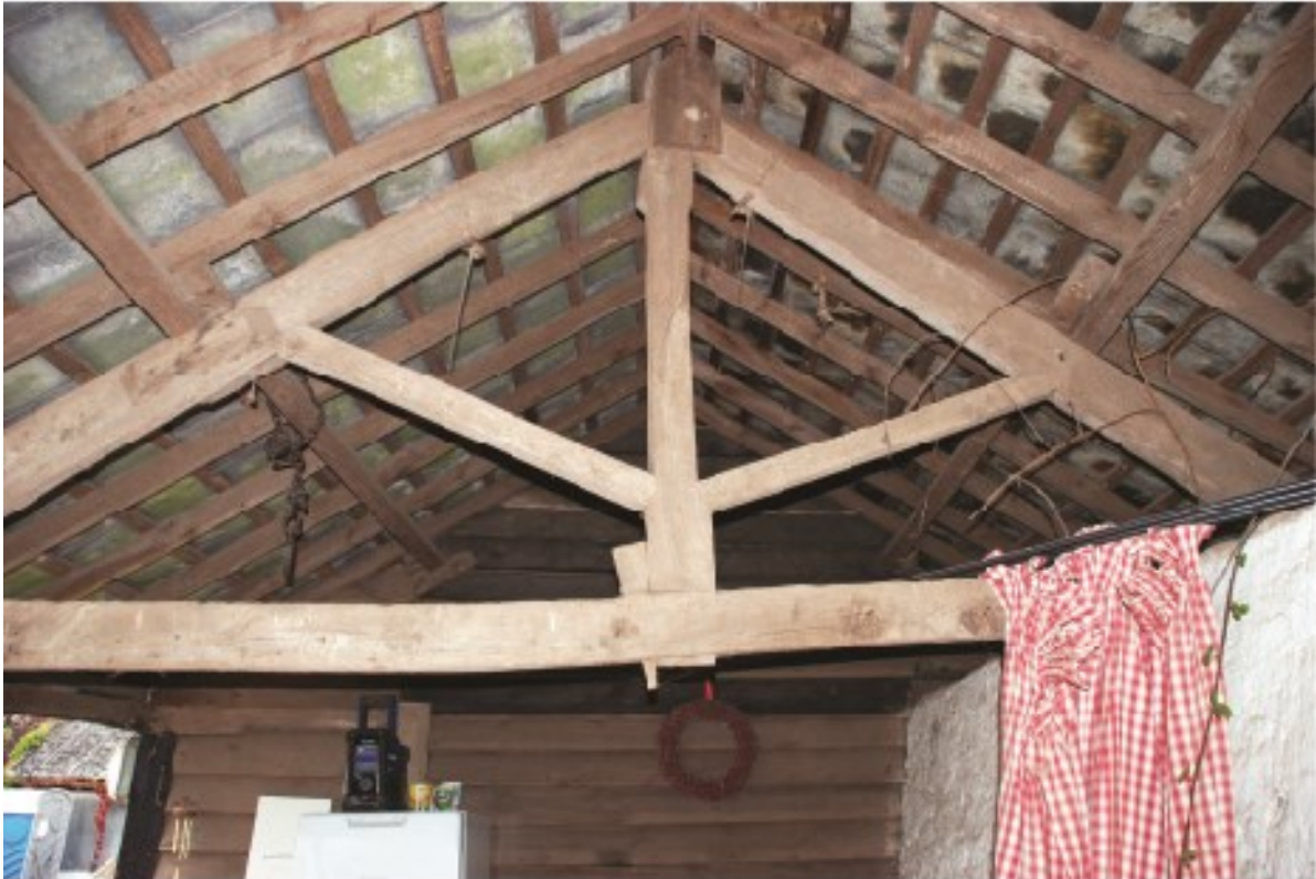
Plate 31 19th-century king-post roof over well house, looking north.
