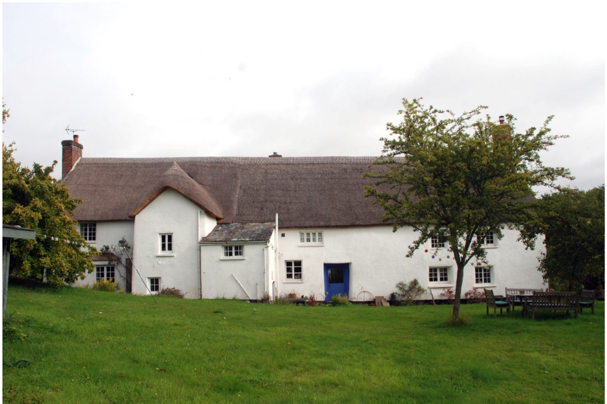
Plate 2 The rear elevation of the house, looking north.
