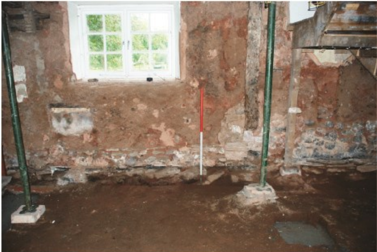
Plate 13 Trench-dug stone rubble footings exposed beneath the south wall, looking south.
