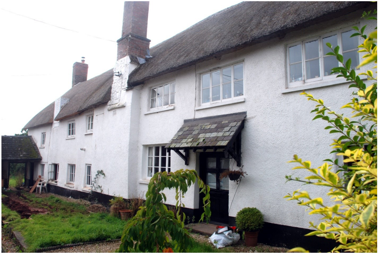
Plate 1 The front elevation of the house, looking northeast.
