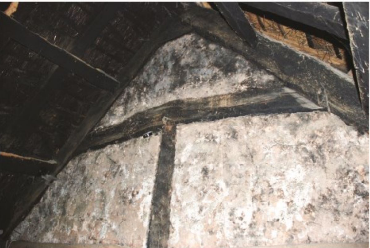
Plate 10 The full height partition between the passage and lower end, showing top rail pegged to the truss, looking southwest.
