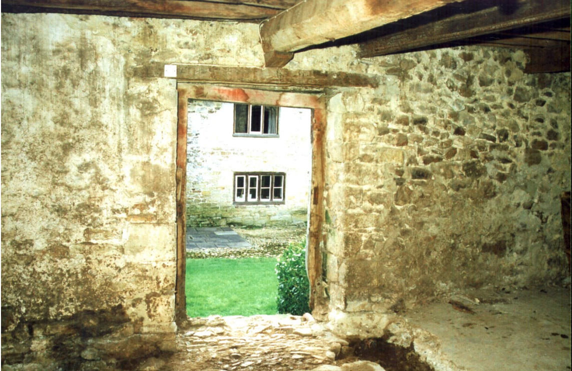
Plate 11 The easternmost doorway in the south wall, looking South.
