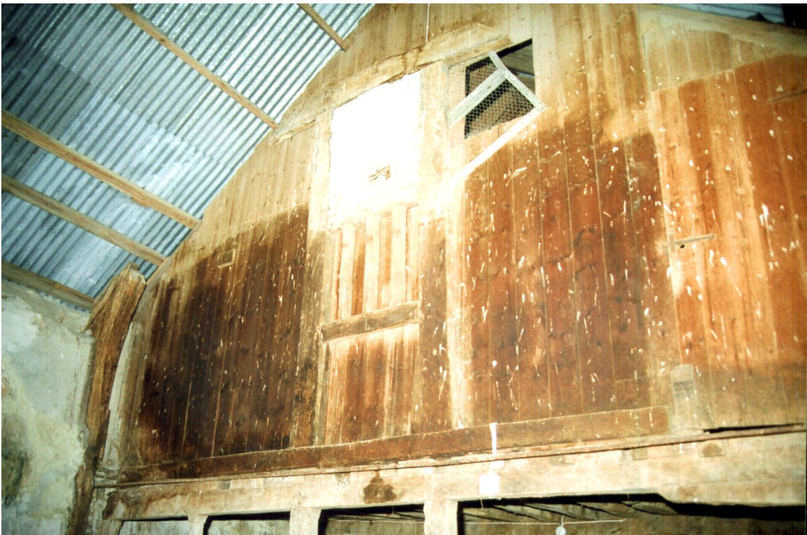
Plate 12 The late medieval timber-framed cross-wall above the screen, looking South-west.
