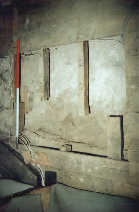
Plate 1 Trench 1, looking E
