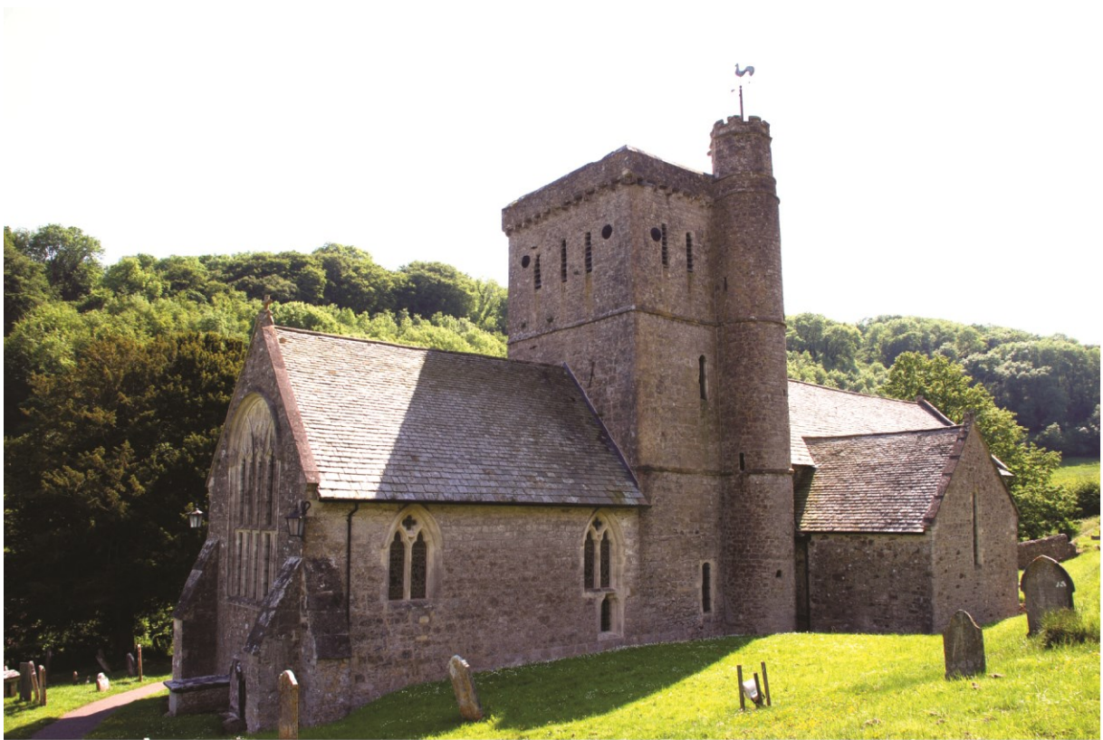
Plate 12 Branscombe church Norman tower and stair turret, looking southwest.
