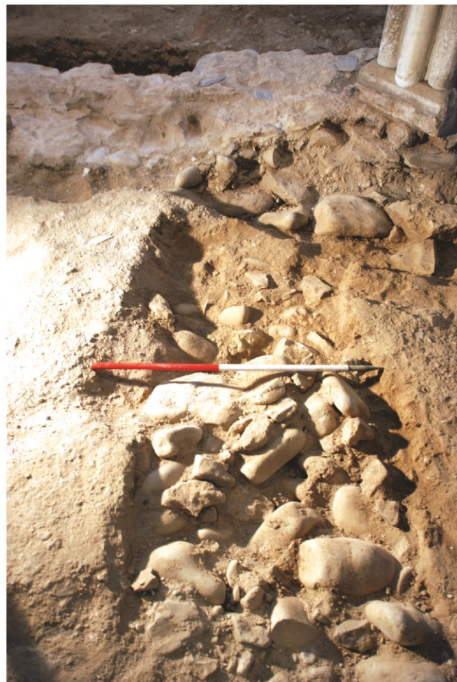
Plate 7 13th-century transept foundation (57), looking north.
