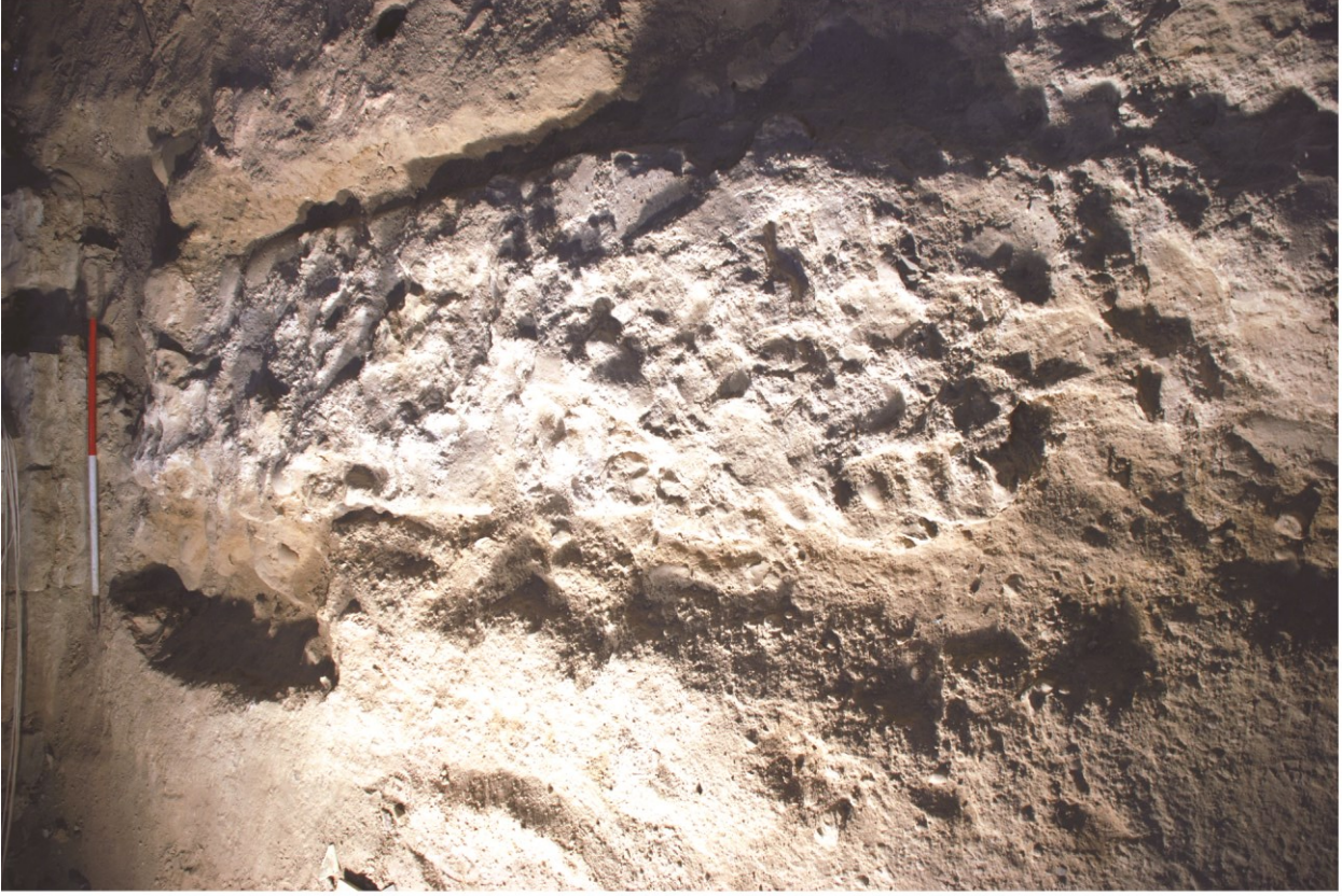
Plate 9 15th-century chancel foundation (43), looking east.
