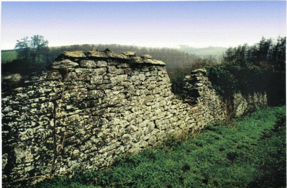
Plate 46. Deer park wall, showing intact coping stones.
