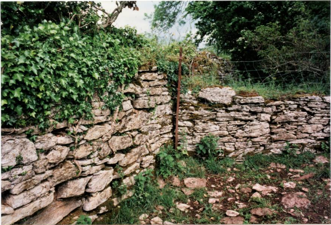
Plate 43. Junction of 'inner wall' with deer park wall, showing the former abuts the latter, looking east.
