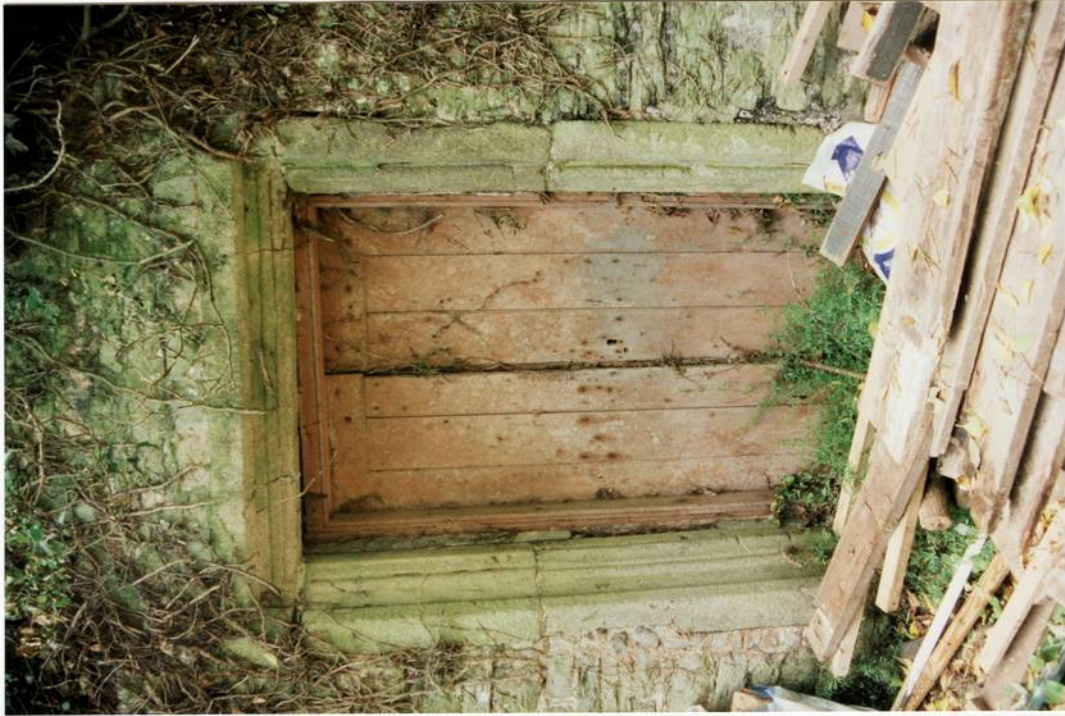
Plate 25. Granite door surround in ruined stable and coach house, looking south.
