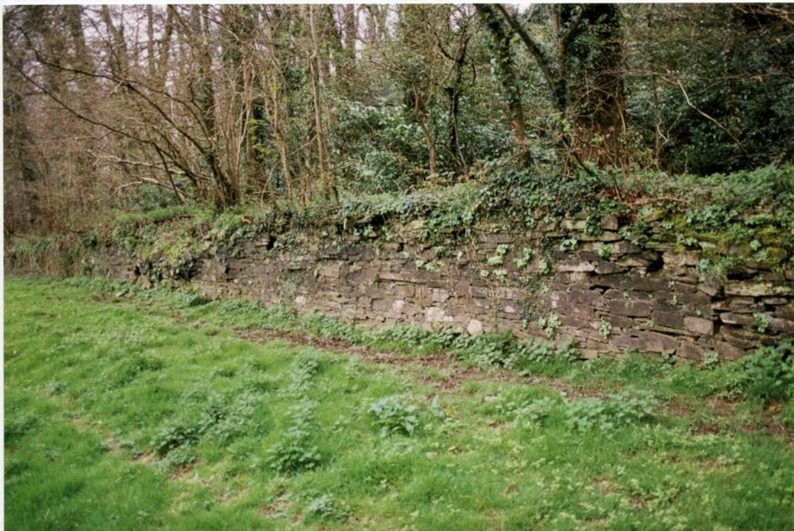
Plate 42. Stone boundary wall flanking old carriage drive, looking north-east.
