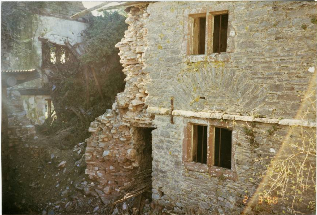
Plate 32. Week farmhouse, showing red sandstone, 16th-century windows and Beer stone string course.
