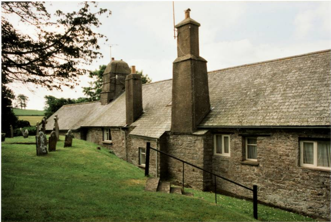
Plate 20. Rear of old church house to west of church, looking south-west.
