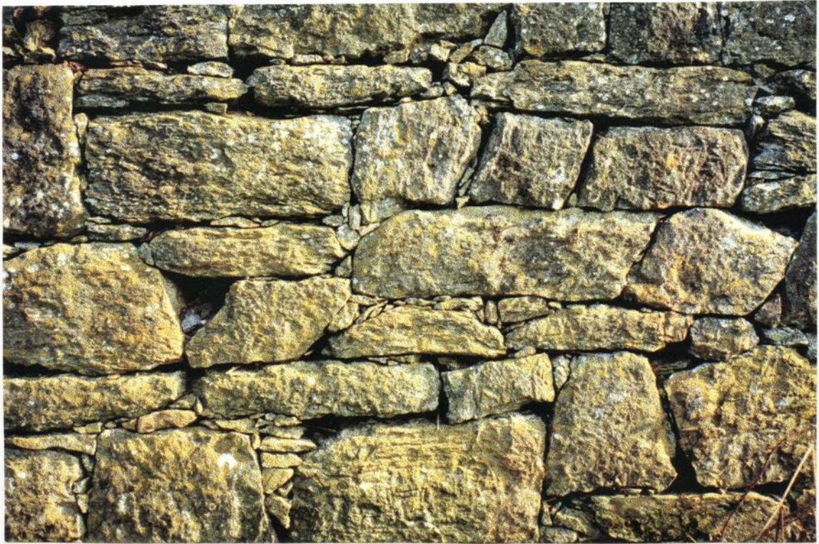
Plate 45. Deer park wall, showing detail of construction.
