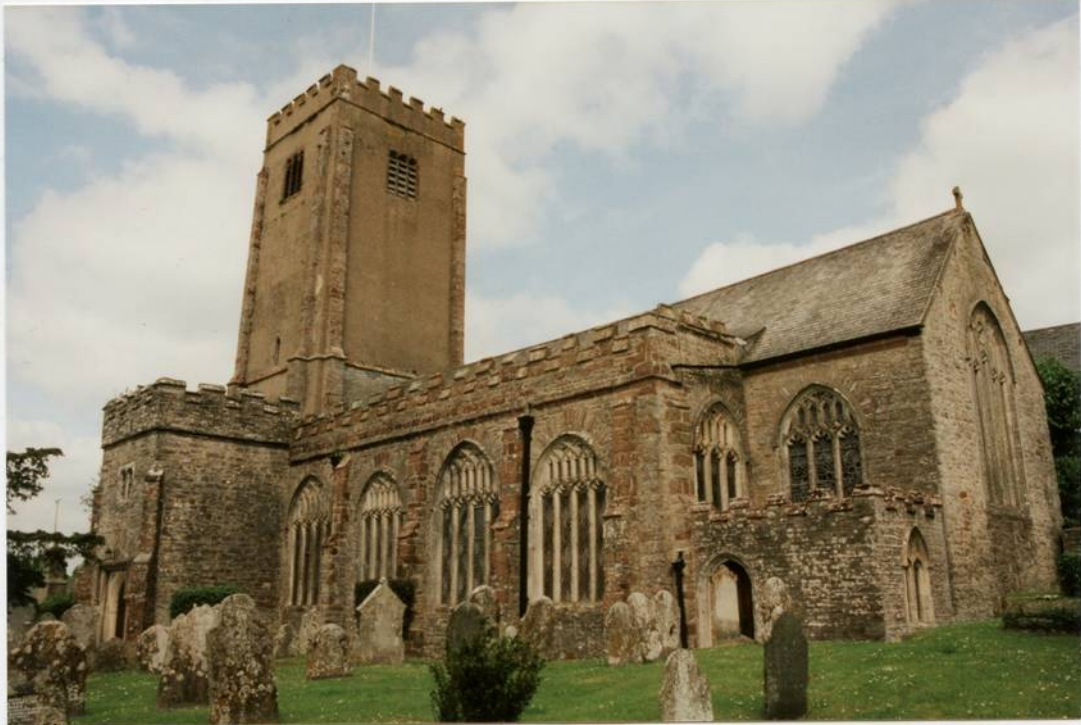
Plate 14. St. Mary's Church, looking north-west.
