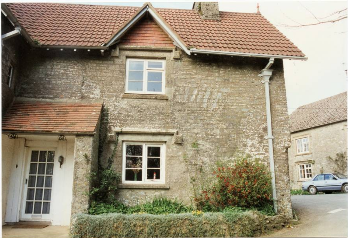
Plate 44. Castle Lodge, showing old relieving arch in front wall, looking north.
