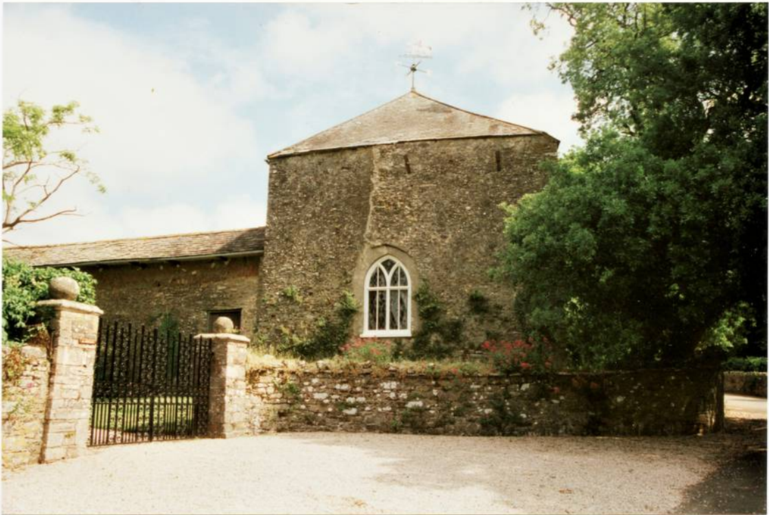
Plate 19. Late medieval or 16th-century stone barn to east of church, looking north.
