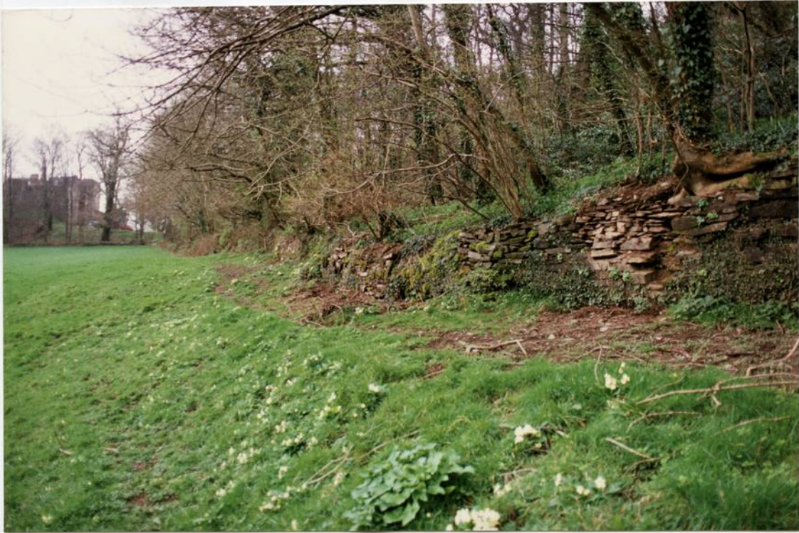
Plate 41. Stone revetment for old carriage drive leading to the castle, looking north-east.
