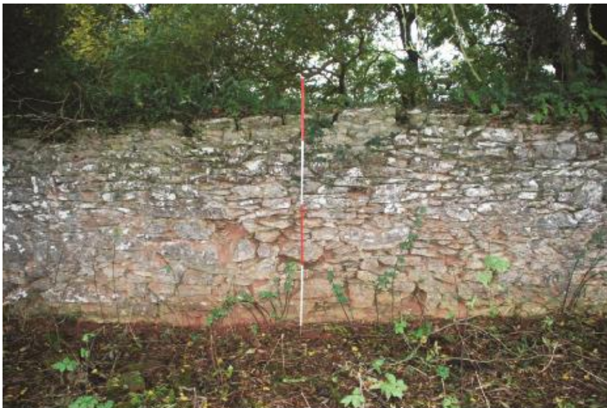
Plate 11 The wall in Torr, showing red earth bonding, looking southwest.
