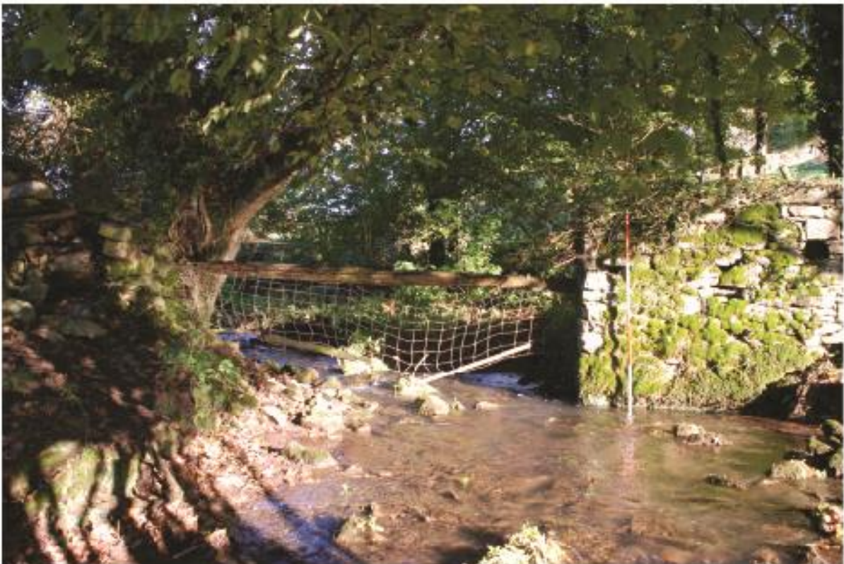
Plate 30 The gap in the wall to let Gatcombe Brook through at the west end of the park, looking east.
