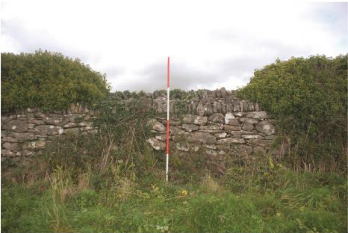
Plate 24 The wall in Clumps showing post-medieval pitched stone capping, looking northeast.
