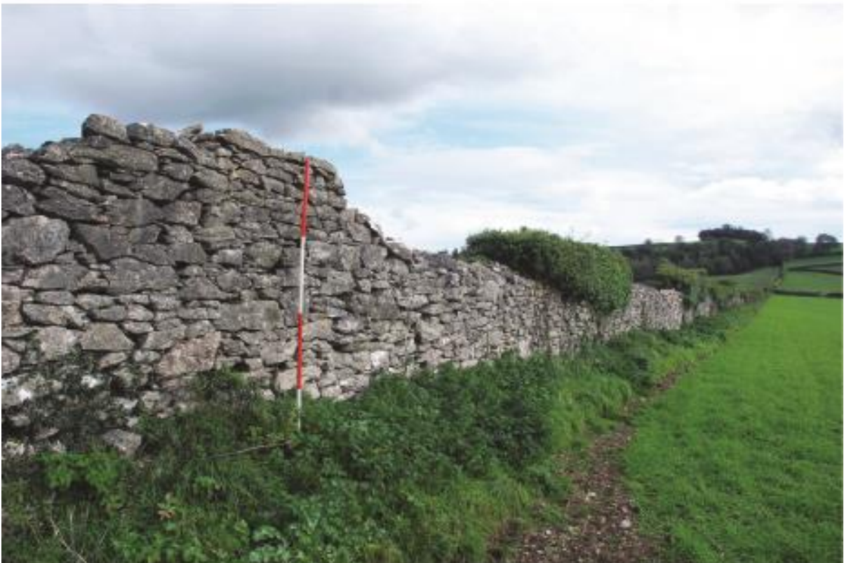
Plate 16 The wall in Great Slade showing large irregular stones with little coursing, looking east.
