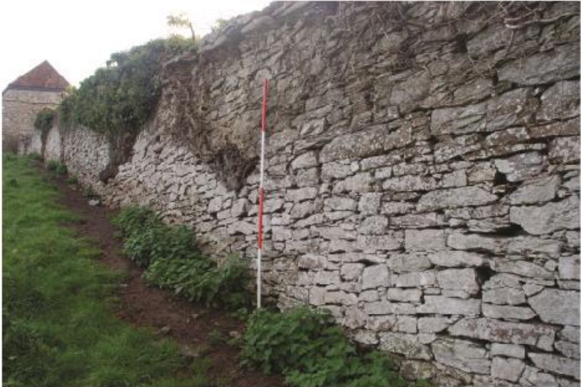
Plate 17 The wall in Big Summerhill showing courses kept level on slope, looking southeast.
