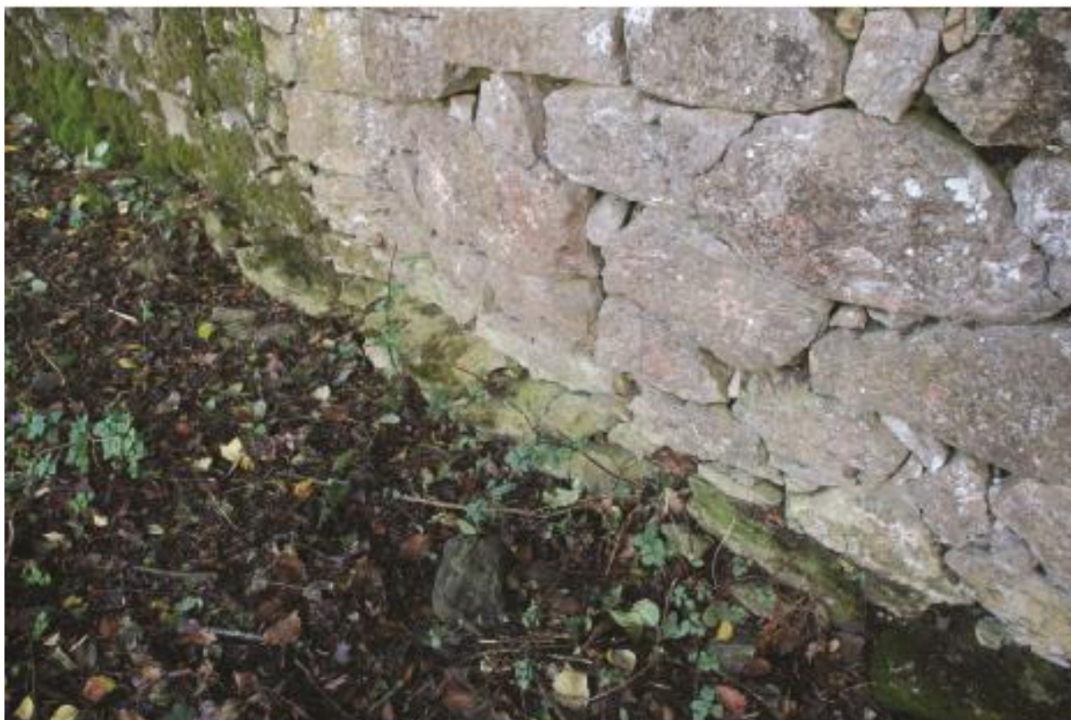
Plate 12 The plinth on the outside of the wall in Waynaps, looking southeast.
