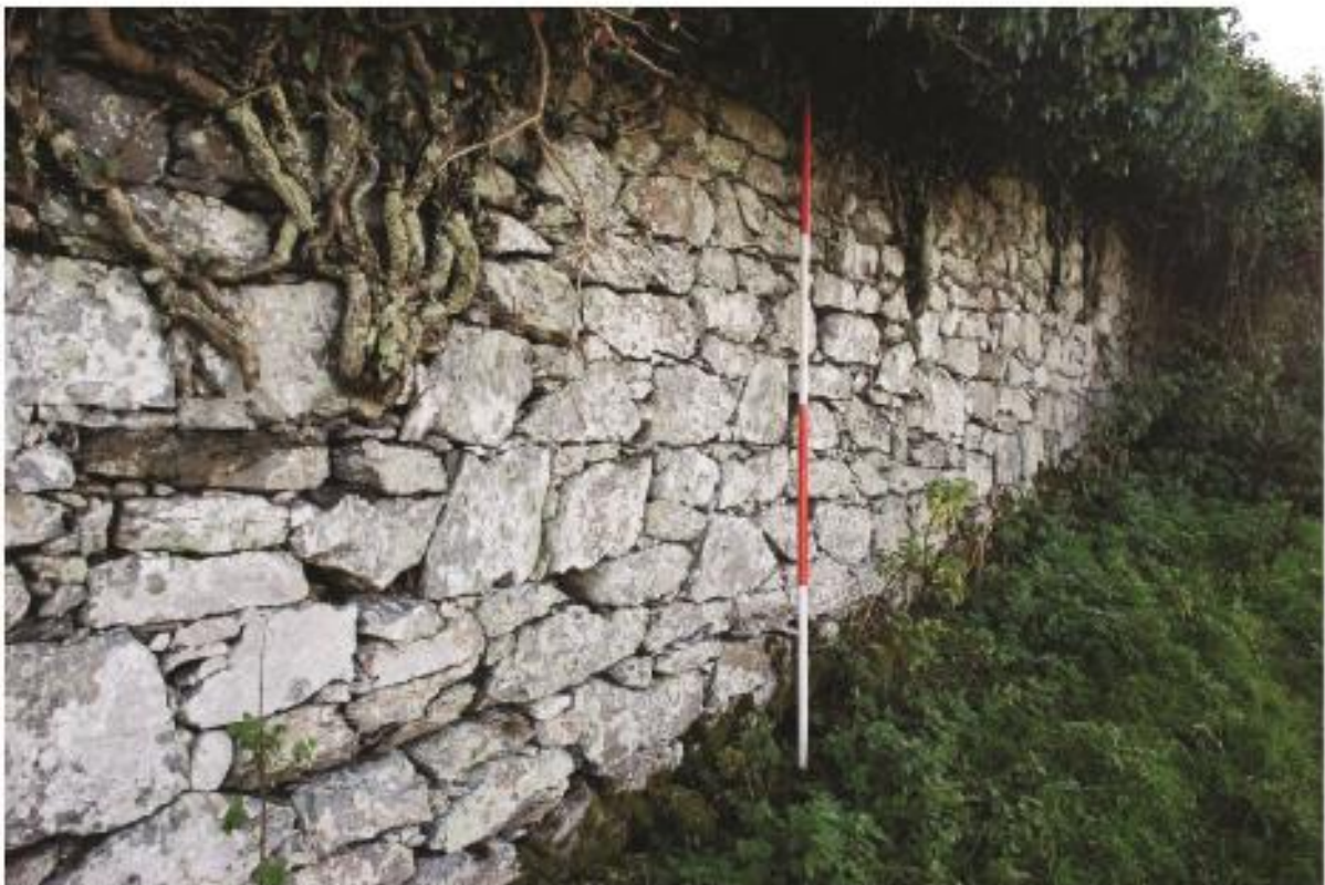
Plate 18 The wall in Croft showing courses kept level on slope and small stone packing, looking south.
