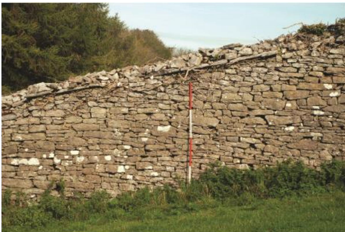
Plate 9 Almost intact section of the wall in Lodge Meadow, looking north.
