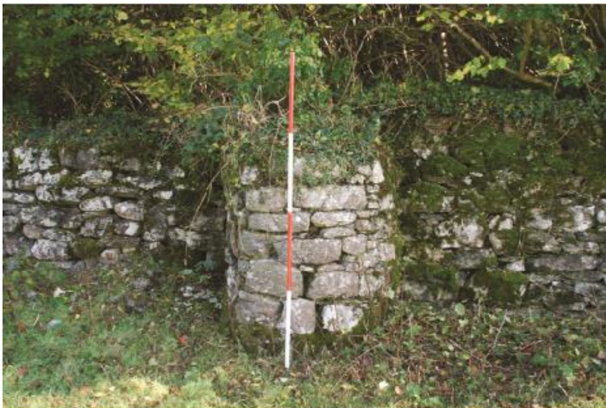
Plate 25 The wall in Custer Park showing post-medieval round gate pier built against the wall, looking east.
