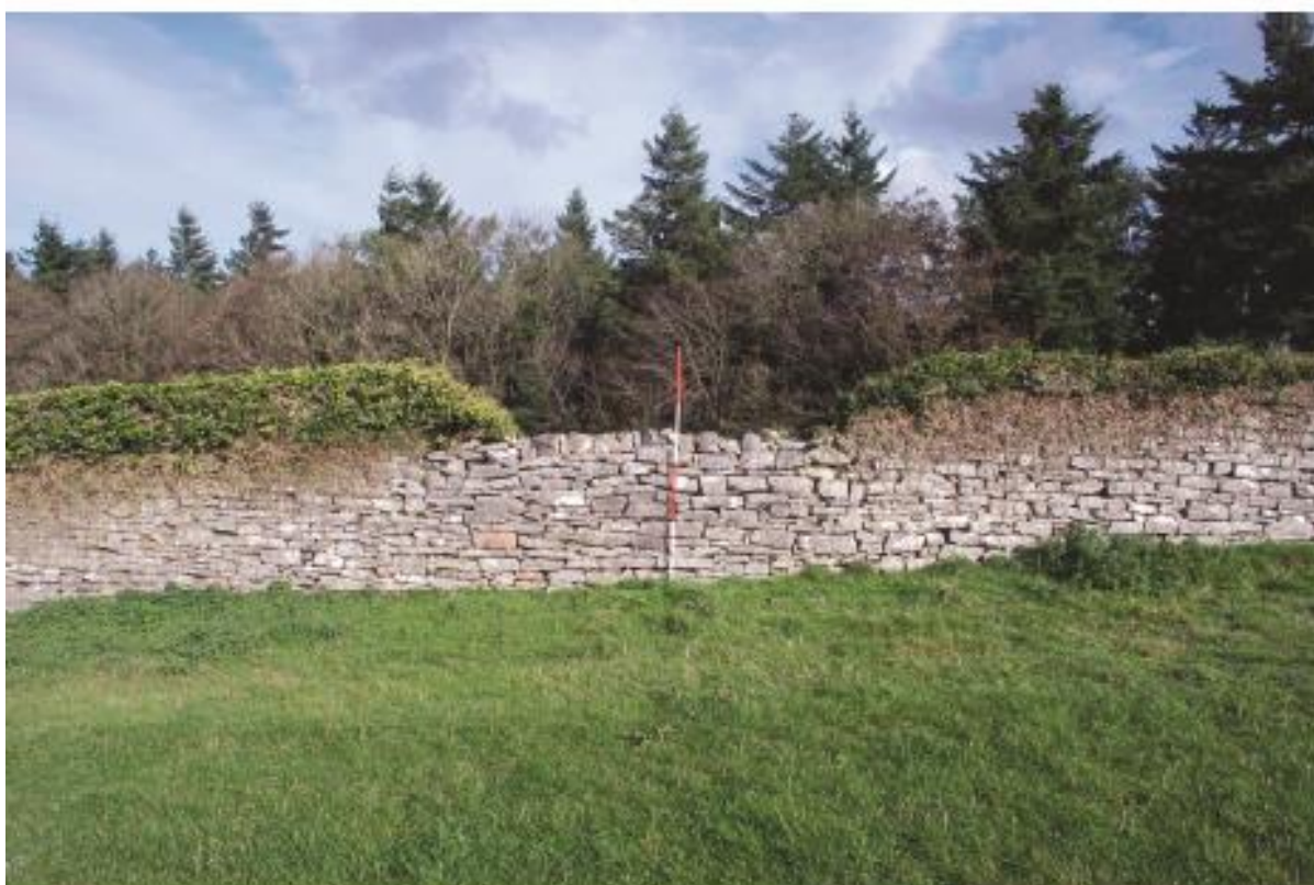
Plate 26 The wall in Little Slade showing modern repair, looking northeast.
