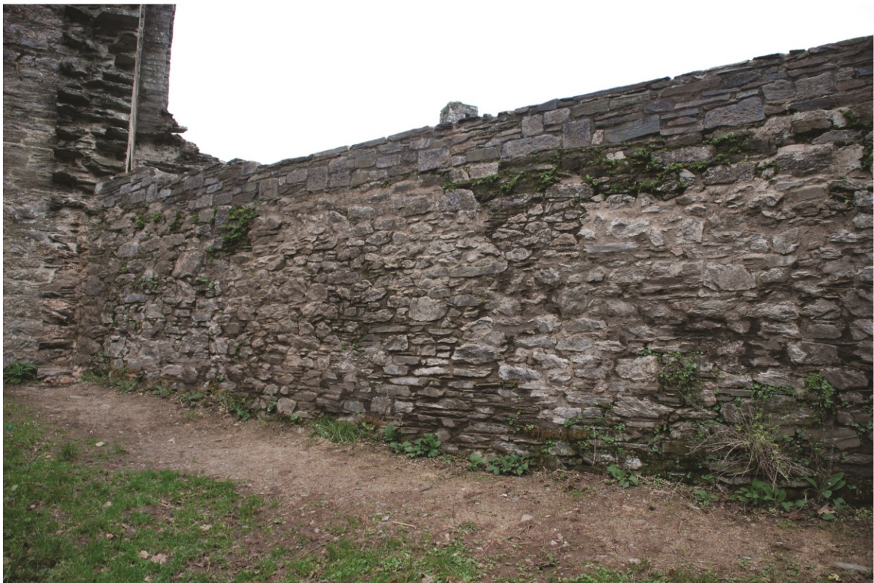
Plate 26 The boundary wall after re-pointing, looking north.
