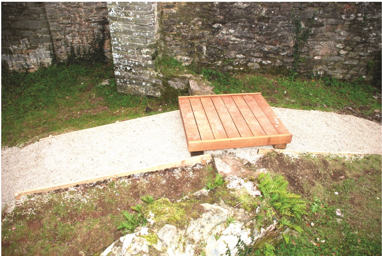
Plate 23 The new access ramp leading to the north terrace, looking west.
