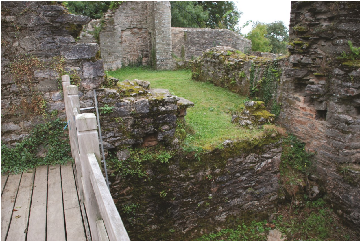
Plate 16 The northeast wall of the kitchen before extension of decking, looking west.
