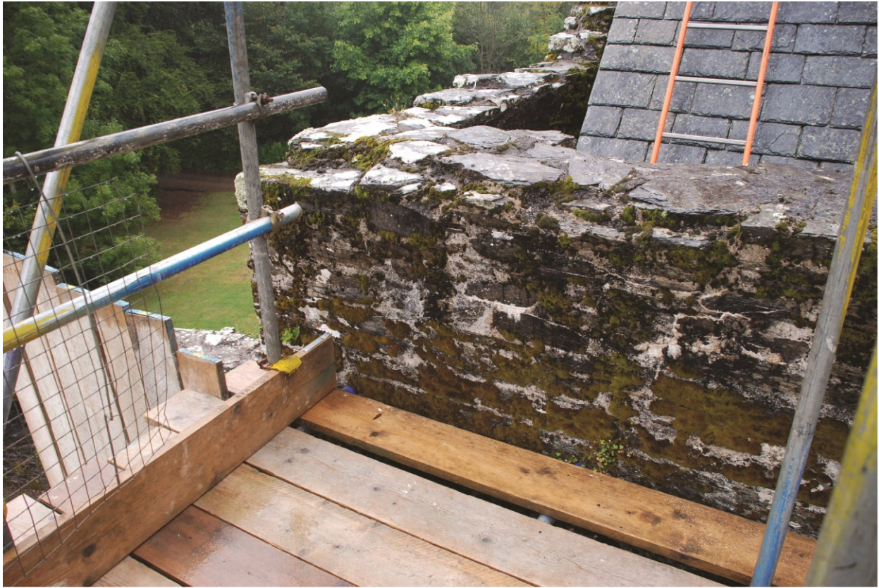
Plate 3 The gatehouse parapet wall, NE corner, before conservation work, looking east.
