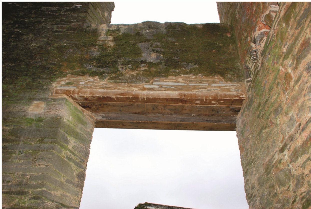
Plate 12 The kitchen quarter after conservation work, new first-floor lintels, looking northeast.
