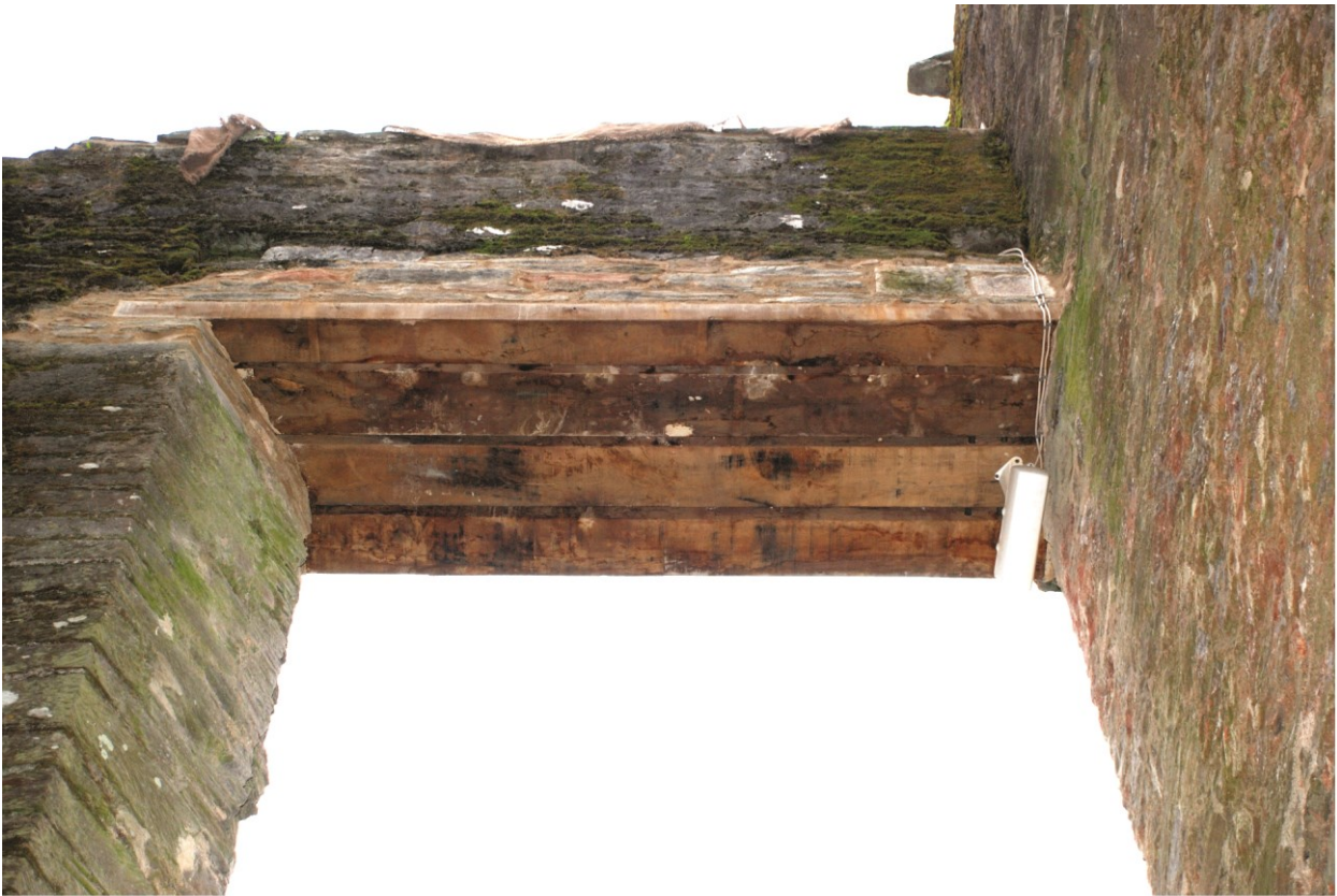
Plate 11 The kitchen quarter after conservation work, new second-floor lintels, looking northeast.
