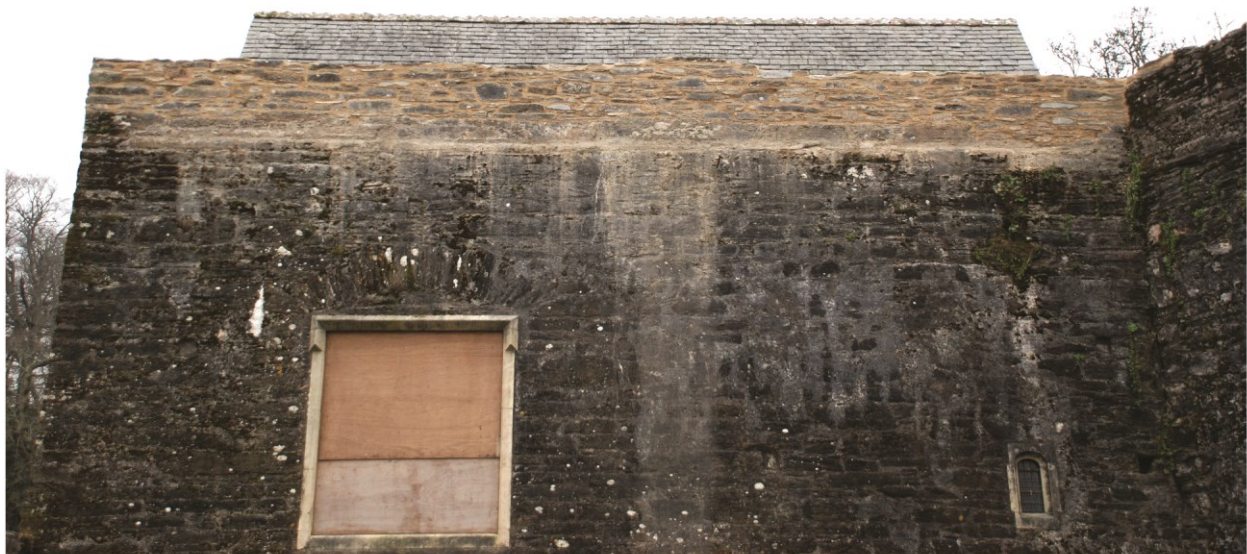
Plate 6 The gatehouse parapet wall after conservation work, looking southeast.
