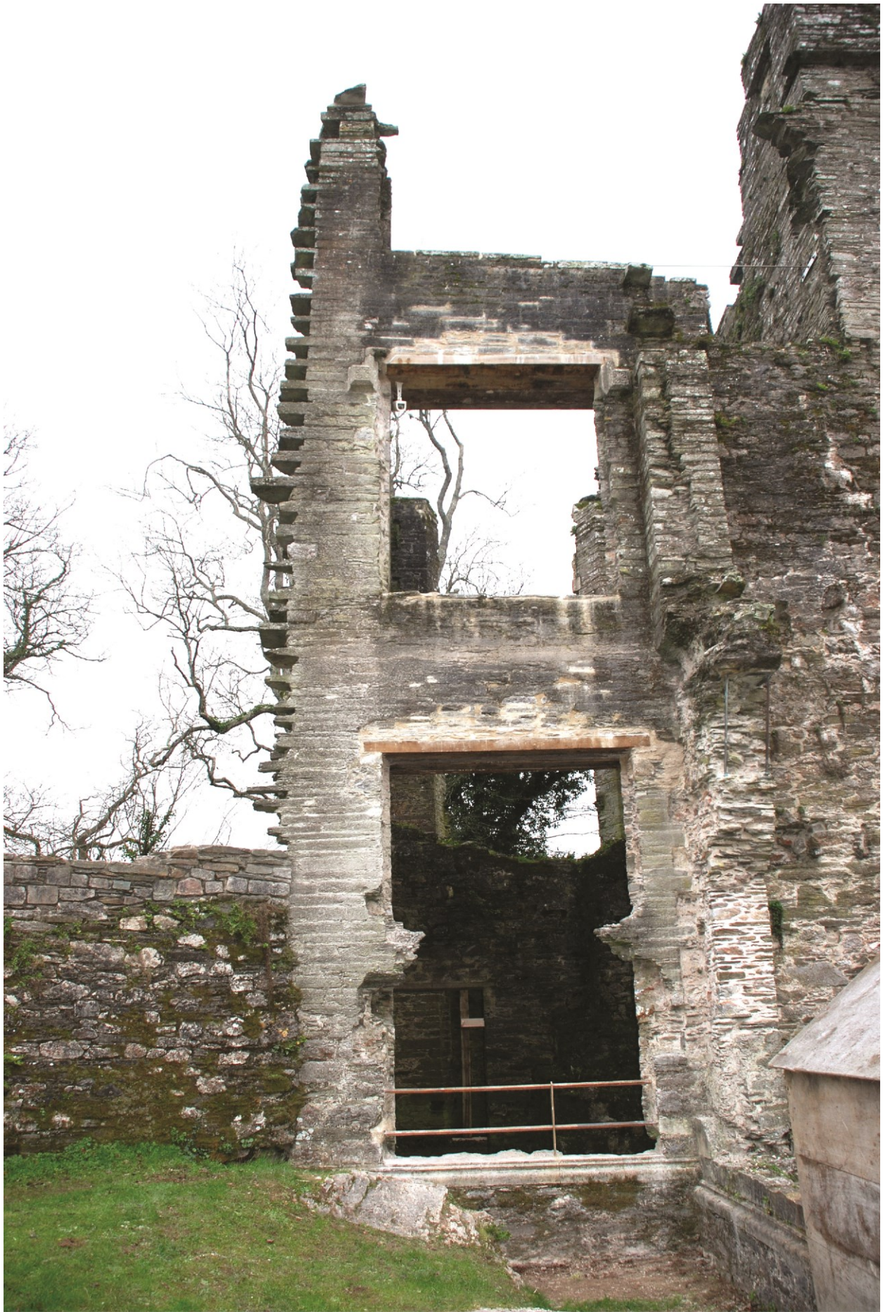
Plate 15 The kitchen quarter after conservation work, looking southwest.
