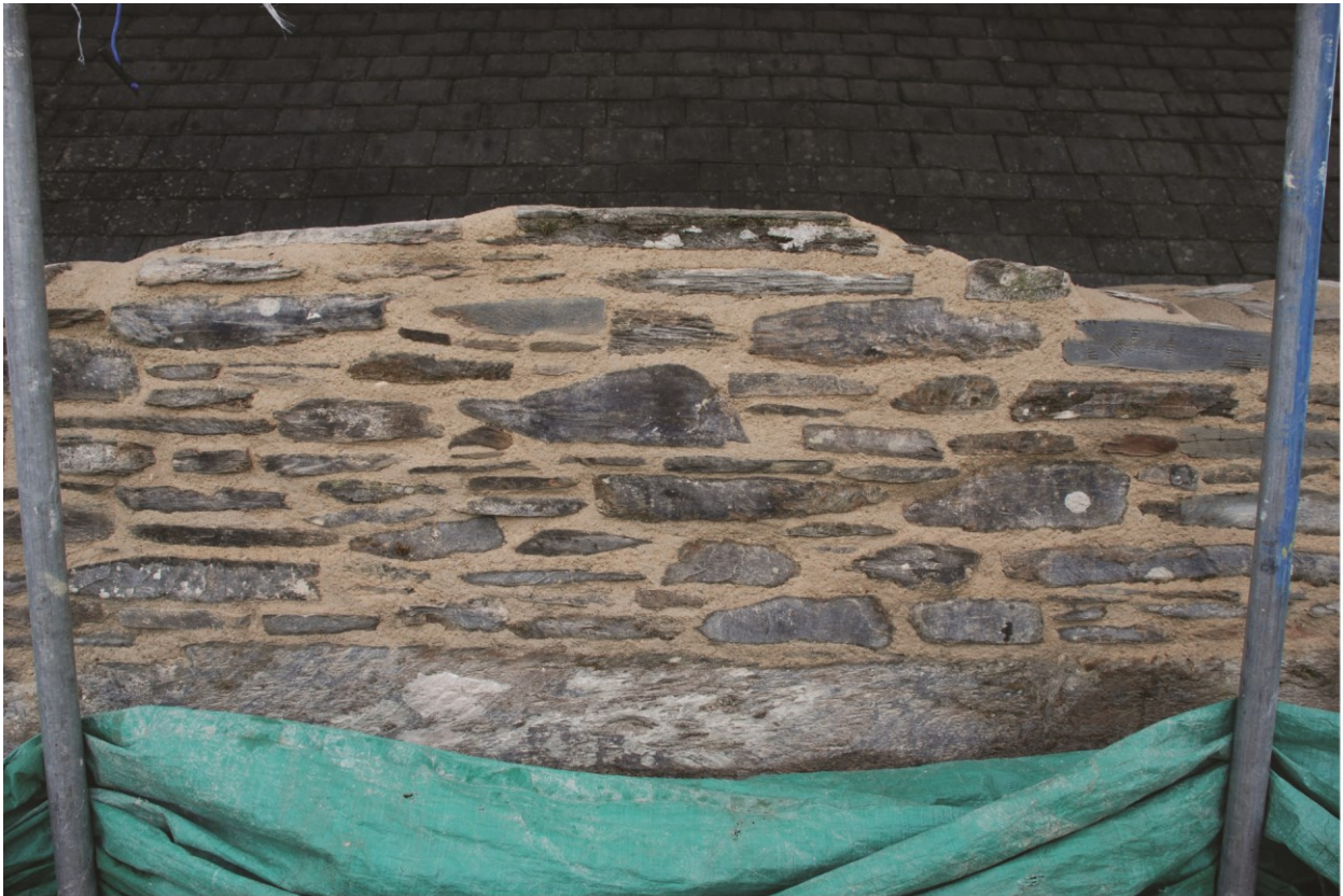
Plate 5 Detail of the gatehouse parapet wall after conservation work, looking southeast.
