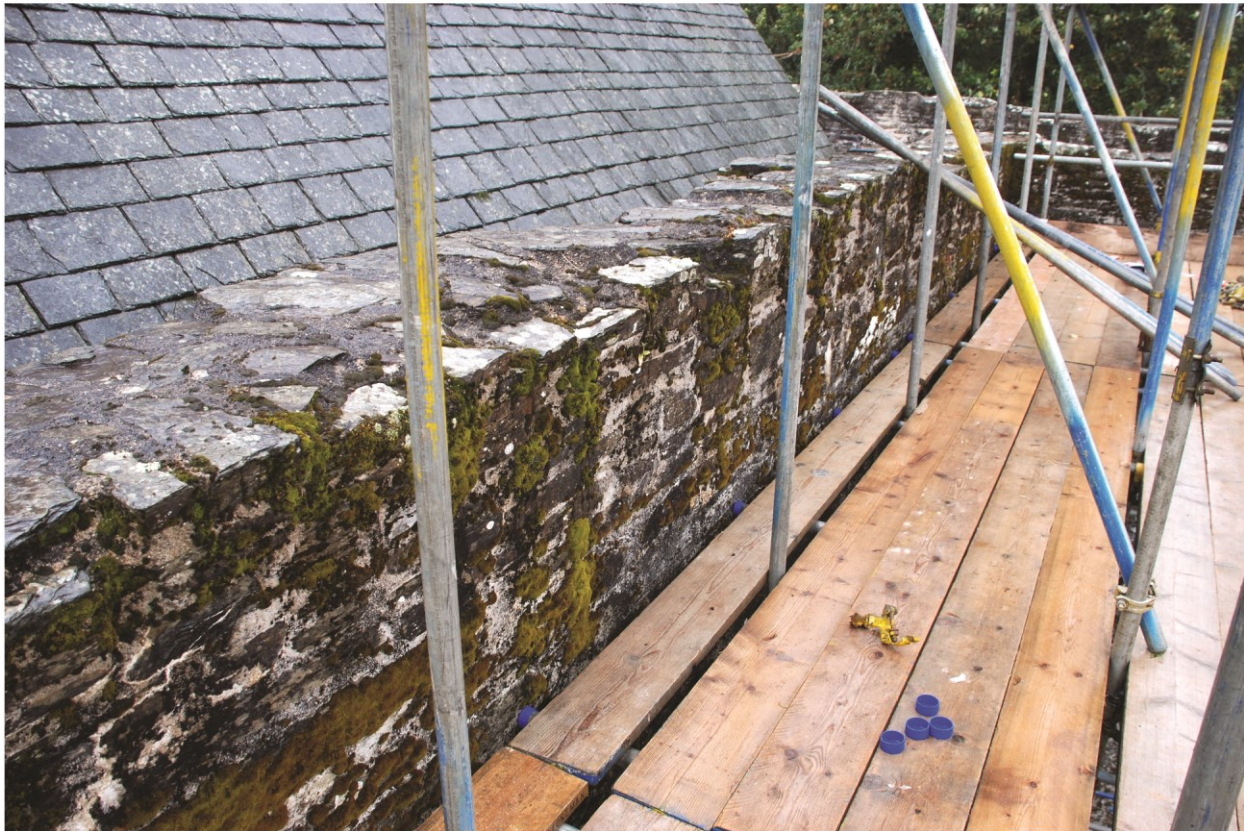
Plate 2 The gatehouse parapet wall before conservation work, looking south.
