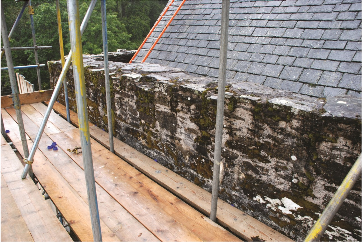
Plate 1 The Gatehouse parapet wall before conservation work, looking east.
