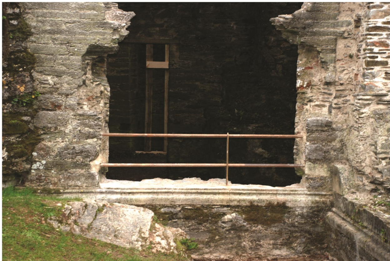
Plate 14 The kitchen quarter after conservation work, new railing and consolidation of the window sill, looking southwest.
