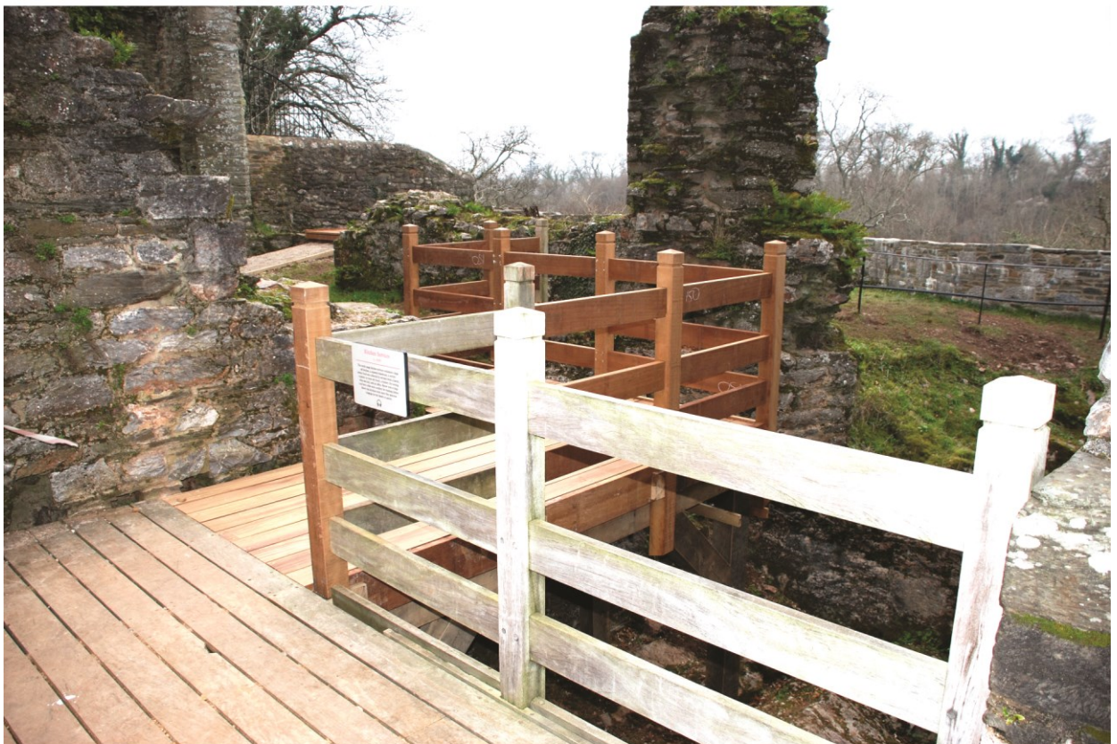
Plate 17 The northeast wall of the kitchen after extension of decking, looking west.
