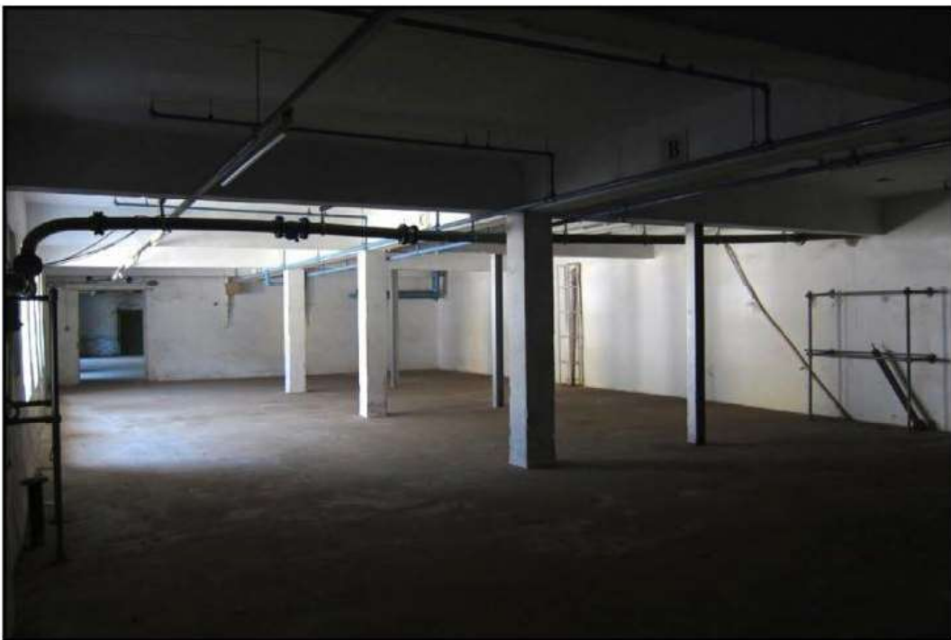
Photo. 14 Basement of the north range, looking south-west.
