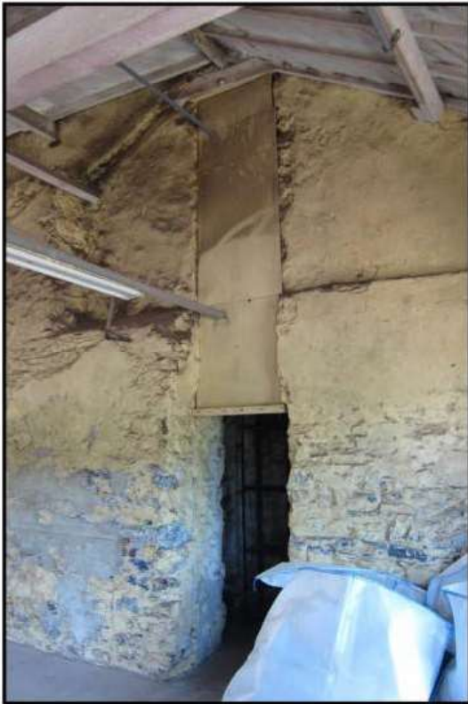
Photo. 13 Lavatory entrance on the second floor of the north range.
