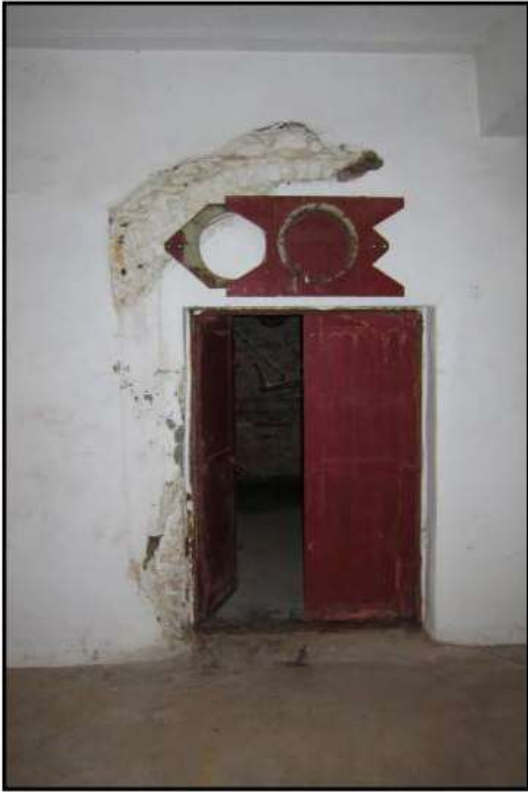
Photo. 15 Tunnel entrance in north-west corner of the north range basement.
