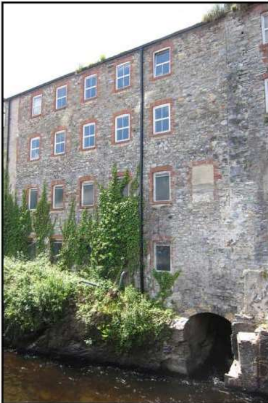
Photo. 4 The leat outlet at the north-east corner of the south range, looking south-west.
