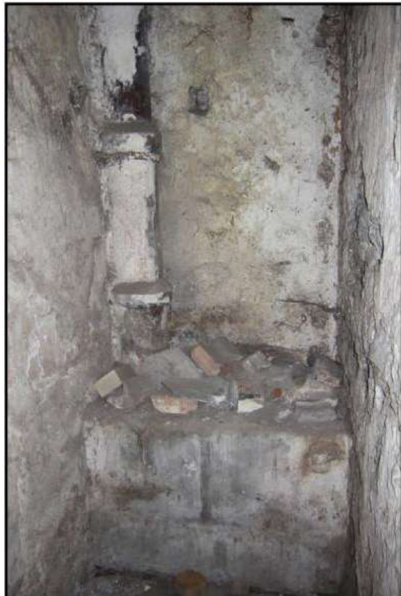
Photo 12. North range, first floor lavatory interior.
