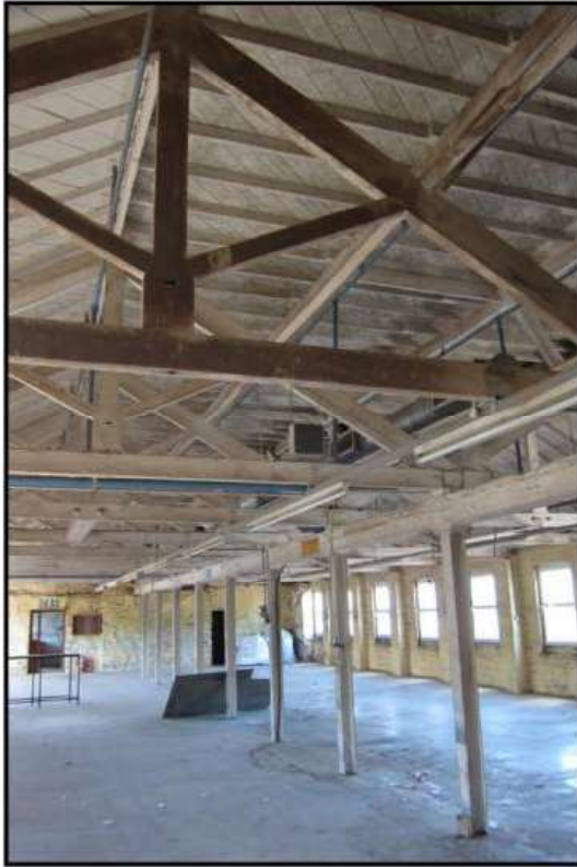
Photo. 9 North range roof, looking north.
