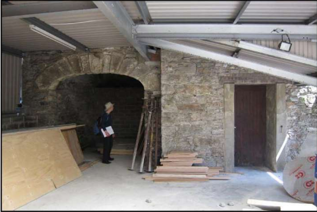
Photo. 5 The archway at the base of the tower, looking east.
