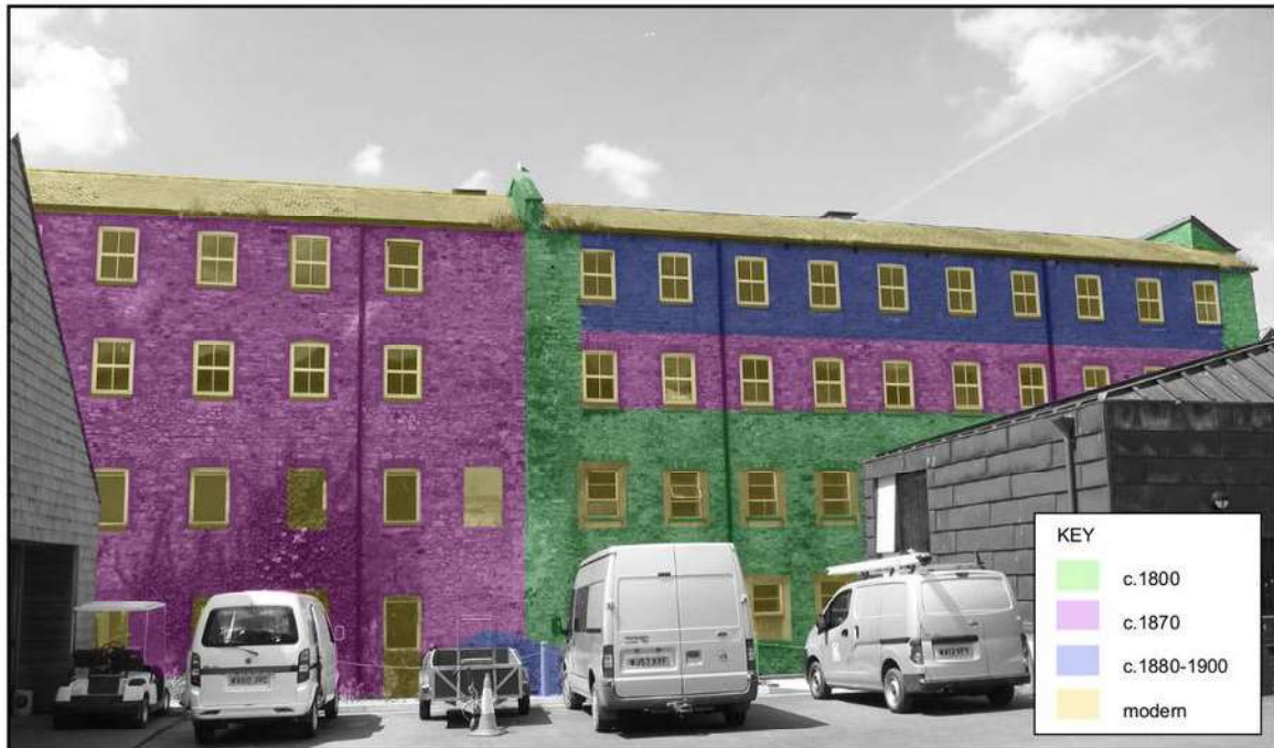
Fig. 11 West elevation construction phases (windows are shown as modern to denote recent replacements, not modern openings).
