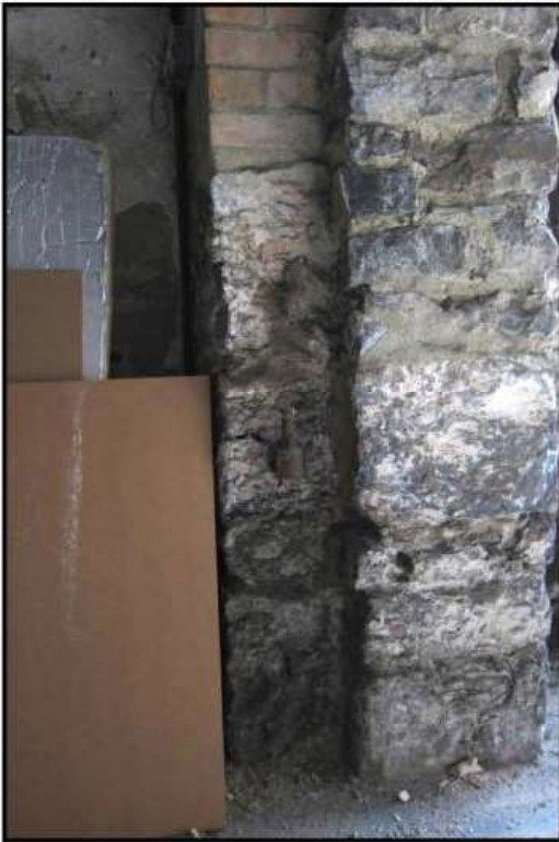
Photo. 6 The pintle within the tower entrance arch, looking south.
