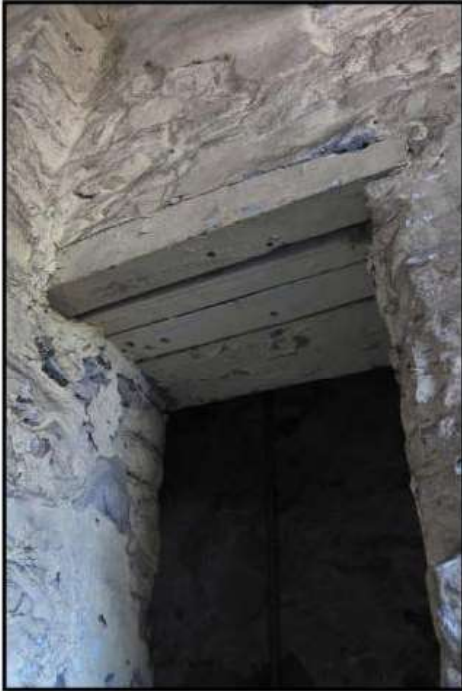
Photo. 11 North range, first floor lavatory doorway.
