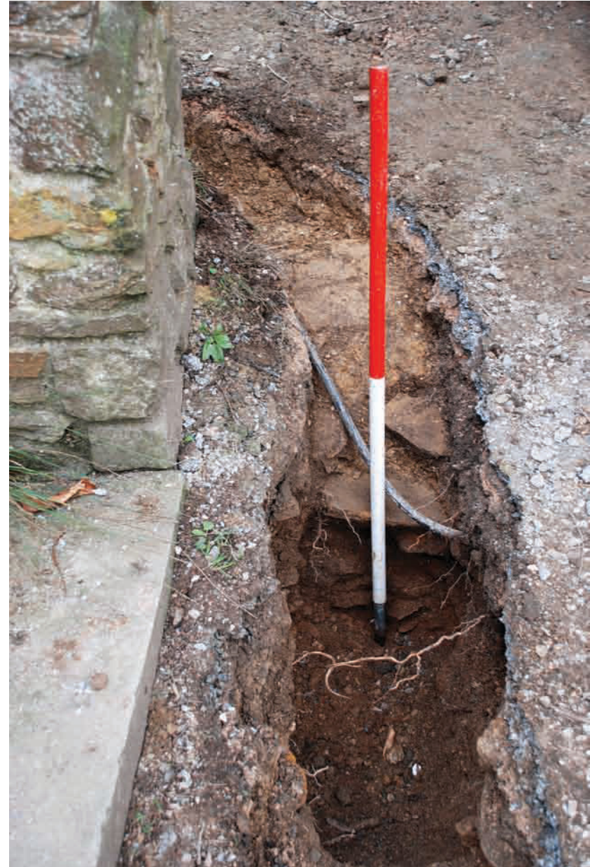
Plate 2 Wall 8, looking W.
