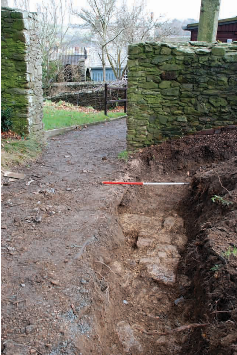
Plate 1 Wall 6, looking E.
