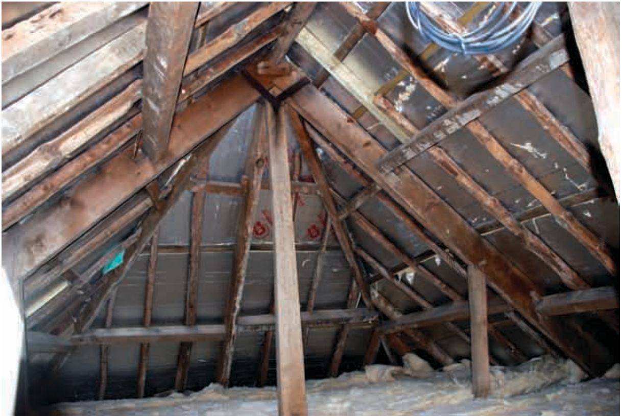
Plate 1 The chapel roof, looking north.
