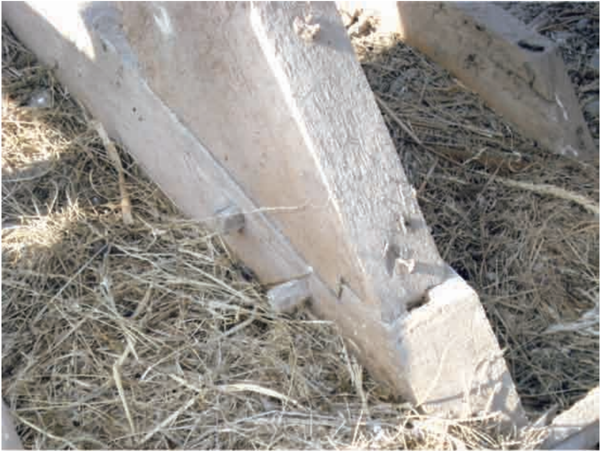
Plate 3 Tie-beam truss pegged mortice and tenon joint, looking southeast.
