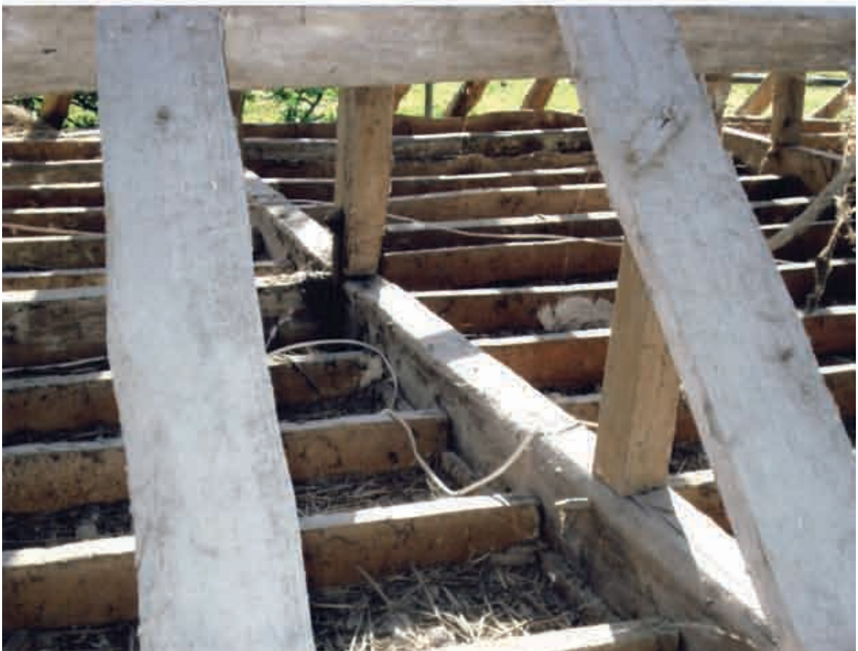
Plate 4 Ceiling timbers, looking southeast.
