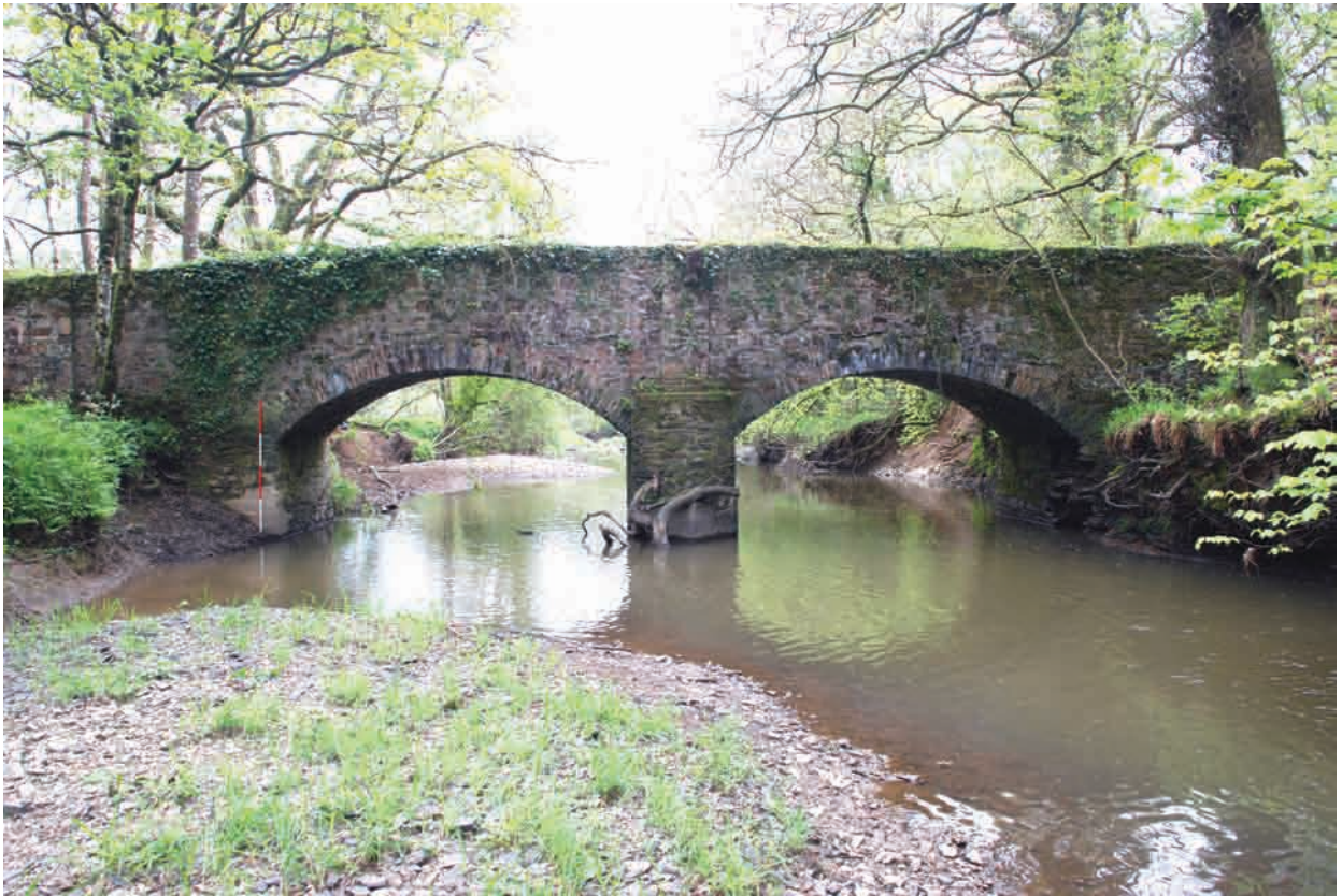
Plate 1 The upstream (northwest) elevation of the bridge.
