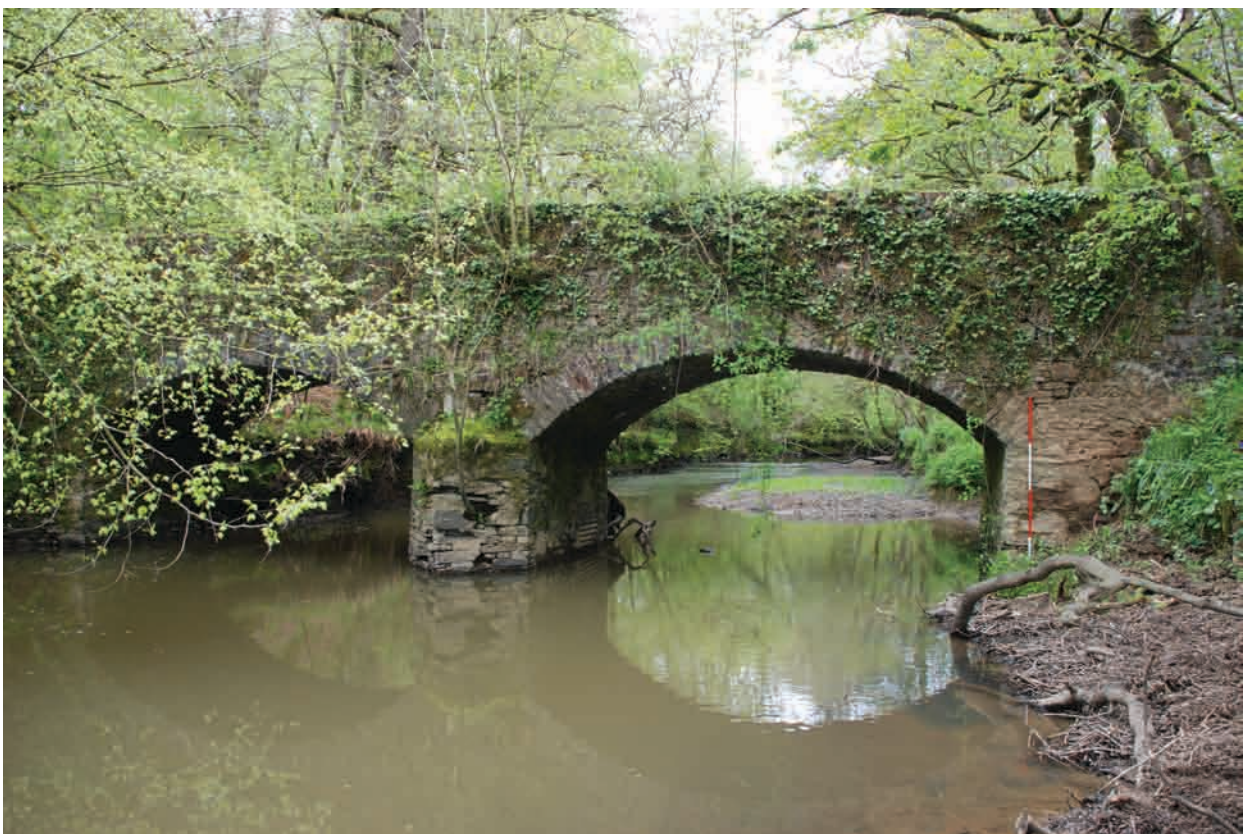
Plate 2 The downstream (southeast) elevation of the bridge.
