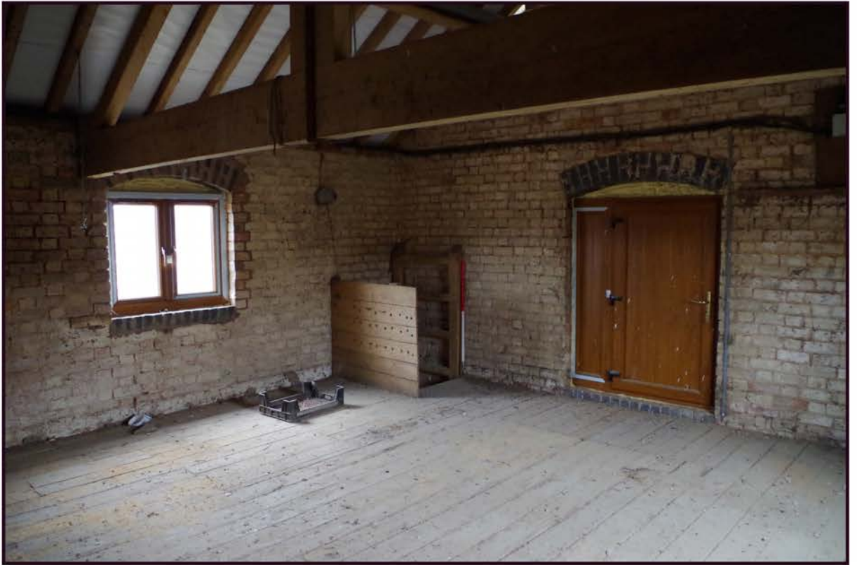
Fig 21: Phase 3 cart shed and stable; first floor
