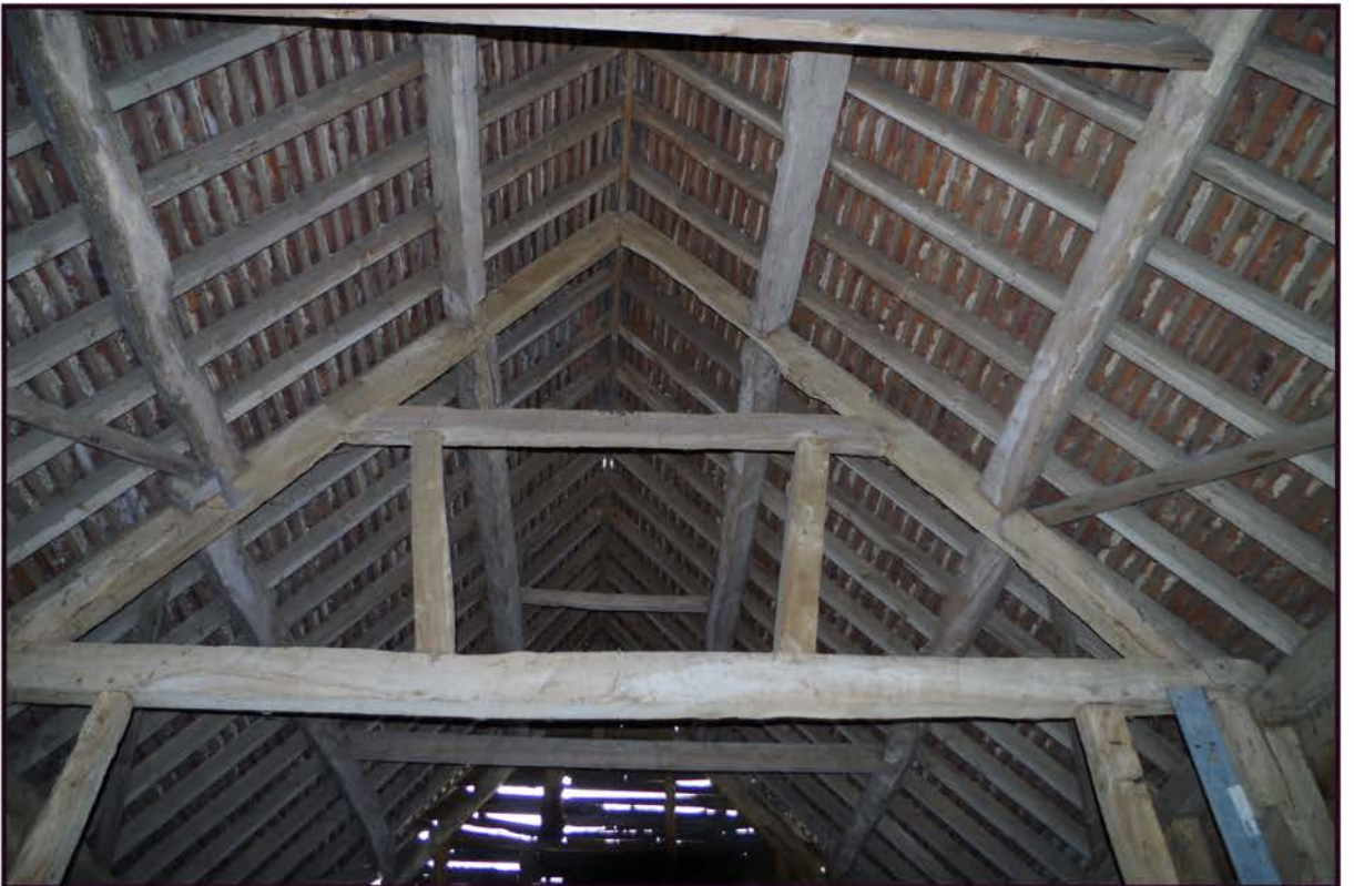
Fig 24: Phase 1 barn; detail of roof truss
