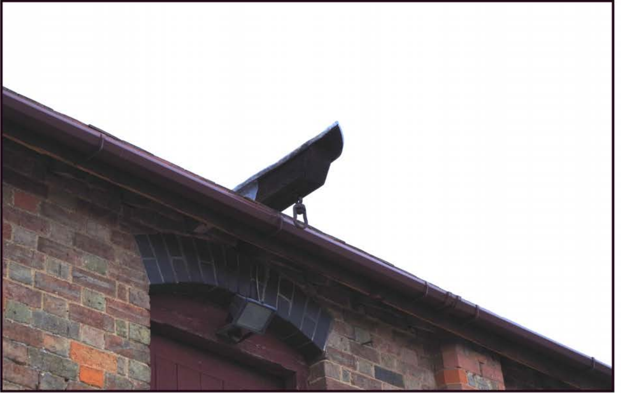
Fig 11: Phase 3 cart shed and stable; east elevation, detail of sack hoist
