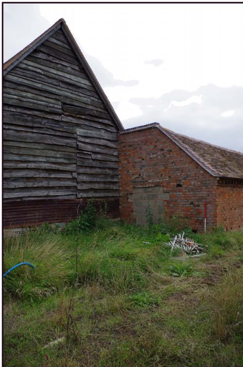
Fig 15: Phase 1 barn; west elevation and Phase 2 shelter shed/implement shed; north elevation
