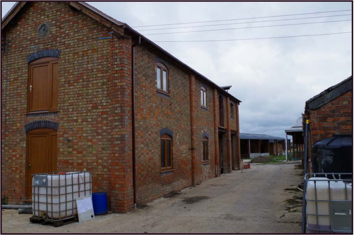
Fig 9: Phase 3 cart shed and stable; east elevation
