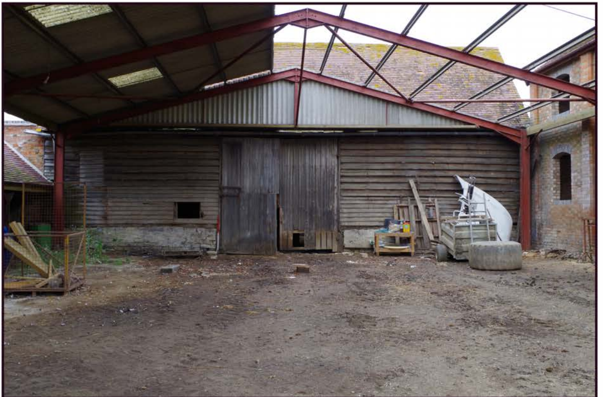
Fig 5: Phase 1 barn; south elevation
