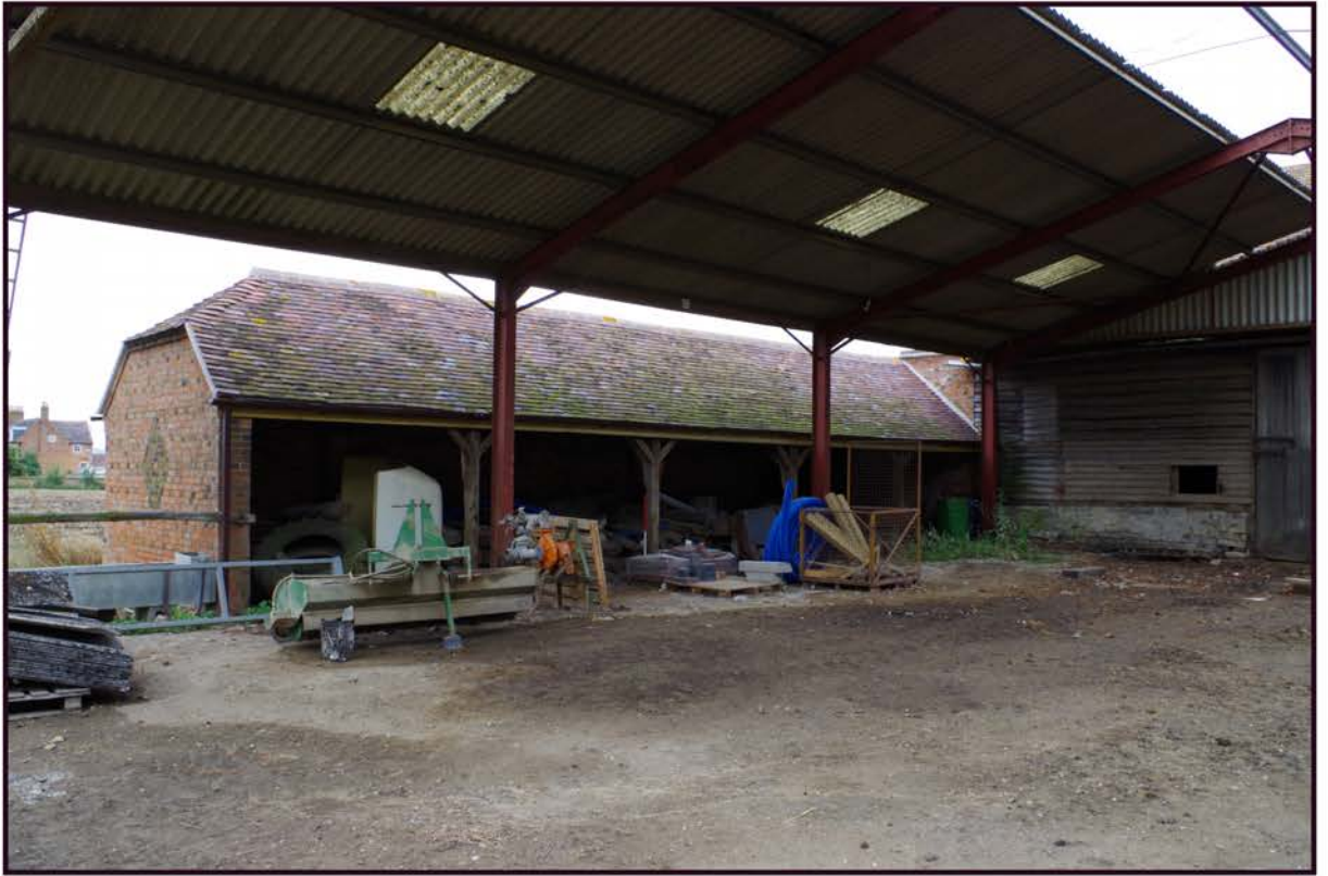
Fig 4: Phase 2 shelter shed/implement shed; east elevation
