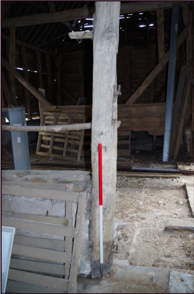
Fig 27: Phase 1 barn; detail of originally gated opening to bay division
