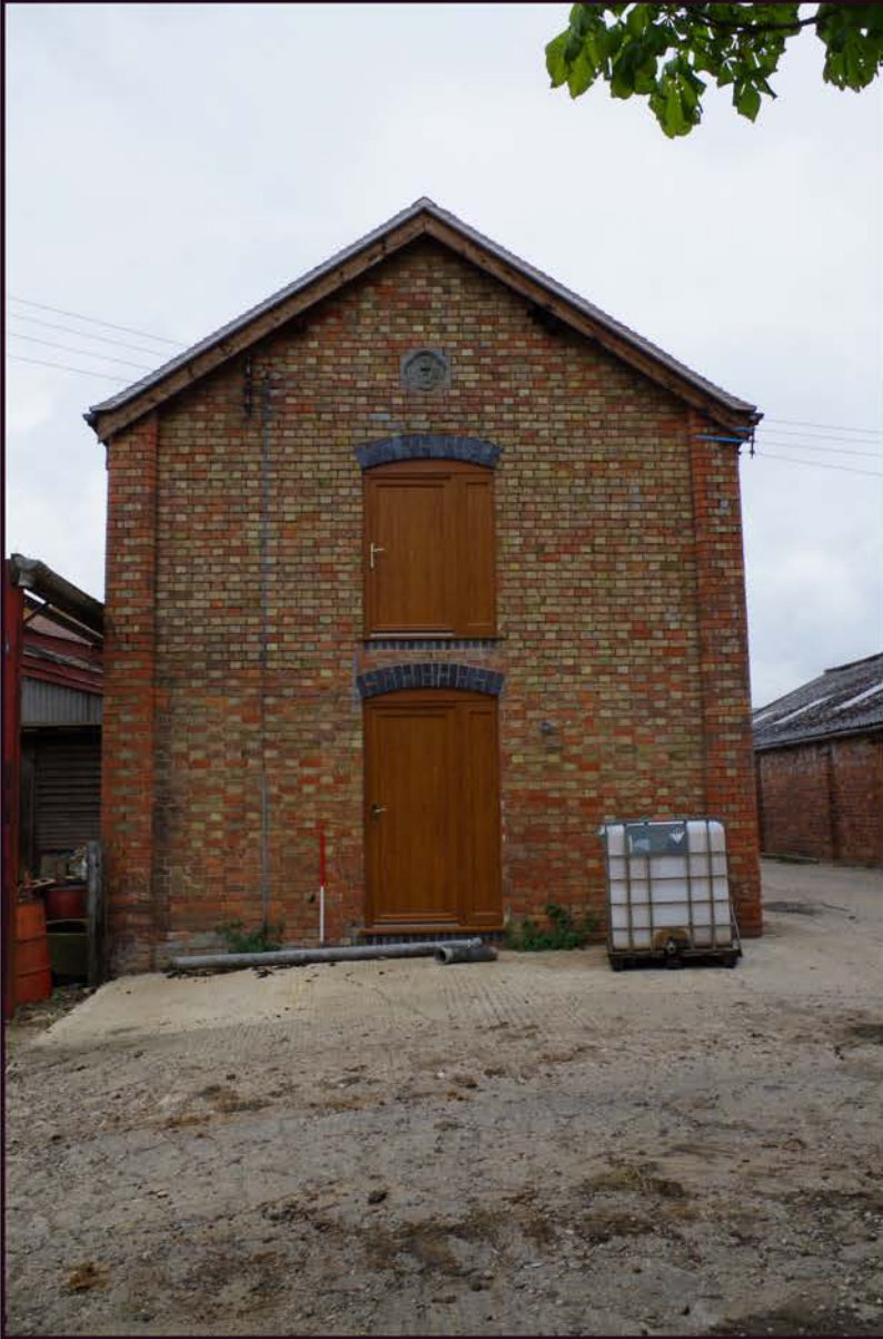
Fig 8: Phase 3 cart shed and stable; south elevation
