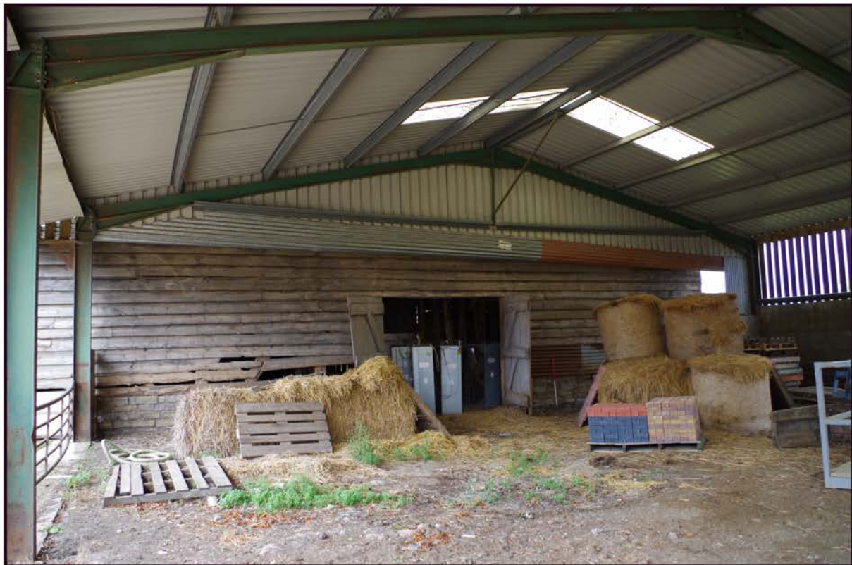
Fig 13: Phase 1 barn; north elevation
