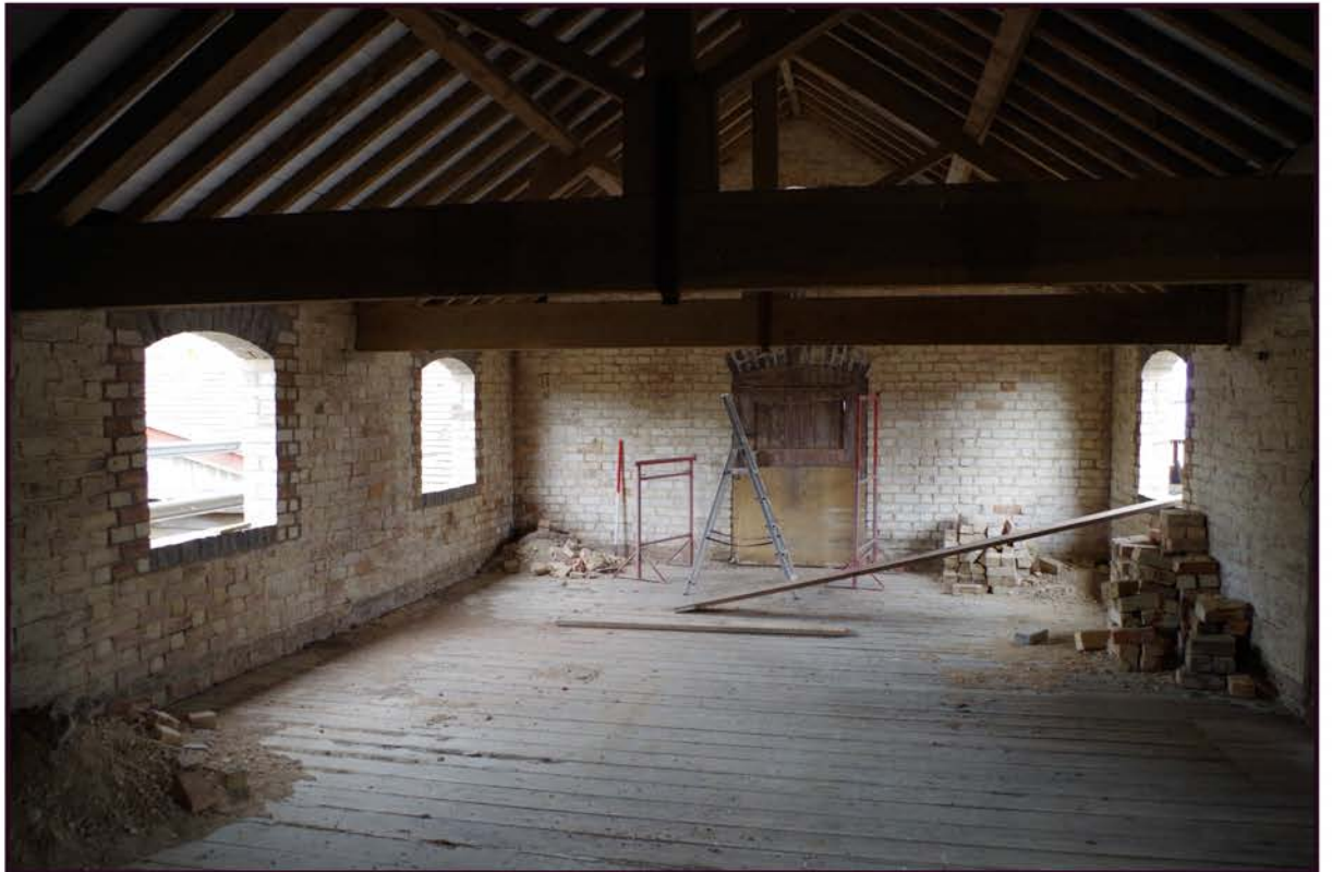
Fig 22: Phase 3 cart shed and stable; first floor
