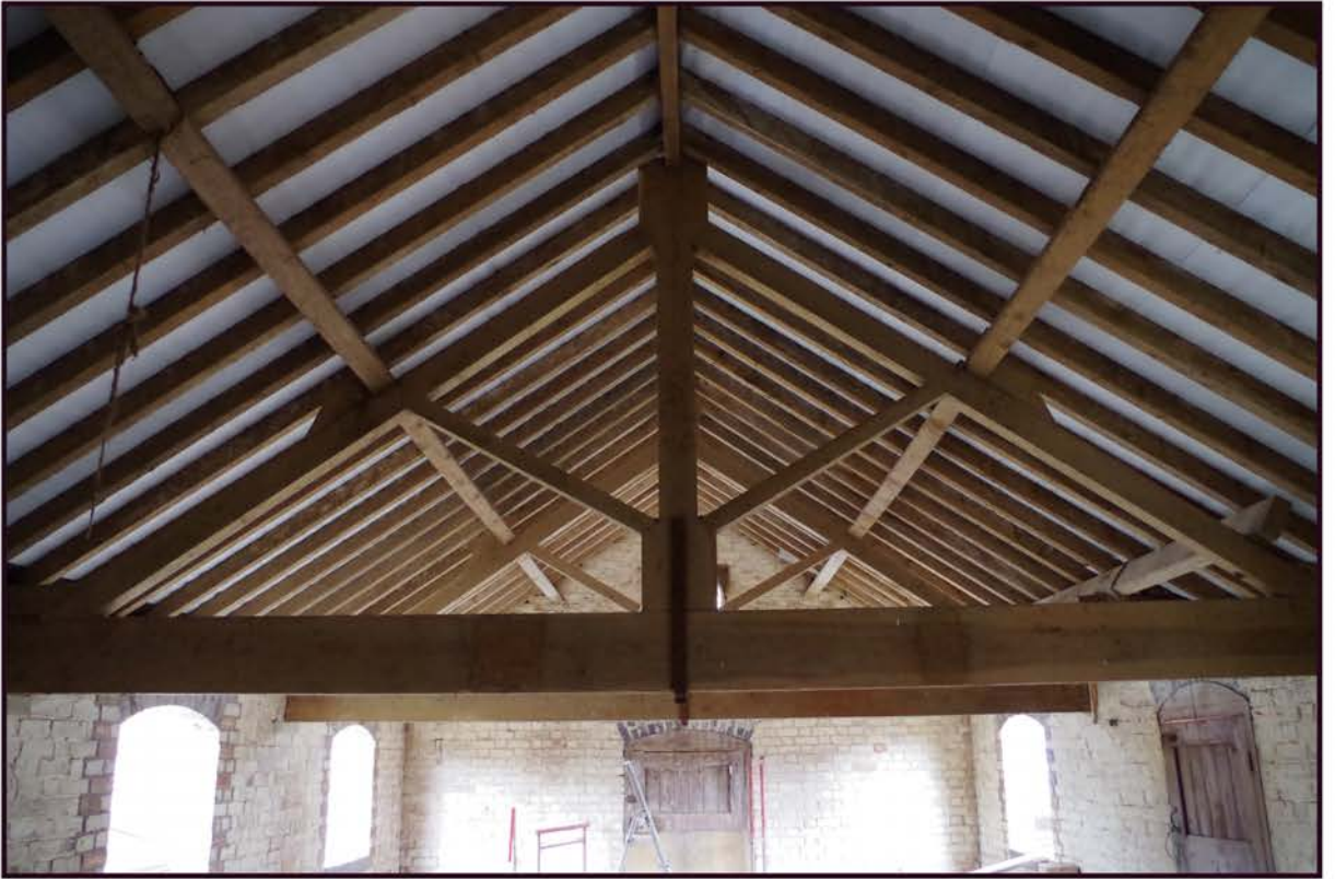
Fig 23: Phase 3 cart shed and stable; detail of roof truss
