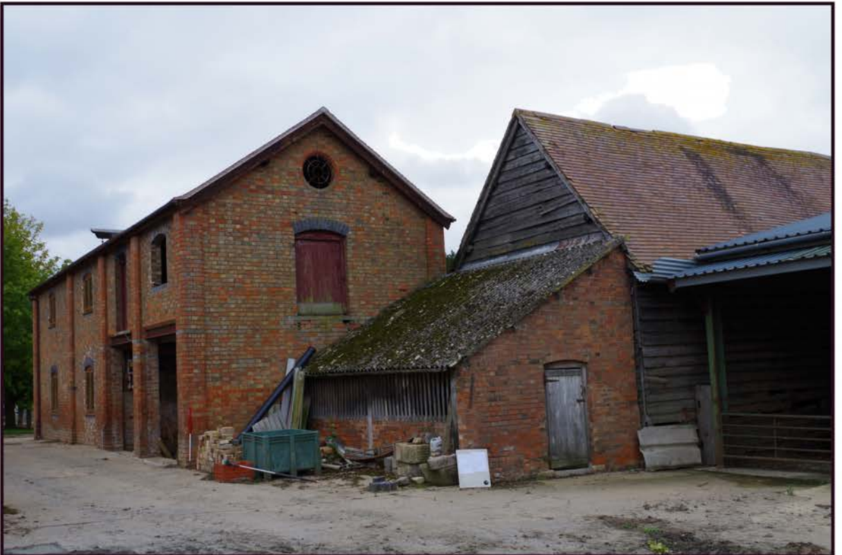
Fig 12: Phase 3 cart shed and stable; north elevation and Phase 4 lean-to
