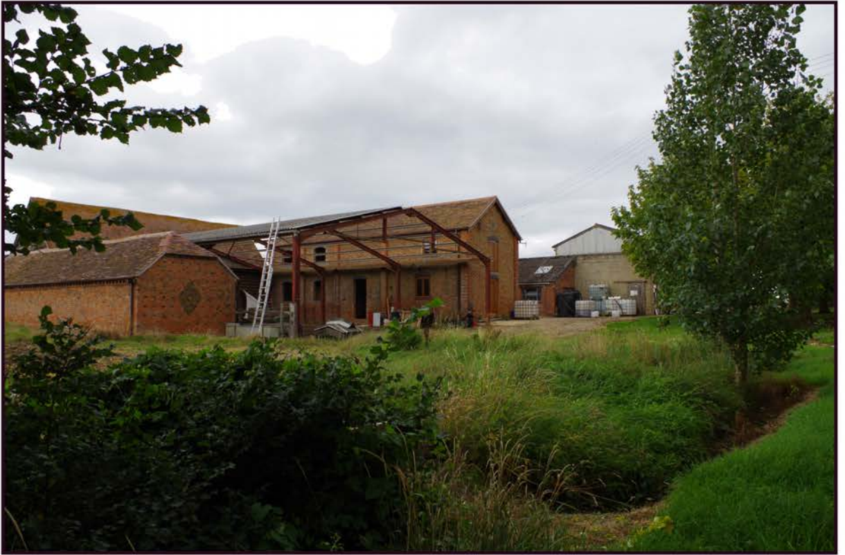
Fig 30: General view of recorded buildings from the south-west
