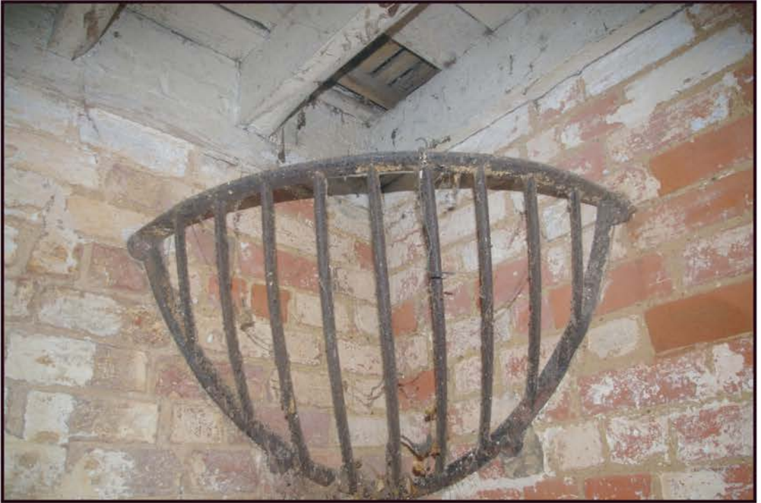
Fig 17: Feeding basket showing hatch in hayloft floor for replenishment
