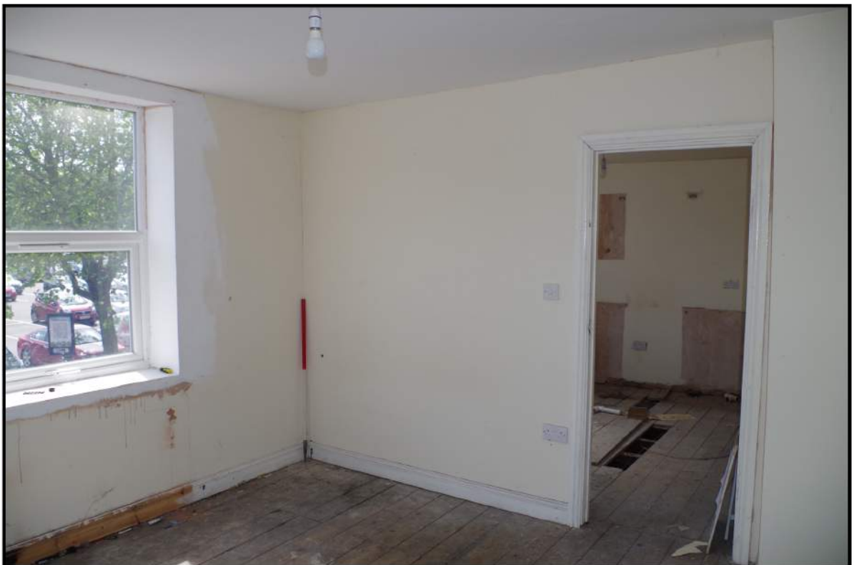
Fig 28: First floor, room 11
