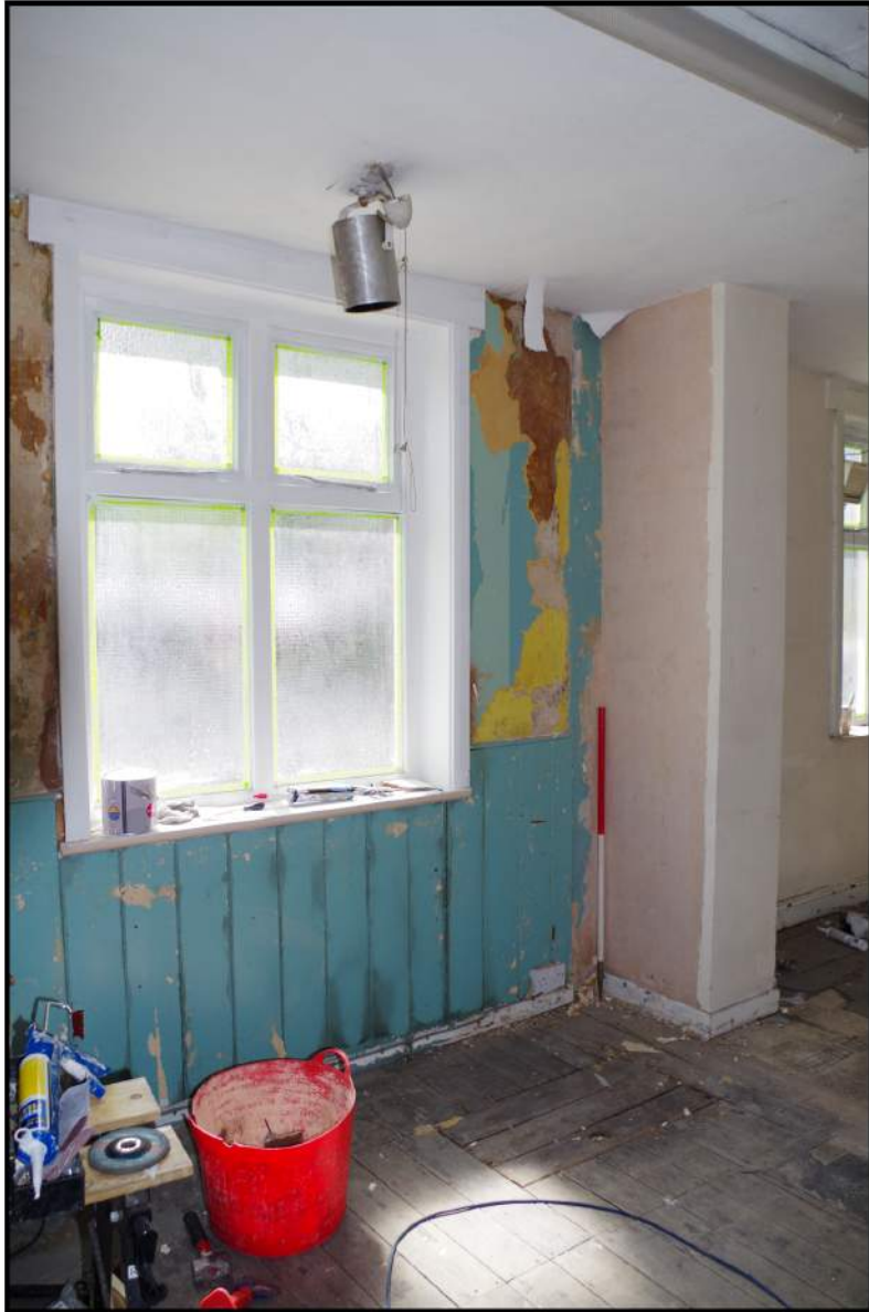
Fig 16: Ground floor, room 1; detail of wall cladding
