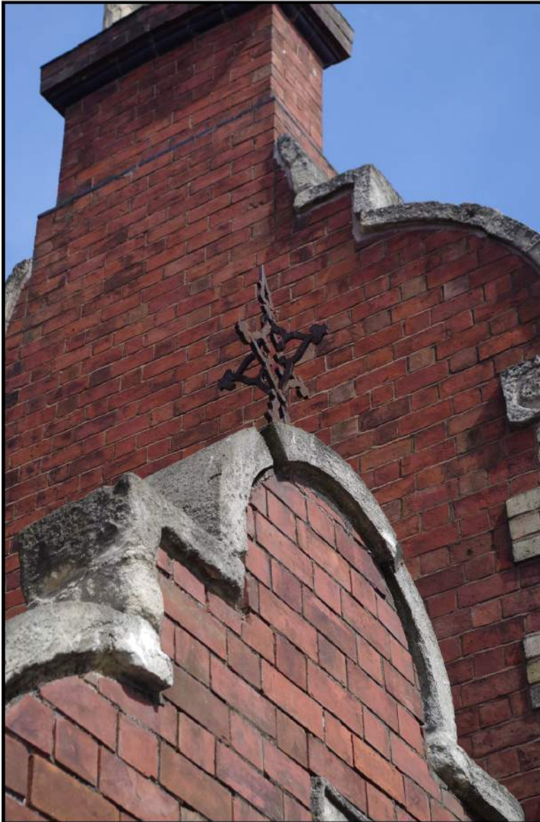
Fig 11: Detail of iron finial on east elevation
