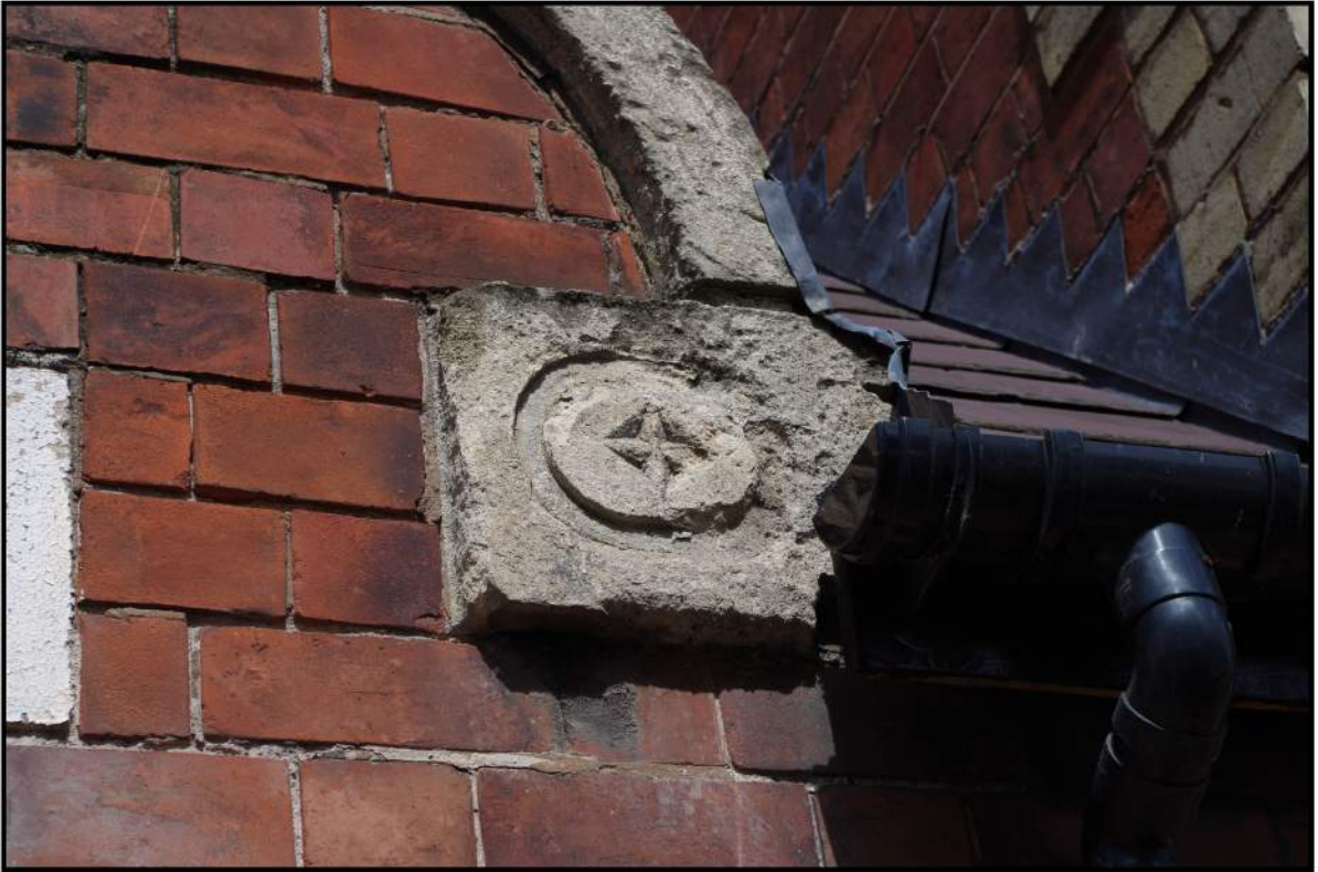
Fig 12: Detail of decorated springing stone on east elevation
