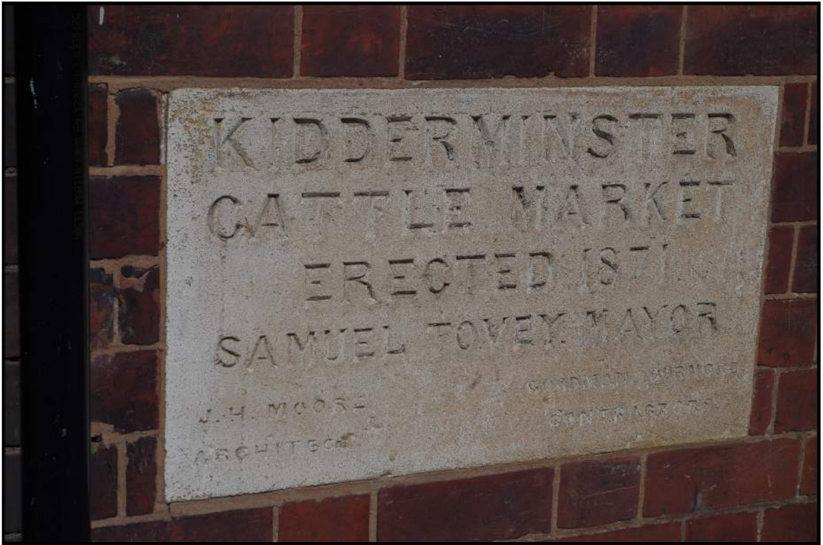
Fig 14: Dedication stone on east elevation
