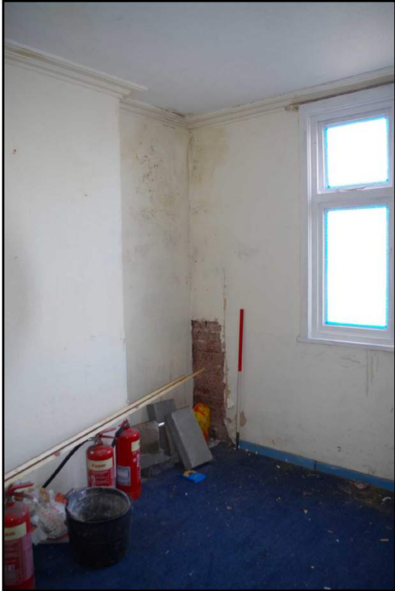
Fig 23: Ground floor, room 7
