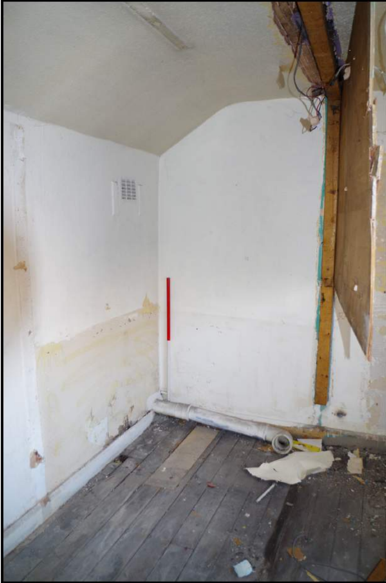
Fig 26: First floor, room 13
