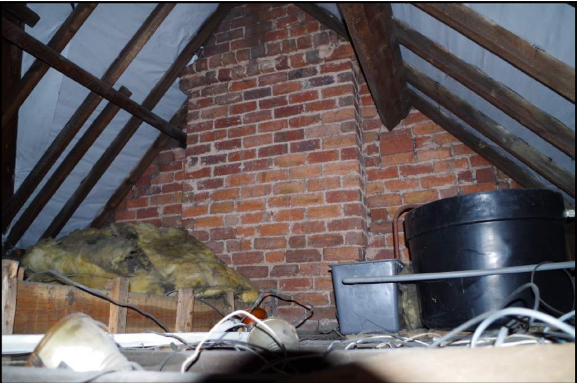
Fig 30: Roof space; showing common rafter roof with purlins
