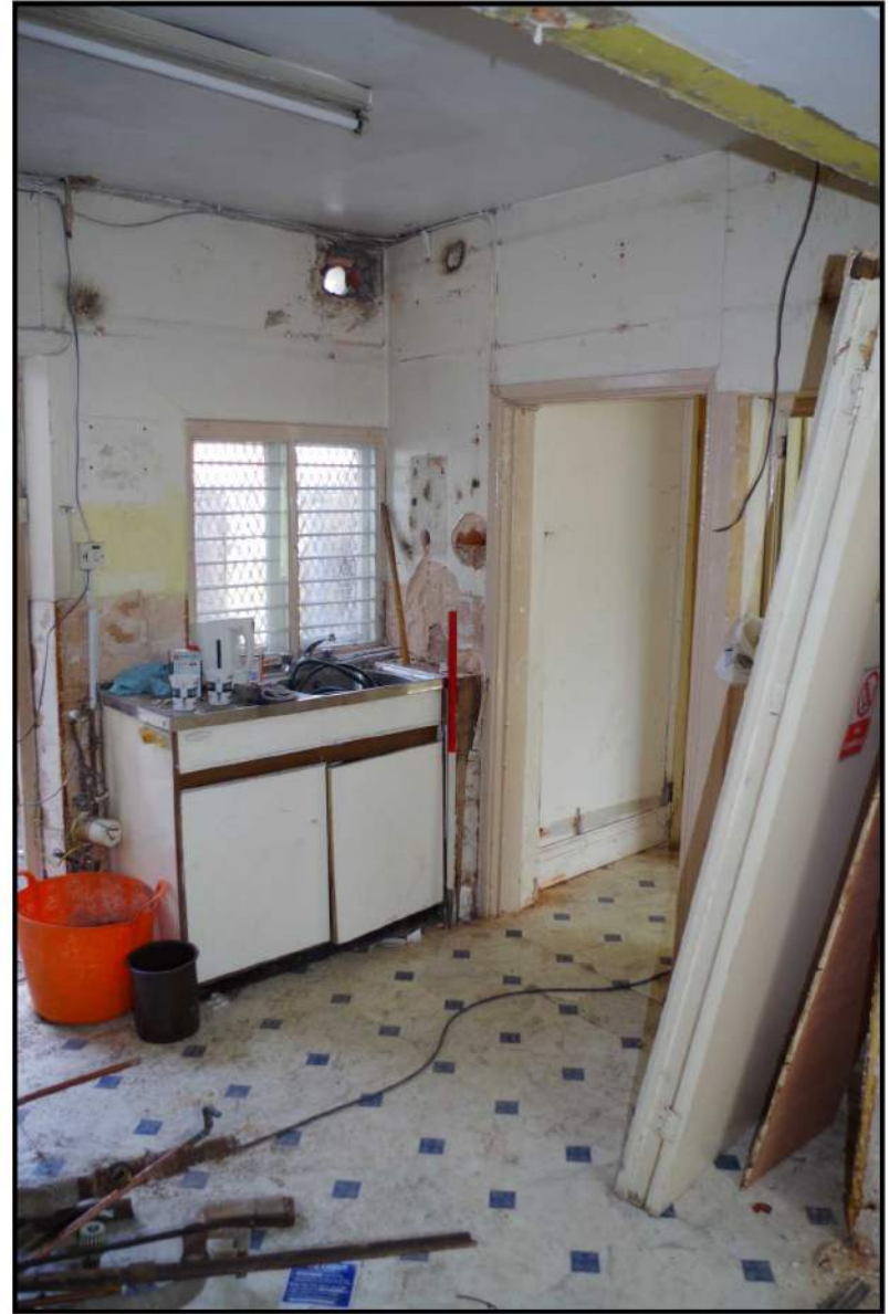
Fig 22: Ground floor, room 5
