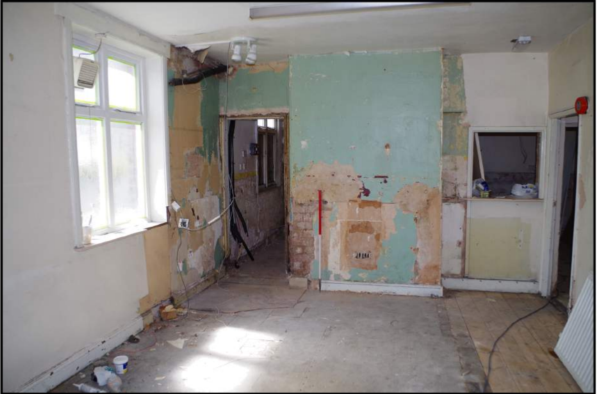
Fig 17: Ground floor, room 2
