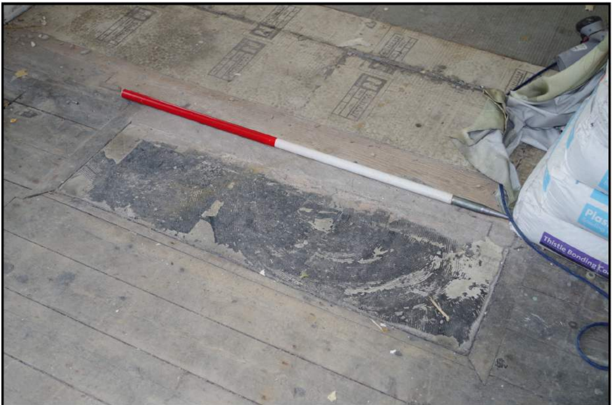
Fig 15: Ground floor, room 1; position of former hearth
