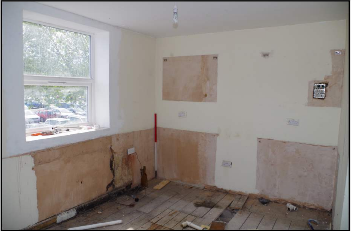
Fig 27: First floor, room 10
