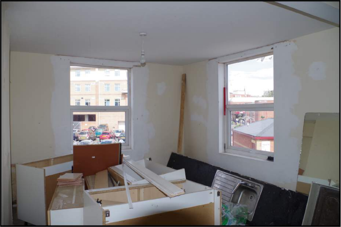
Fig 29: First floor, room 12
