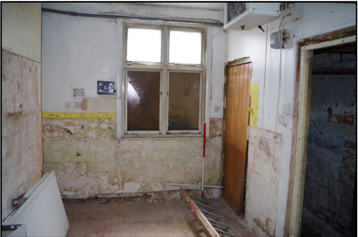
Fig 18: Ground floor, room 3
