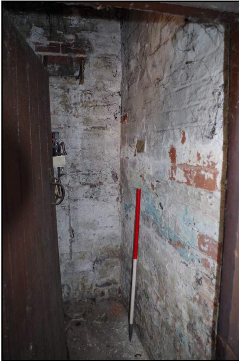
Fig 19: Ground floor, room 4
