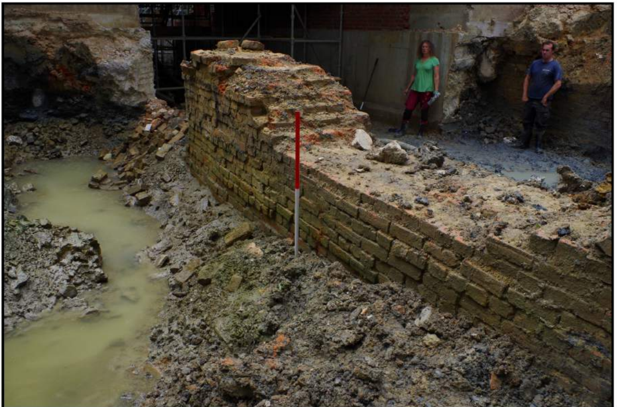
Fig 9: Rear of south-east abutment wall showing English bond brickwork
