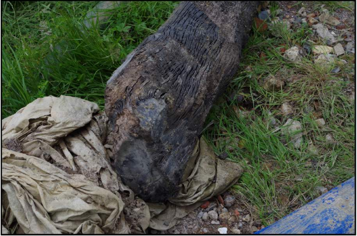
Fig 12: Timber found between abutment walls showing detail of 'spade' end
