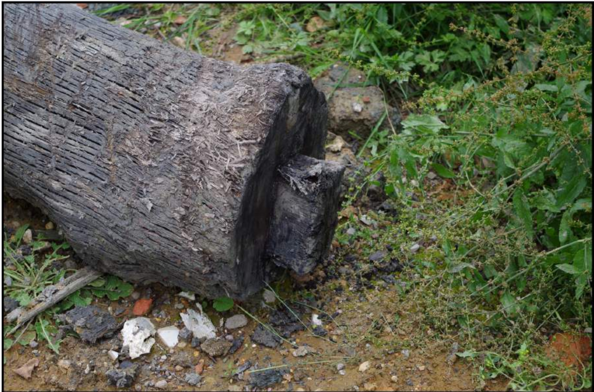
Fig 11: Timber found between abutment walls showing detail of tenon
