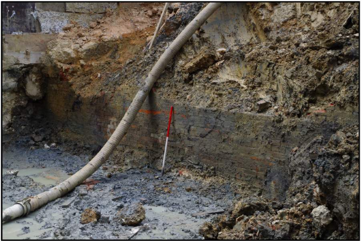
Fig 7: North-west abutment wall
