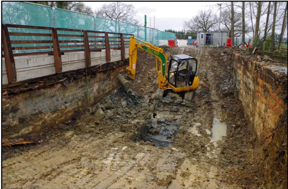
Fig 5: General view of excavation of causeway from south-east
