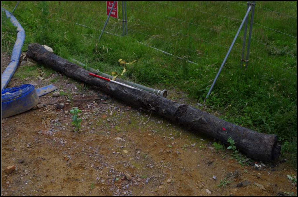
Fig 10: Timber found between abutment walls
