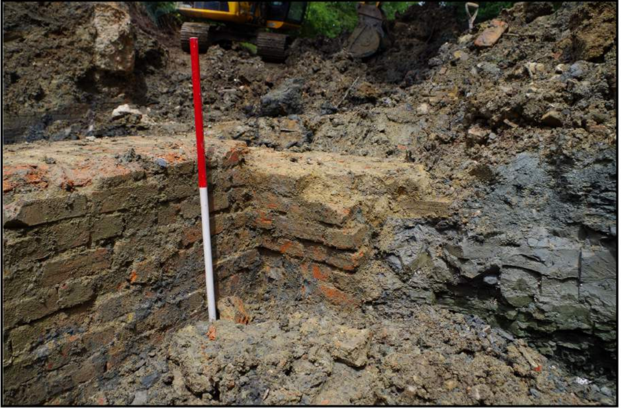
Fig 8: South-east abutment wall showing buttress
