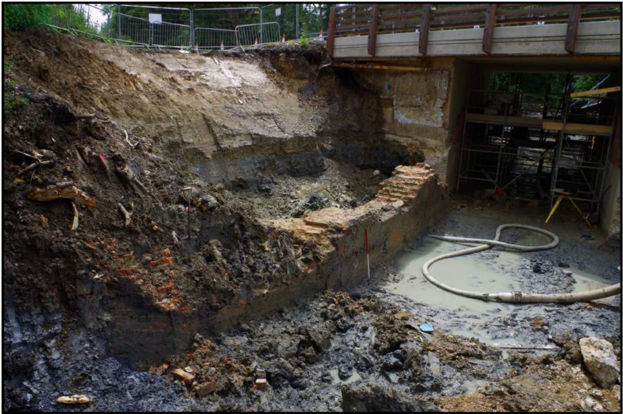
Fig 6: South-east abutment wall
