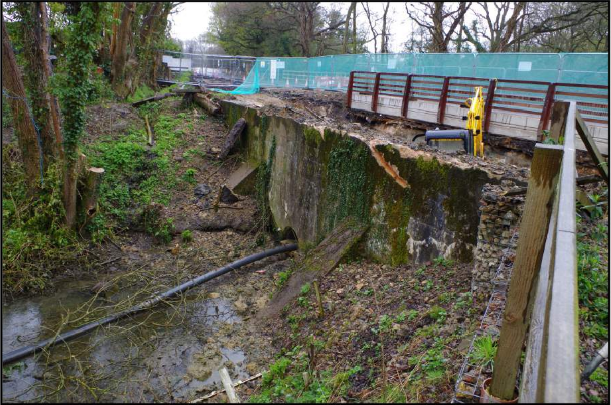
Fig 4: General view of north-east side of causeway showing culvert
