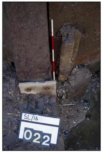
Fig 15: Context 022; early pattern rail, possible part of turf lock
