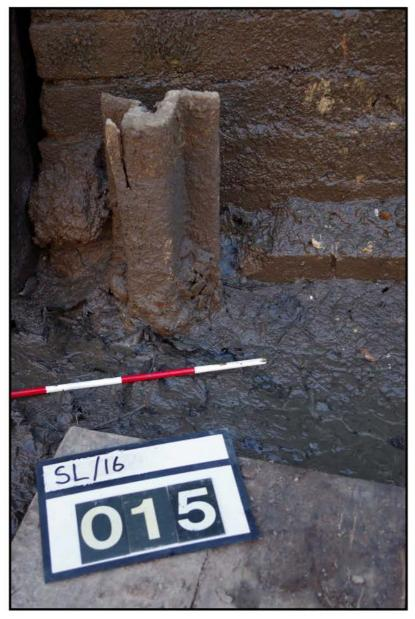
Fig 8: Context 015; early pattern rail, possible part of turf lock
