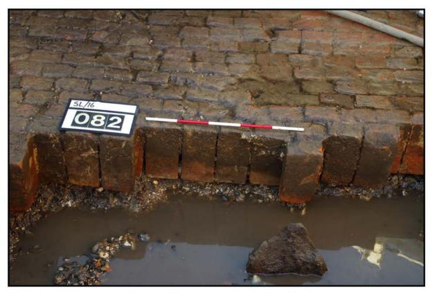
Fig 59: Context 082; rounded flint gravel (natural subsoil) underlying brick invert
