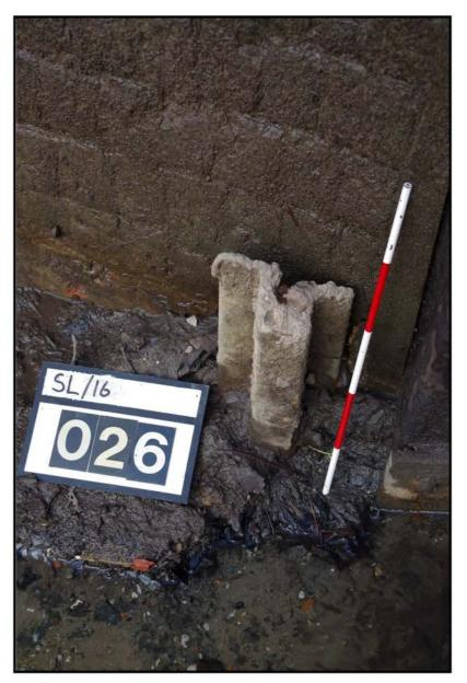
Fig 19: Context 026; early pattern rail, possible part of turf lock
