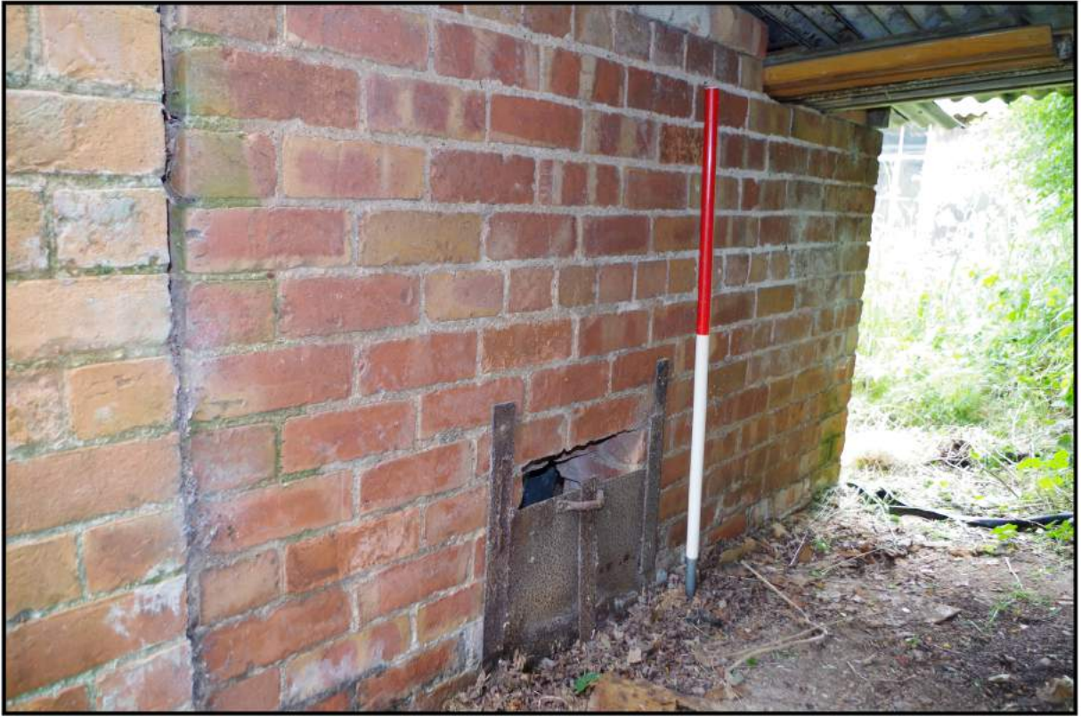
Fig 26: Hatch access to rear of pig sty
