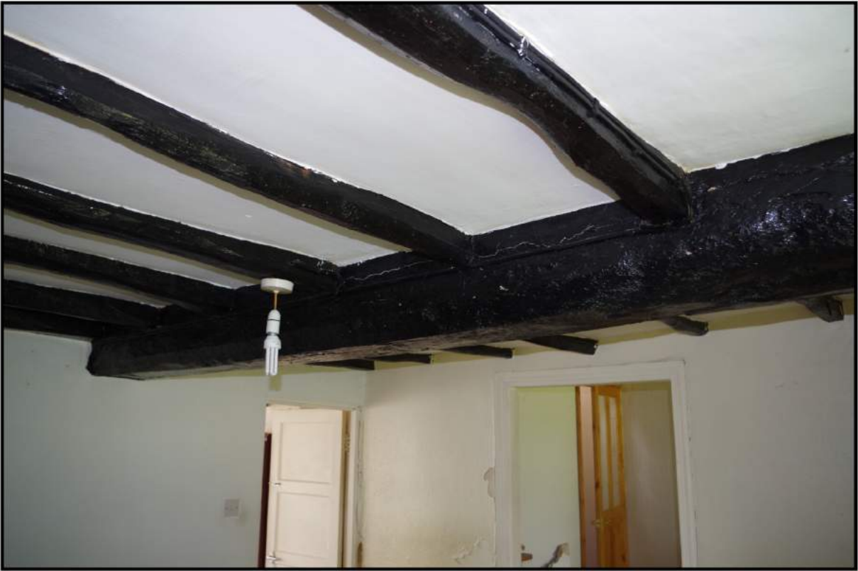
Fig 14: Phase 2, ground floor; showing massive timber supporting first floor
