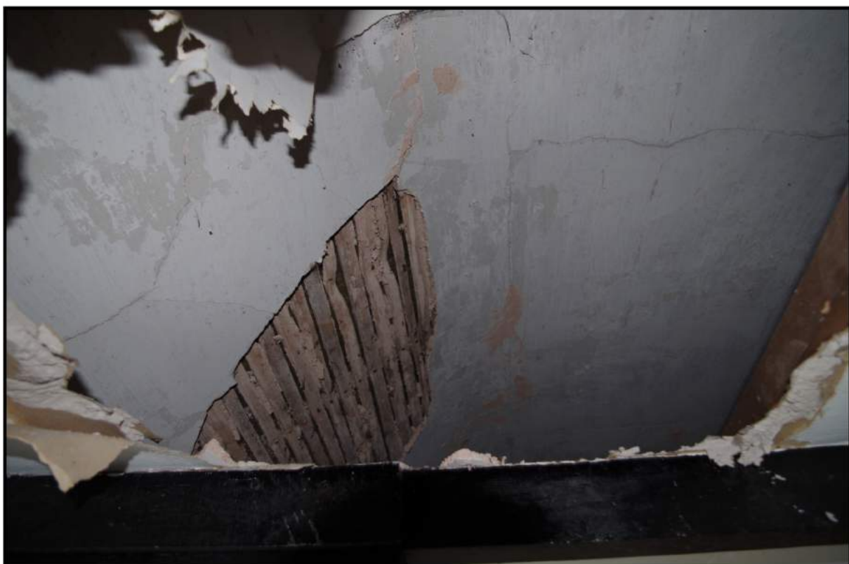
Fig 11: Phase 1, first floor; showing lathe and plaster ceiling
