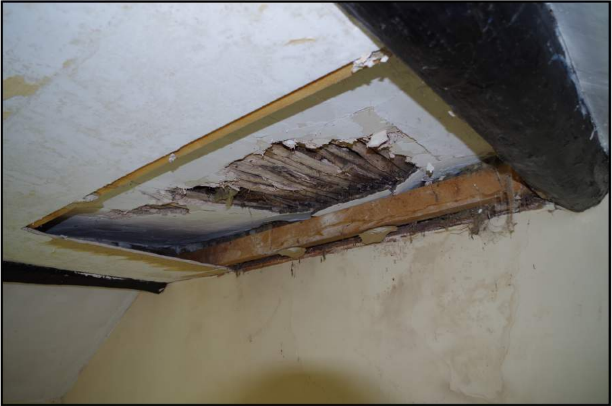
Fig 16: Phase 2, first floor; showing lath and plaster ceiling
