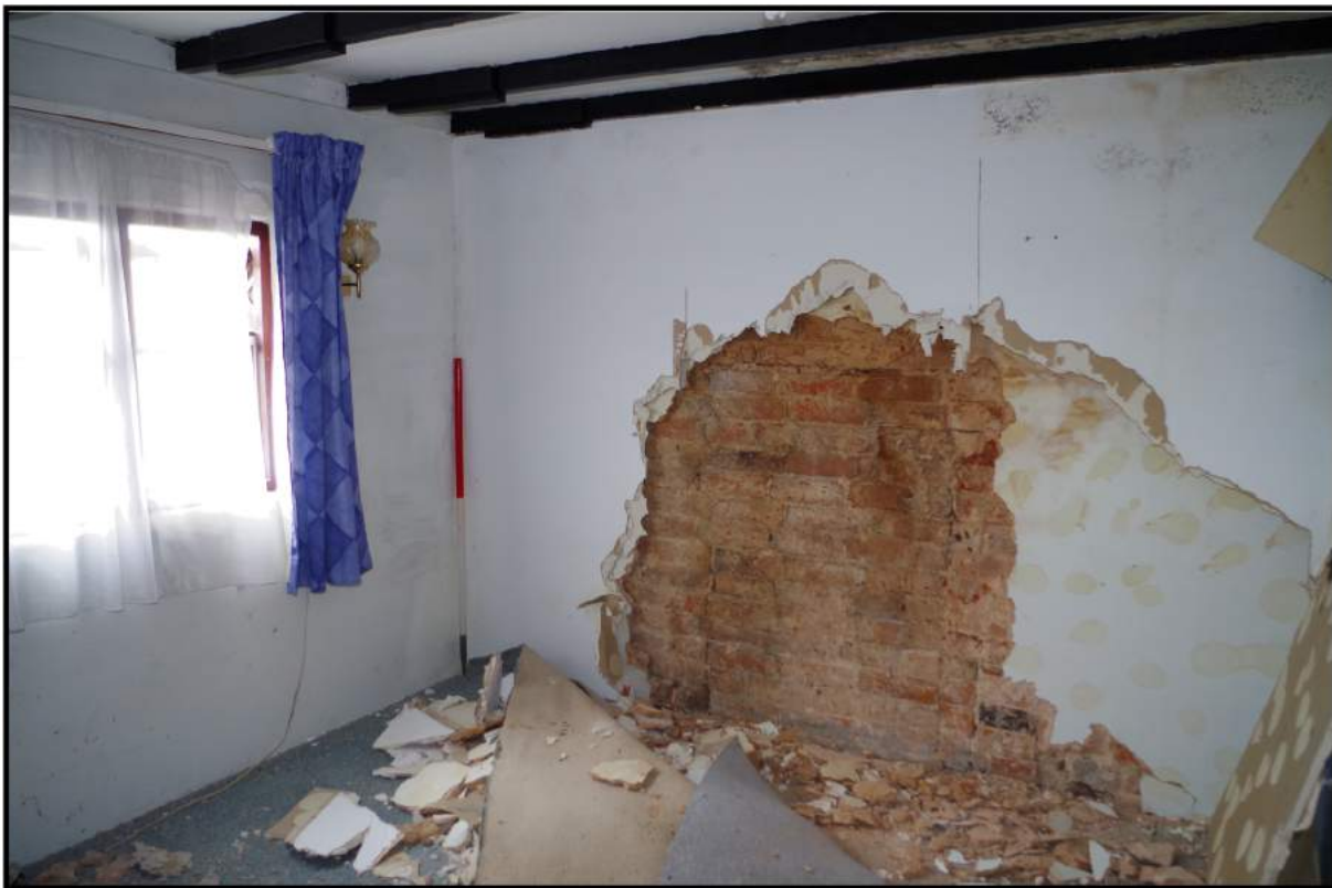
Fig 10: Phase 1, first floor; showing blocked fireplace
