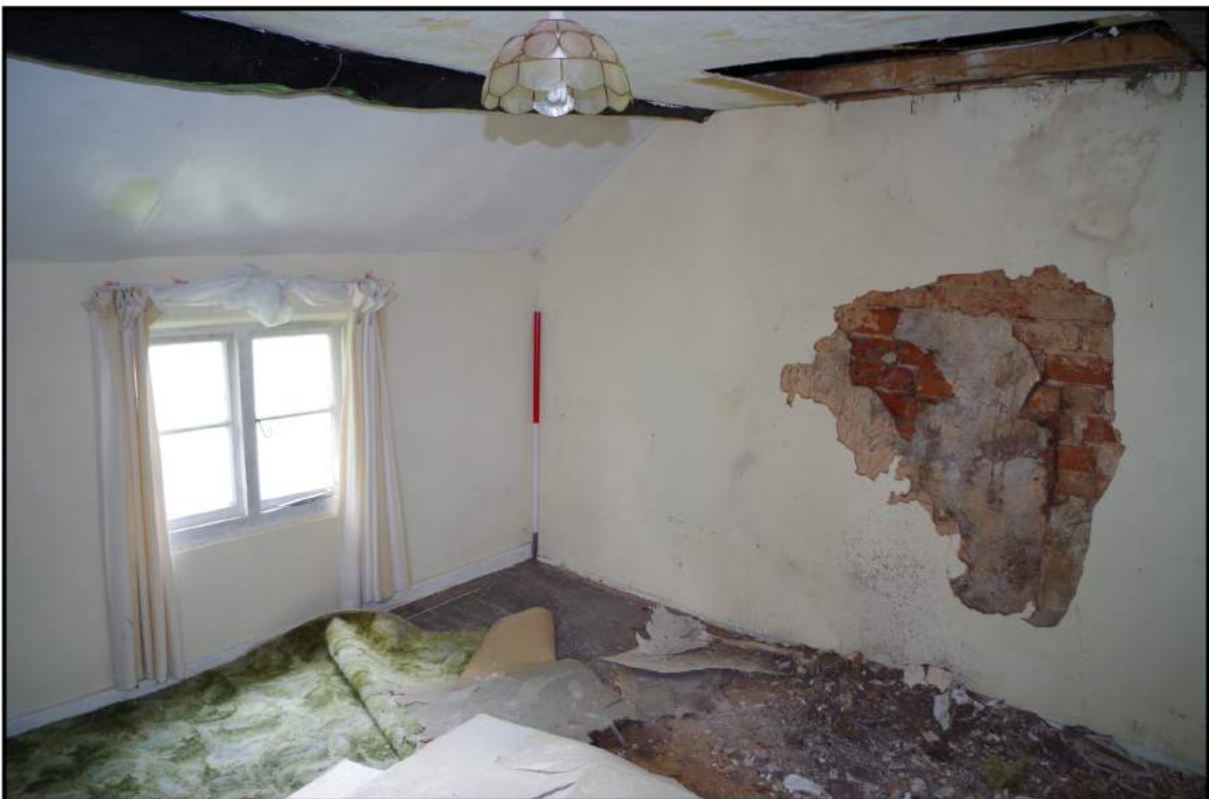
Fig 15: Phase 2, first floor; showing blocked fireplace
