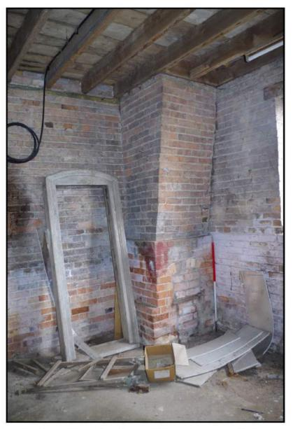
Fig 16: Ground floor of production building showing detail of hearth and chimney
