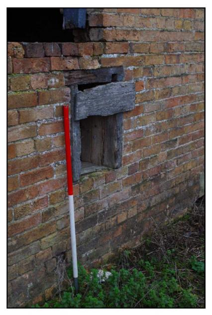
Fig 14: East elevation of production building showing opening for tractor belt drive
