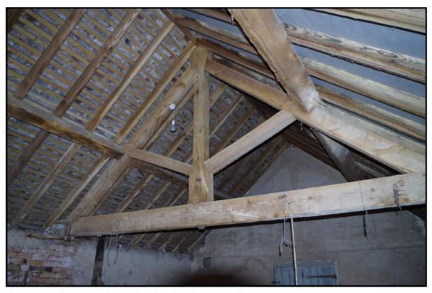
Fig 26: First floor of production building showing detail of roof truss
