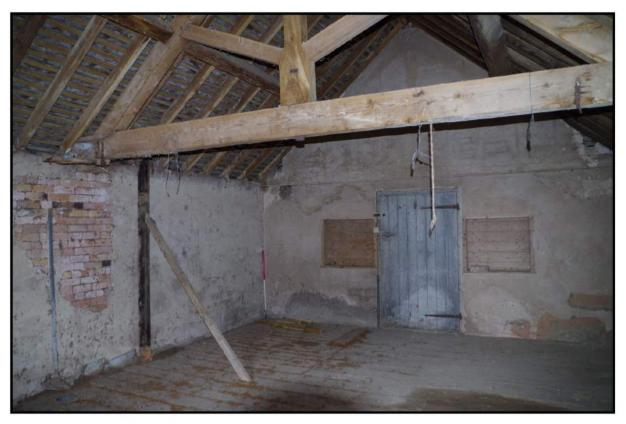
Fig 24: First floor of production building showing hatches and door to hop drying compartment
