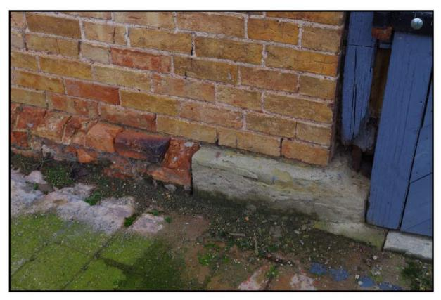
Fig 32: View of footings of barn to east showing evidence that farmstead was rebuilt, substantially on same plan
