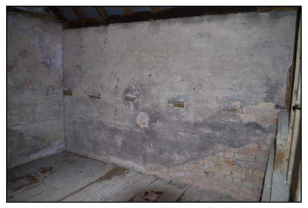
Fig 29: First floor of production building showing wood blocks inserted in wall bond
