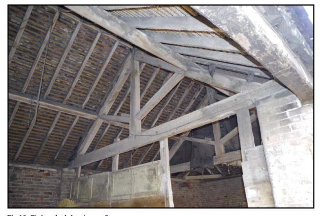
Fig 19: Shelter shed showing roof truss
