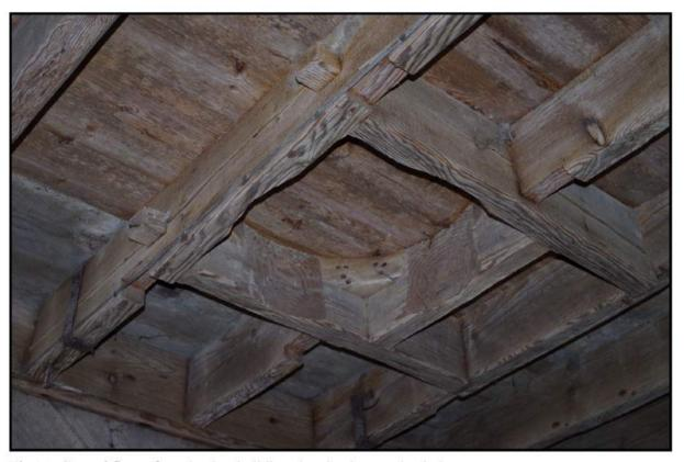
Fig 18: Ground floor of production building showing hop pocket hole
