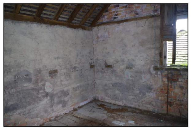
Fig 27: First floor of production building showing area where flue from ground floor enters and wood blocks inserted in wall bond
