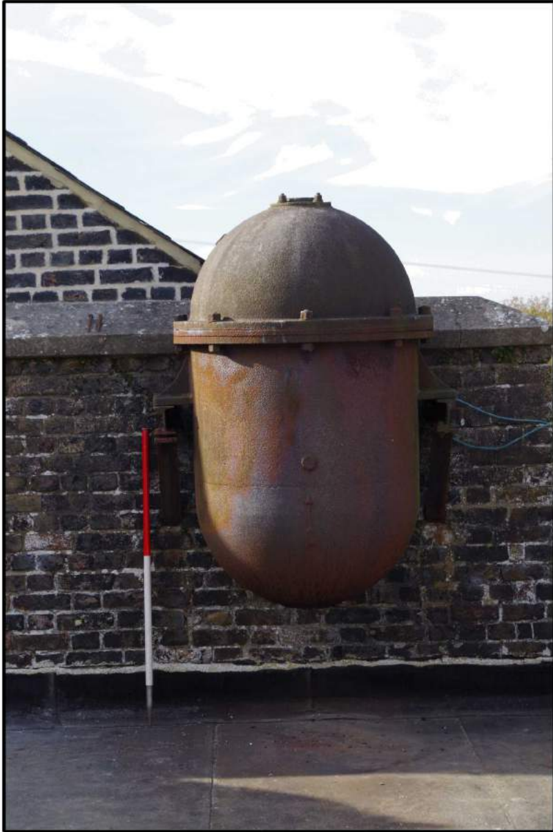
Fig 3: Northern muffler; view from east
