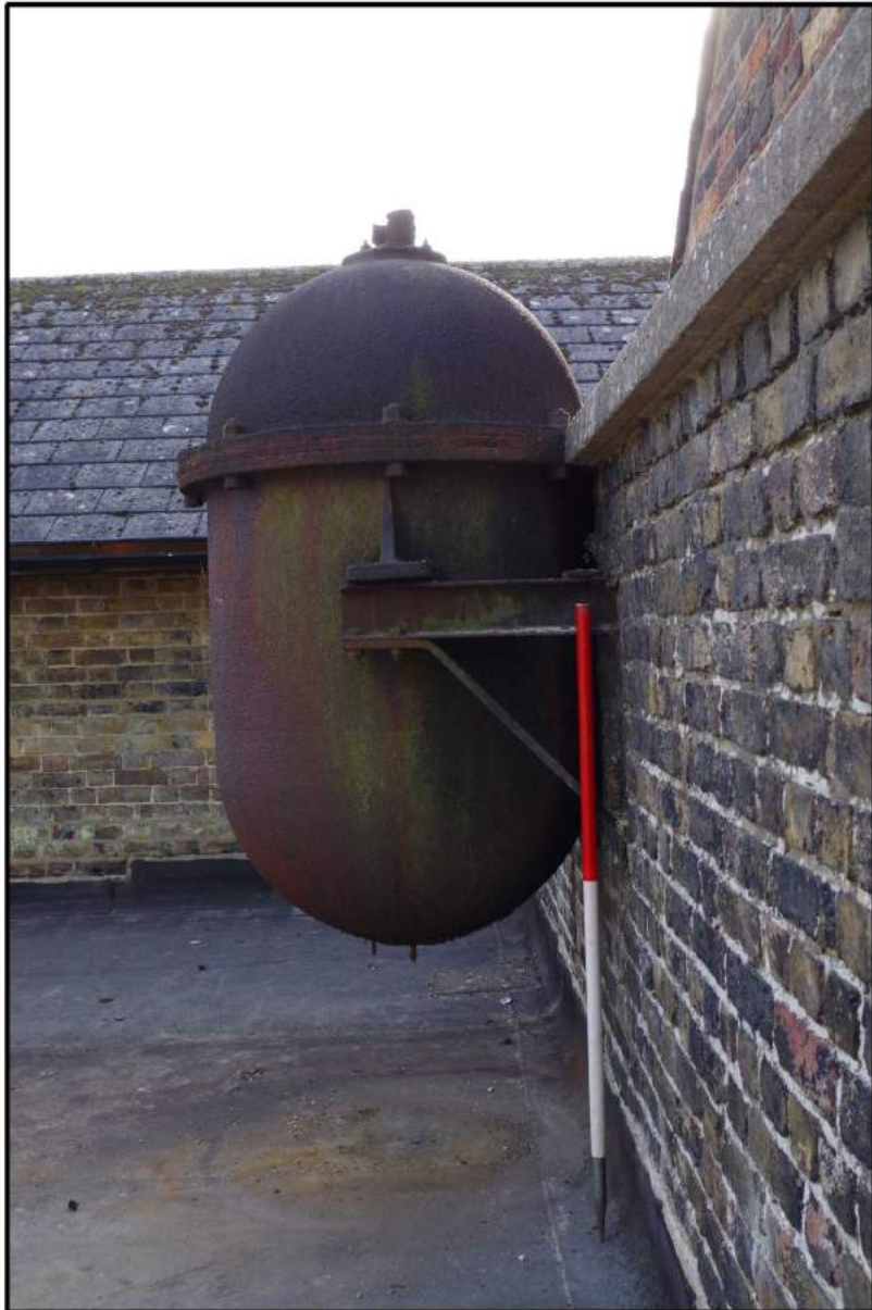
Fig 5: Southern muffler; view from north
