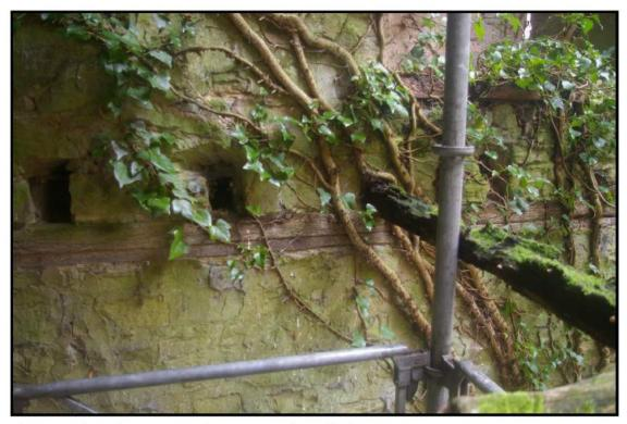
Fig 27: Sockets for transverse beam supporting galleries
