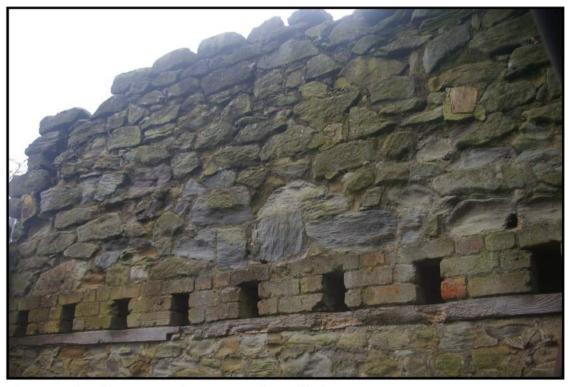
Fig 24: Sockets for transverse beam supporting galleries
