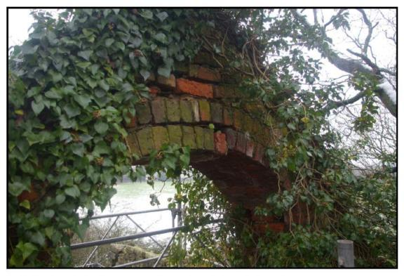
Fig 9: North-east elevation showing damage to arch above bob opening
