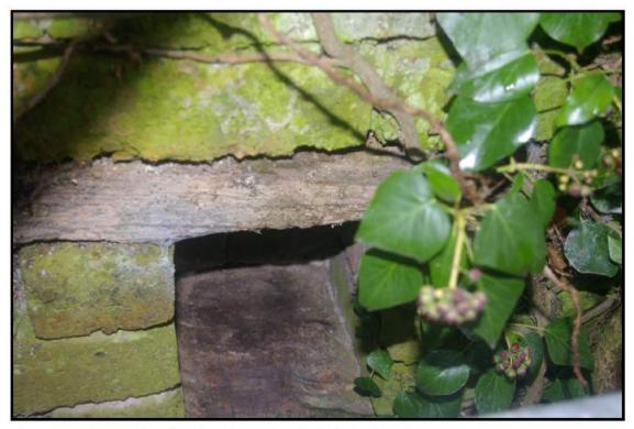
Fig 13: North-east elevation showing socket for bob platform
