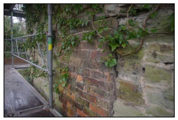
Fig 19: South-east elevation showing blocked opening
