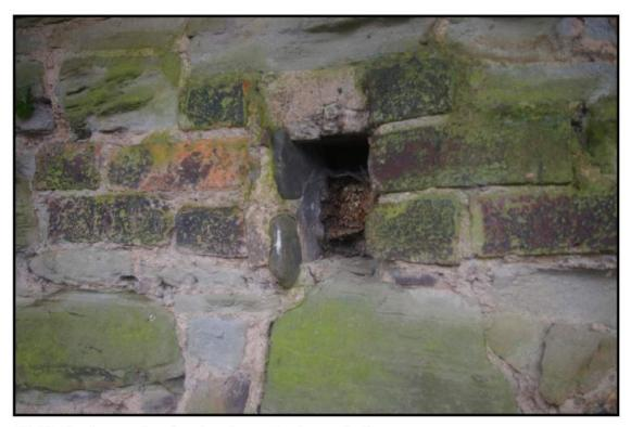
Fig 20: South-east elevation showing socket for attached structure
