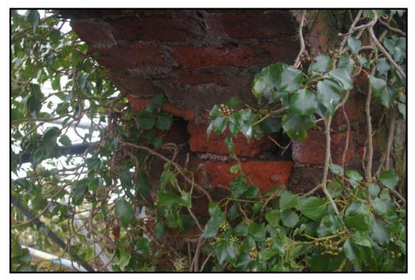
Fig 10: North-east elevation showing holes for formwork under bob opening arch
