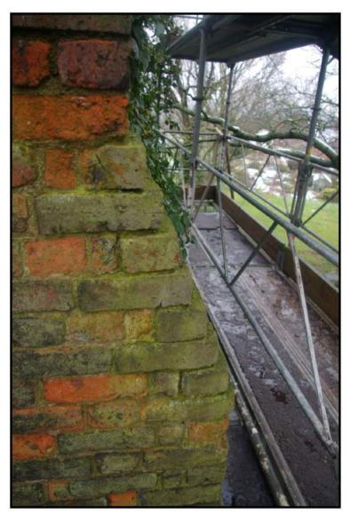
Fig 14: South-east elevation showing stepped brickwork
