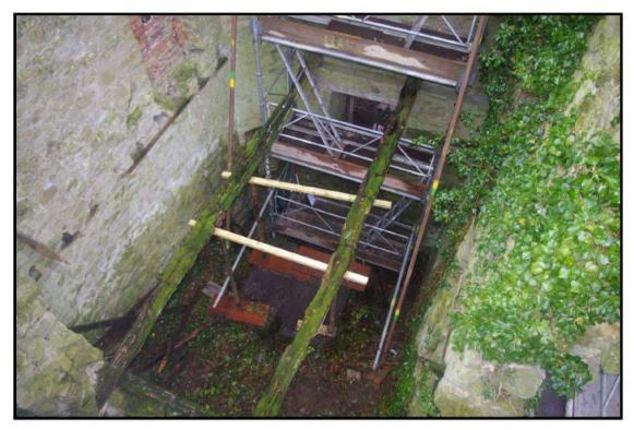
Fig 29: View from top of engine house showing longitudinal beams
