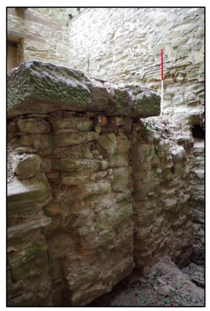
Fig 38: Phase 2 engine loading showing grooves for holding-down bolts
