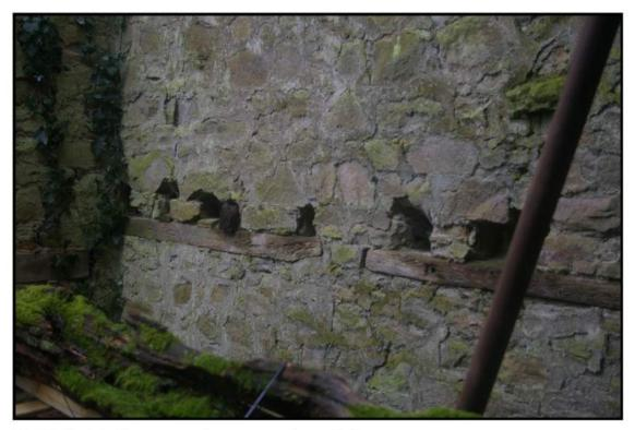
Fig 25: Sockets for transverse beam supporting galleries
