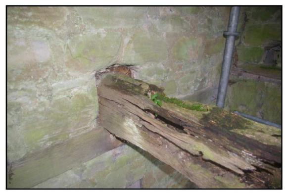
Fig 23: Longitudinal timber supporting the top of the cylinder
