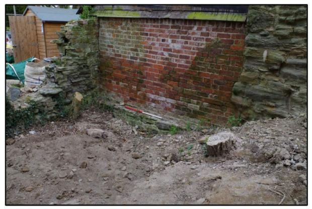
Fig 41: Showing Phase 4 structure sitting upon remaind of Phase 3 structure
