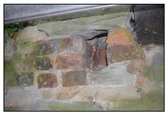
Fig 18: South-east elevation showing socket for attached structure
