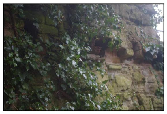
Fig 26: Sockets for transverse beam supporting galleries
