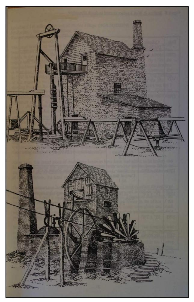
Fig 4.15: Typical examples of a pumping engine (top) and a winding engine (bottom) after Shropshire Caving and Mining Club, account no 18
