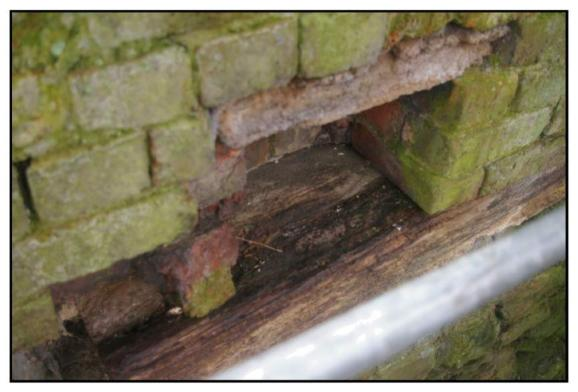
Fig 11: North-east elevation showing socket for bob platform
