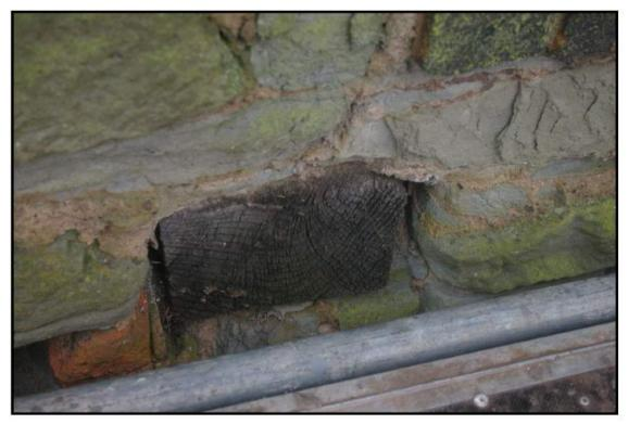
Fig 17: South-east elevation showing timber formerly supporting bob pivot
