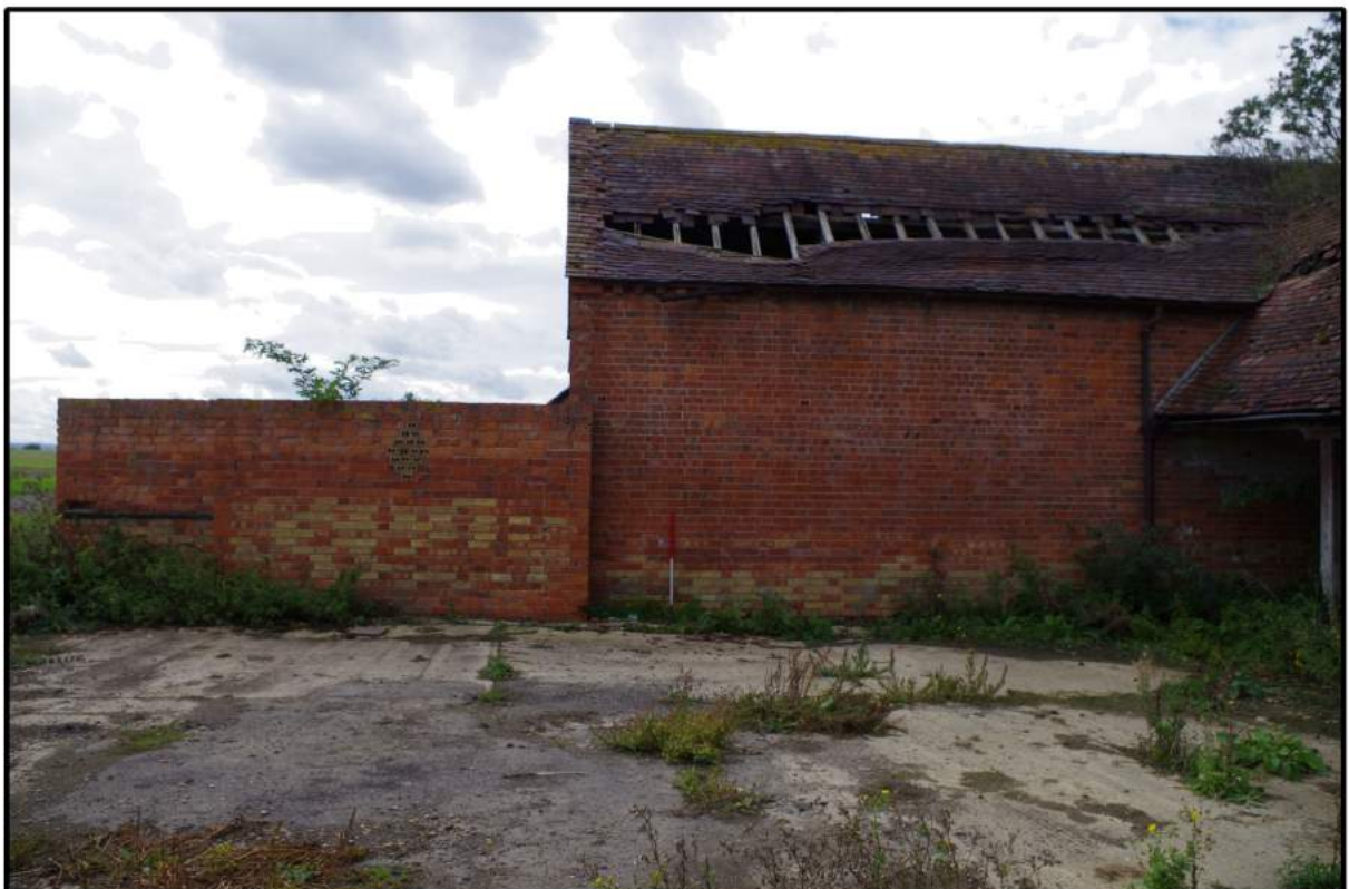
Fig 12: North-north-east elevation showing yellow bricks
