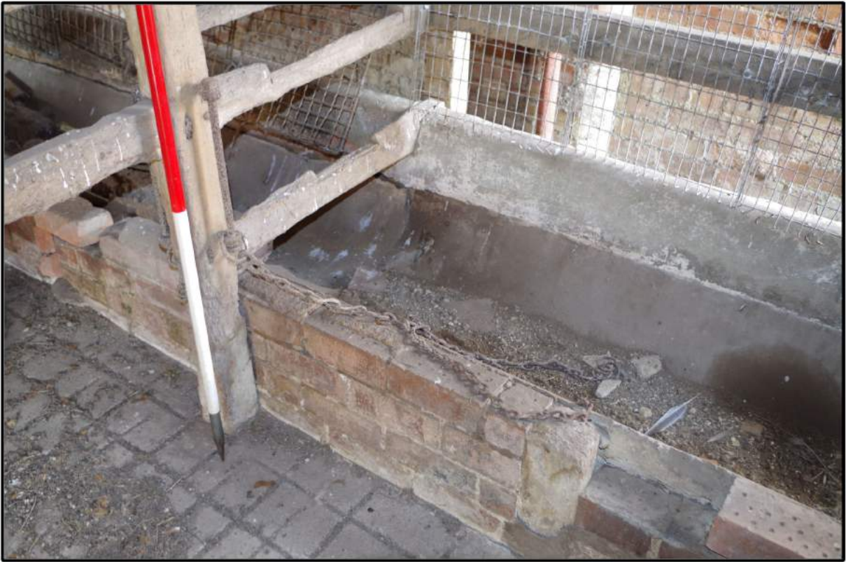
Fig 19: Interior, north end, showing detail of restraining chain
