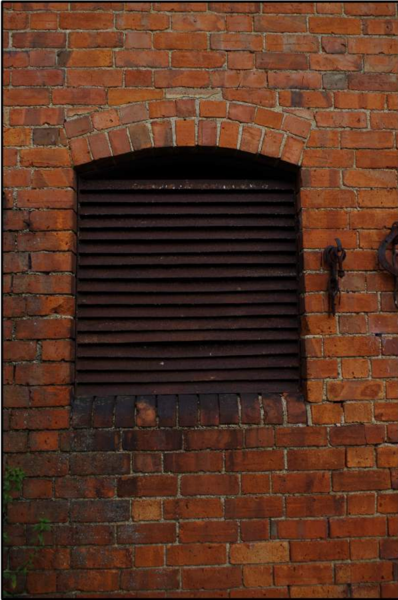
Fig 15: South-south-west elevation, detail of metal louvres
