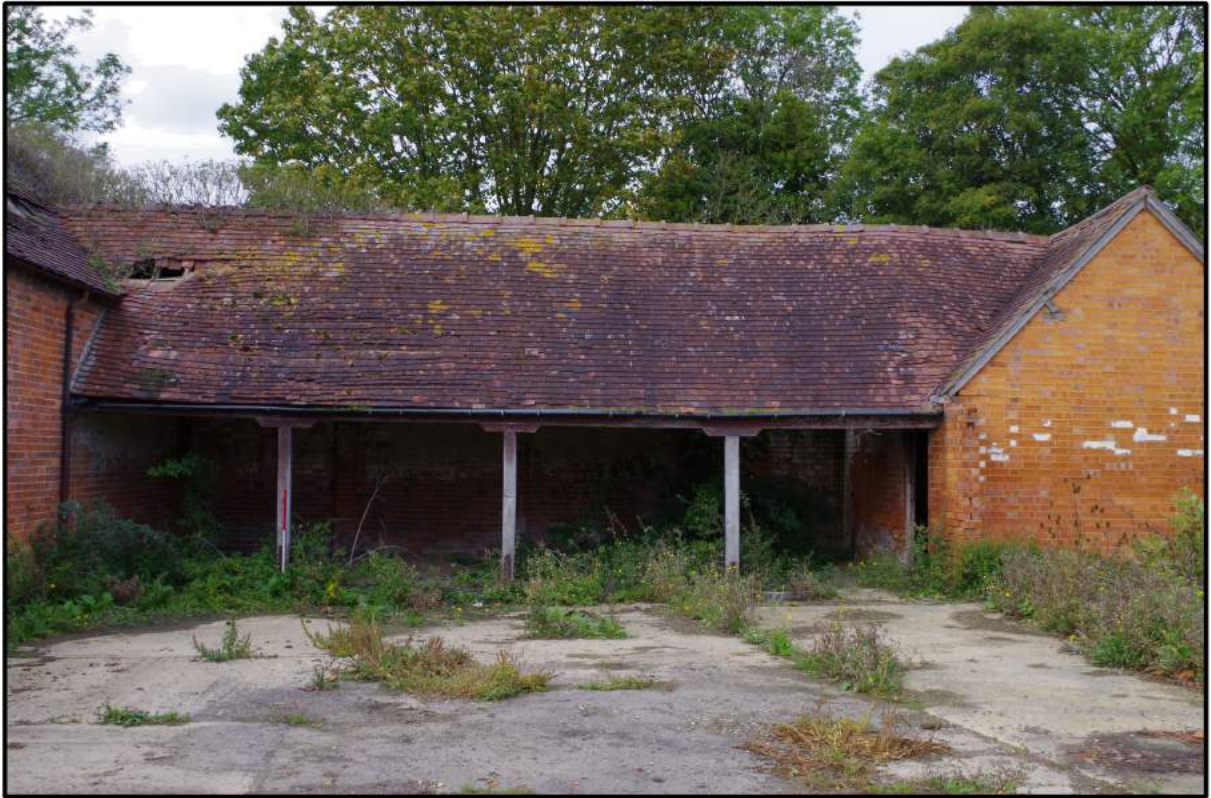
Fig 11: South-south-east elevation, north end
