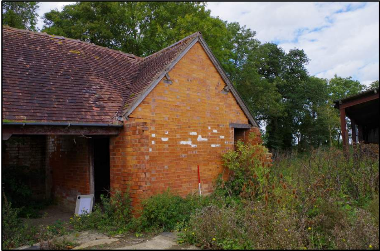
Fig 9: South-south-east elevation, north end gable
