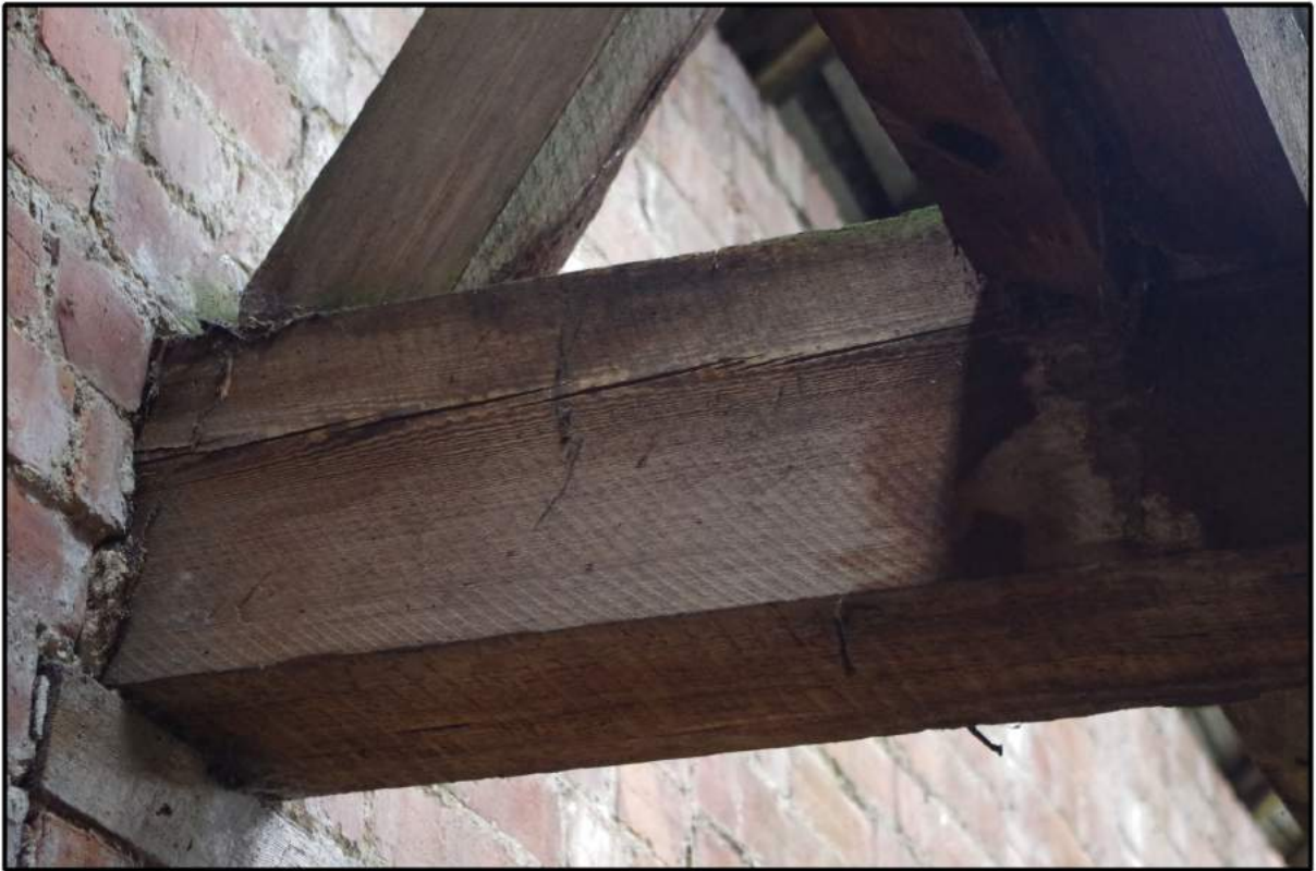
Fig 31: Central block, interior, showing circular saw marks on tie beam
