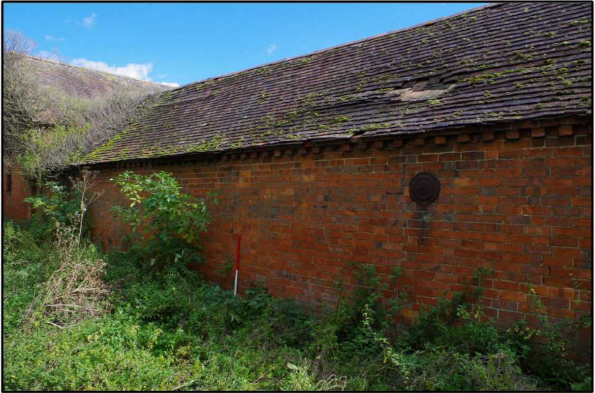
Fig 4: West-north-west elevation, southern end
