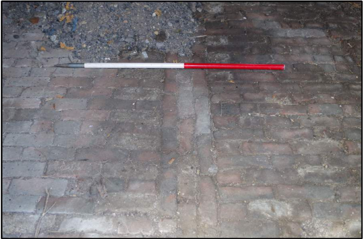
Fig 30: Central block, interior, showing muck channel
