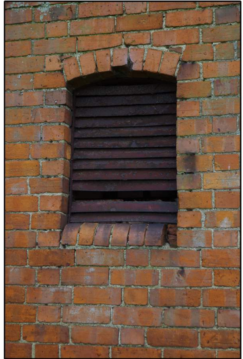
Fig 7: West-north-west elevation, central gable, detail of louvres
