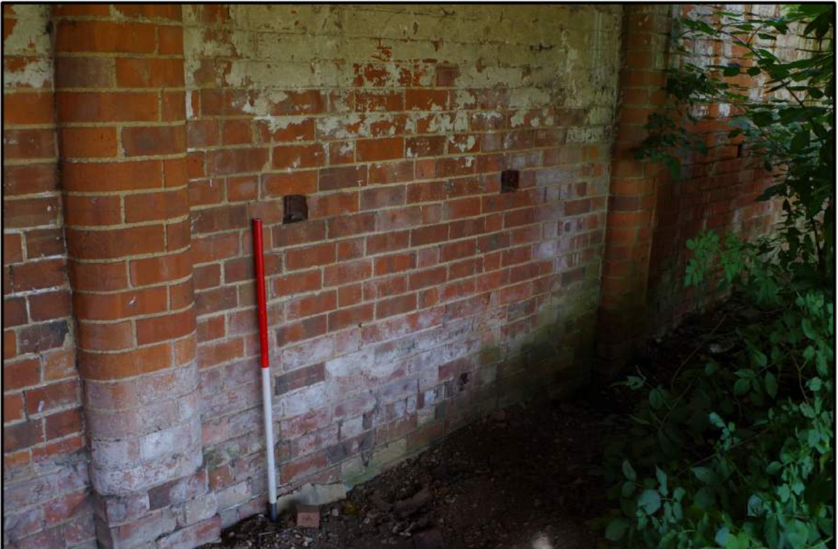
Fig 26: North end interior showing sockets for trough and limewash
