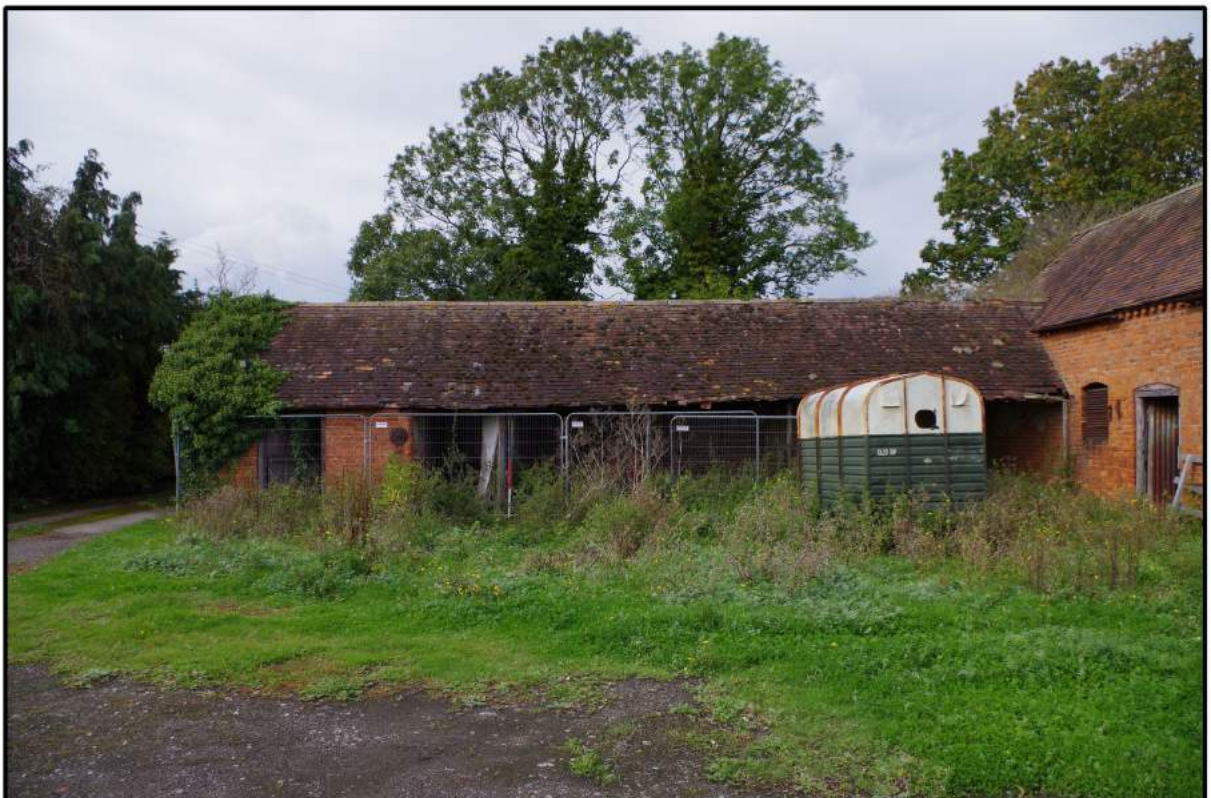
Fig 17: East-south-east elevation, south end
