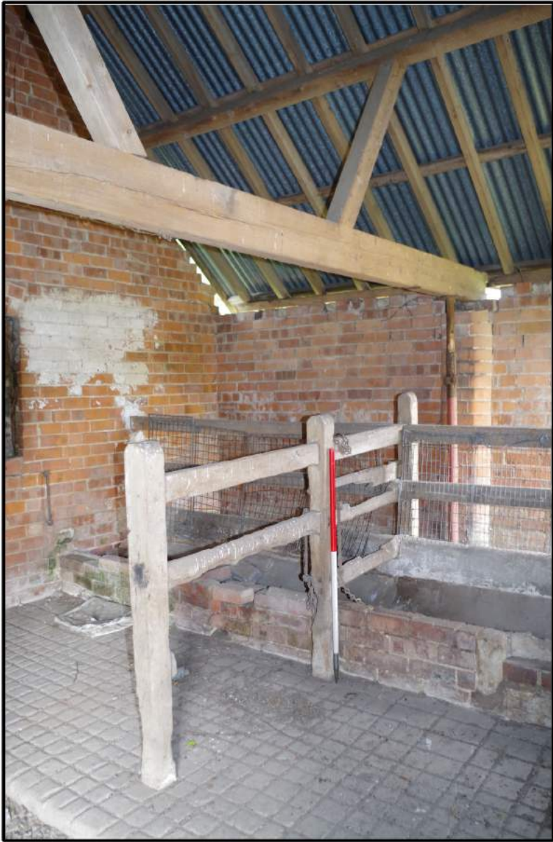
Fig 18: Interior, north end, showing trough and feeding passage
