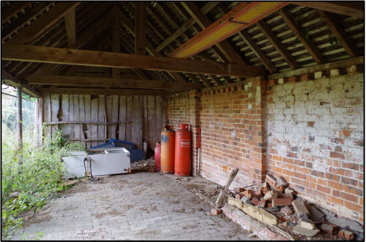
Fig 33: South end interior
