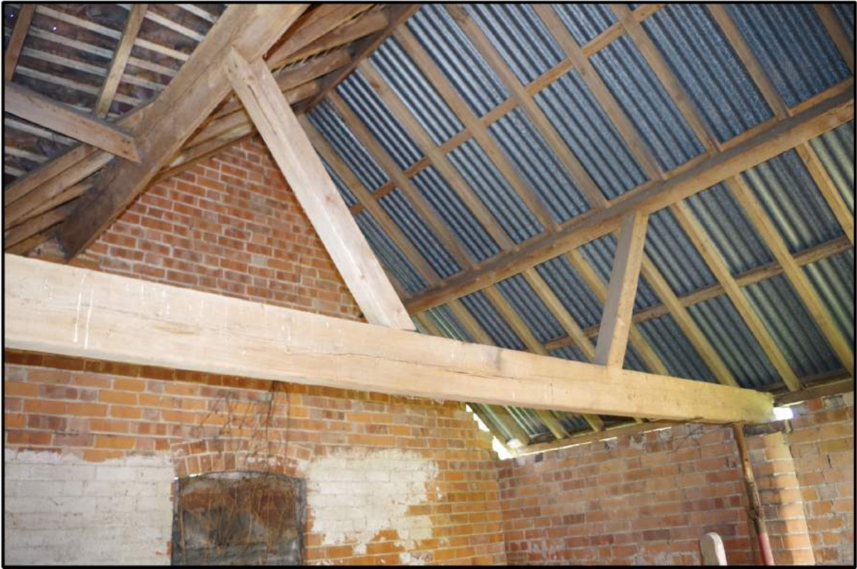
Fig 21: North end roof truss
