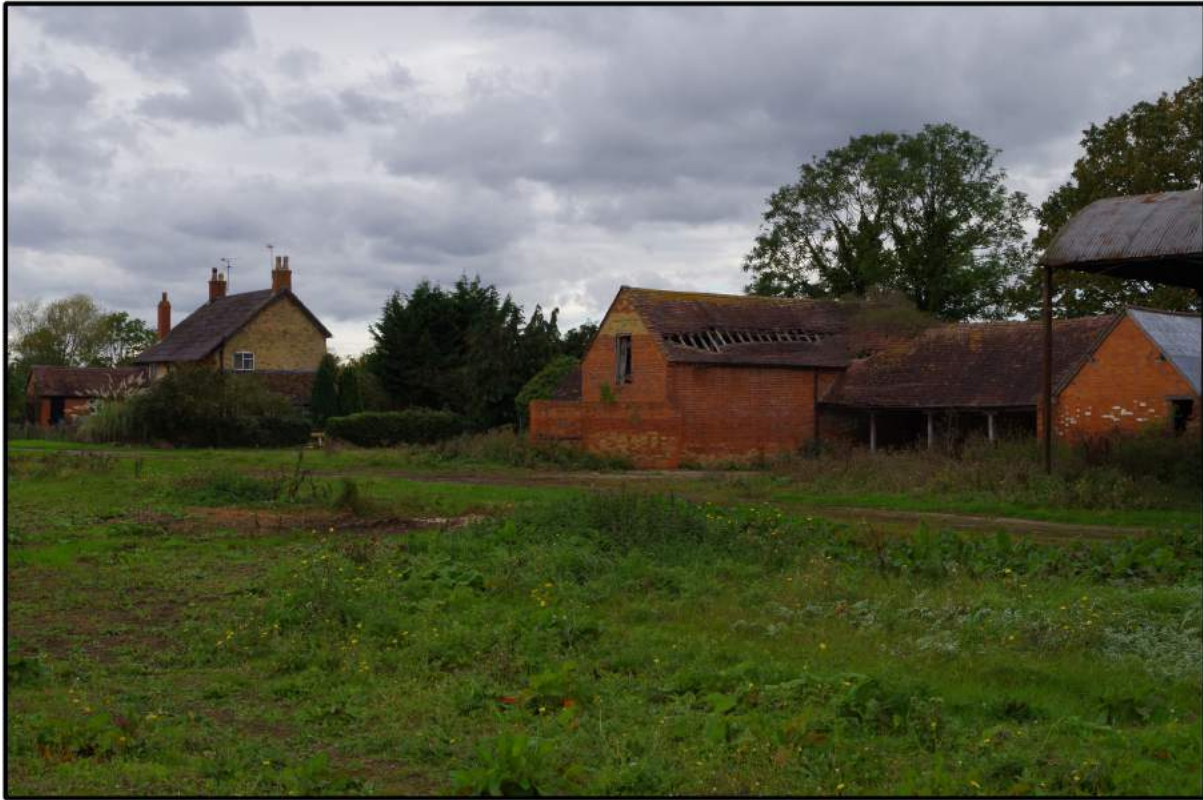
Fig 37: General view from north-east
