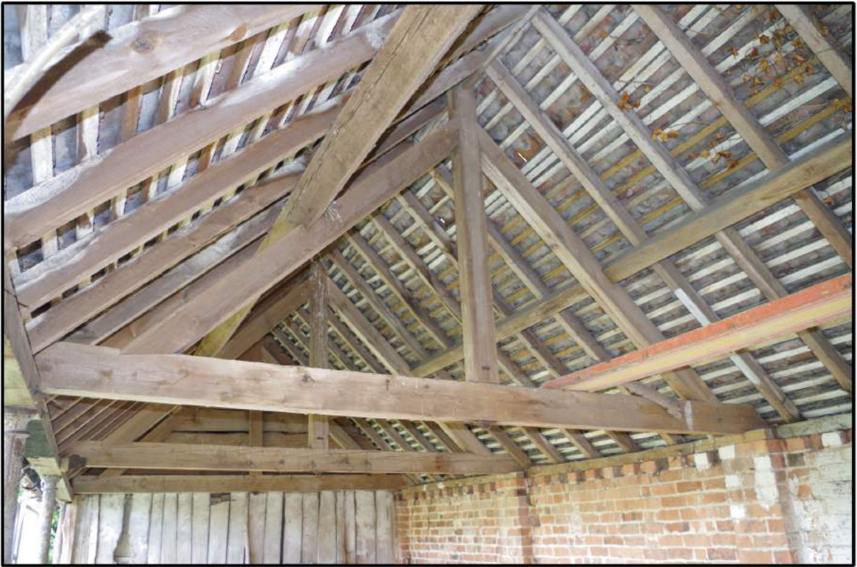
Fig 34: South end, interior, detail of roof truss
