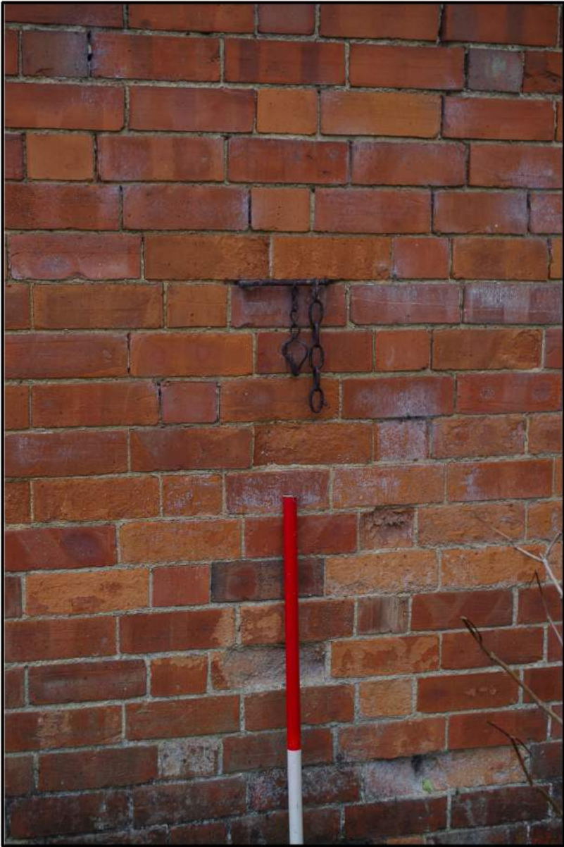
Fig 10: North-north-east elevation, detail of fittings
