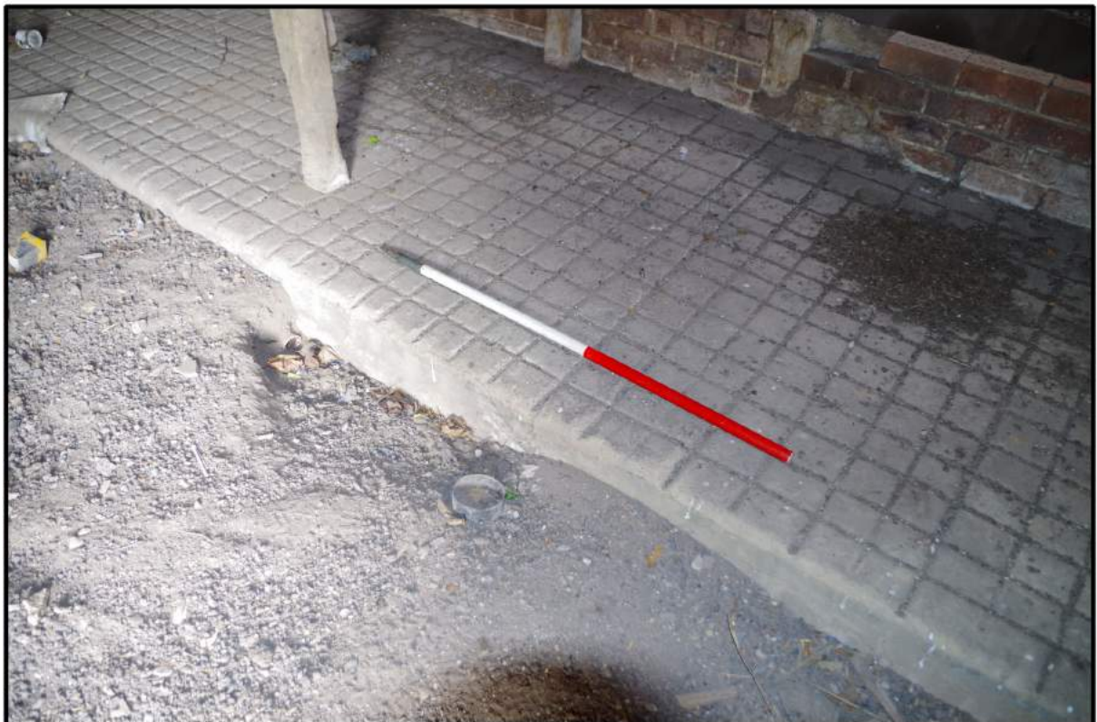
Fig 20: Interior, north end, showing textured concrete floor
