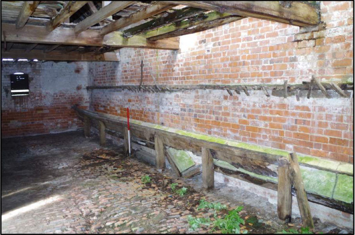
Fig 29: Central block, interior, showing trough, with remains of rack over, and brick floor
