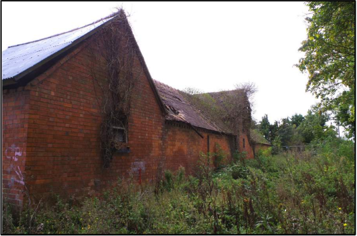
Fig 5: West-north-west elevation, north end
