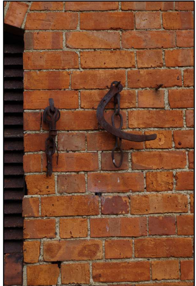
Fig 14: South-south-west elevation showing fittings
