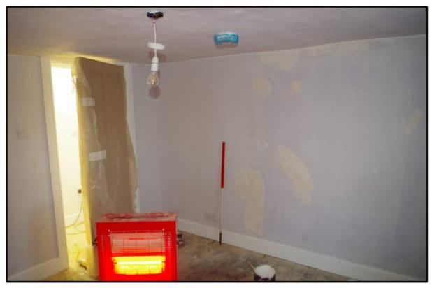
Fig 12: Room 2 showing blocking of former door
