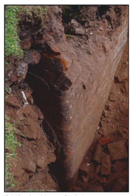
Fig 9: View of rounded corner at foot of stair
