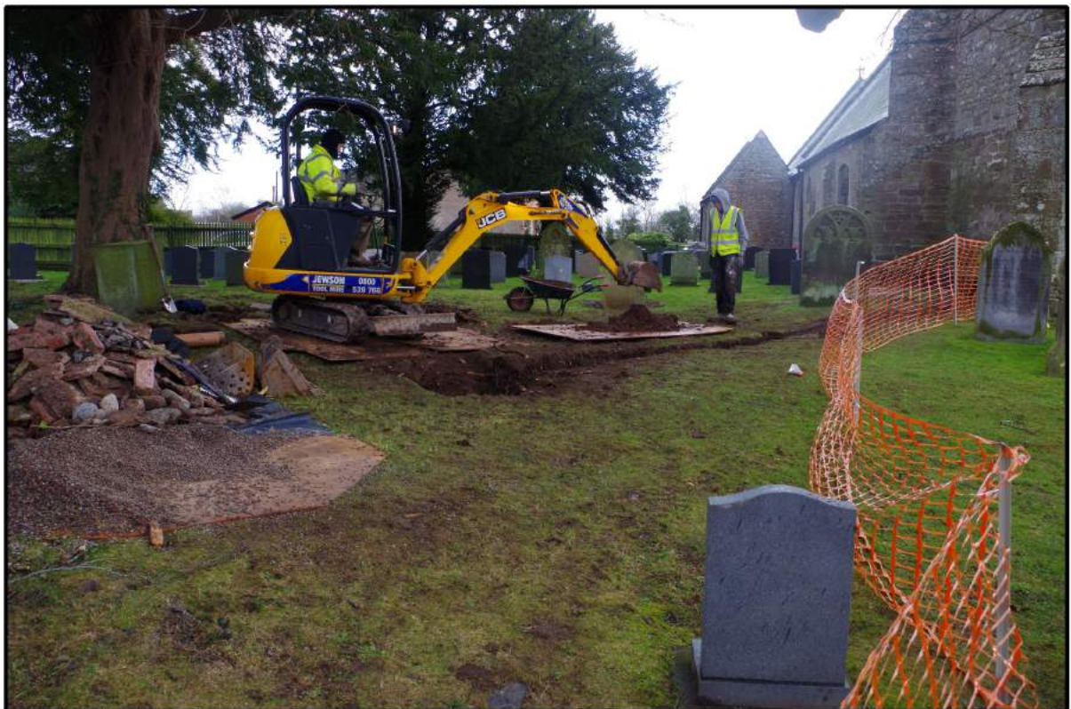
Fig 5: General view of site looking east
