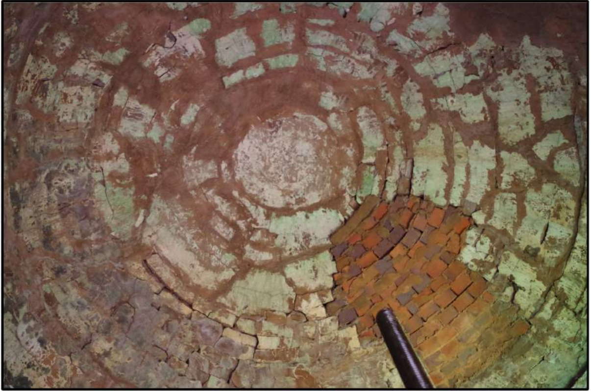
Fig 10: View of the inside of the dome
