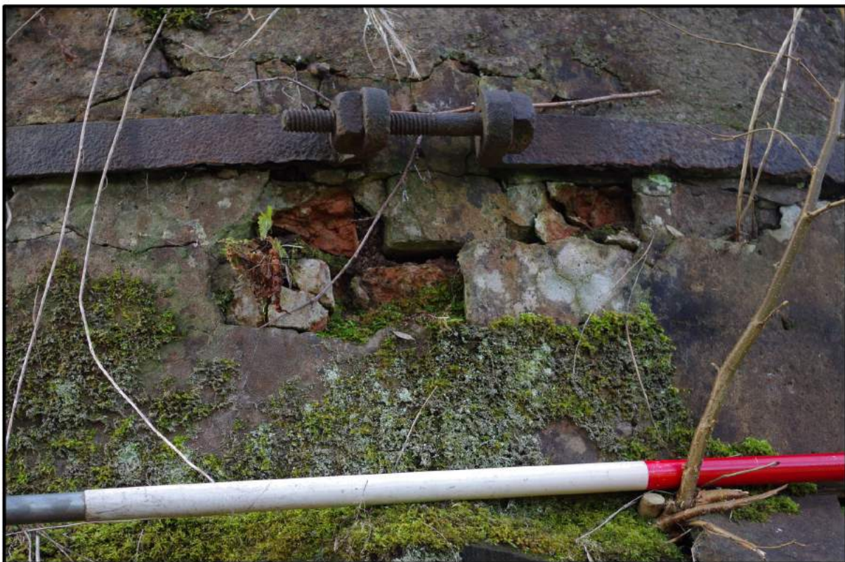
Fig 7: Detail of bolt securing one of the iron straps
