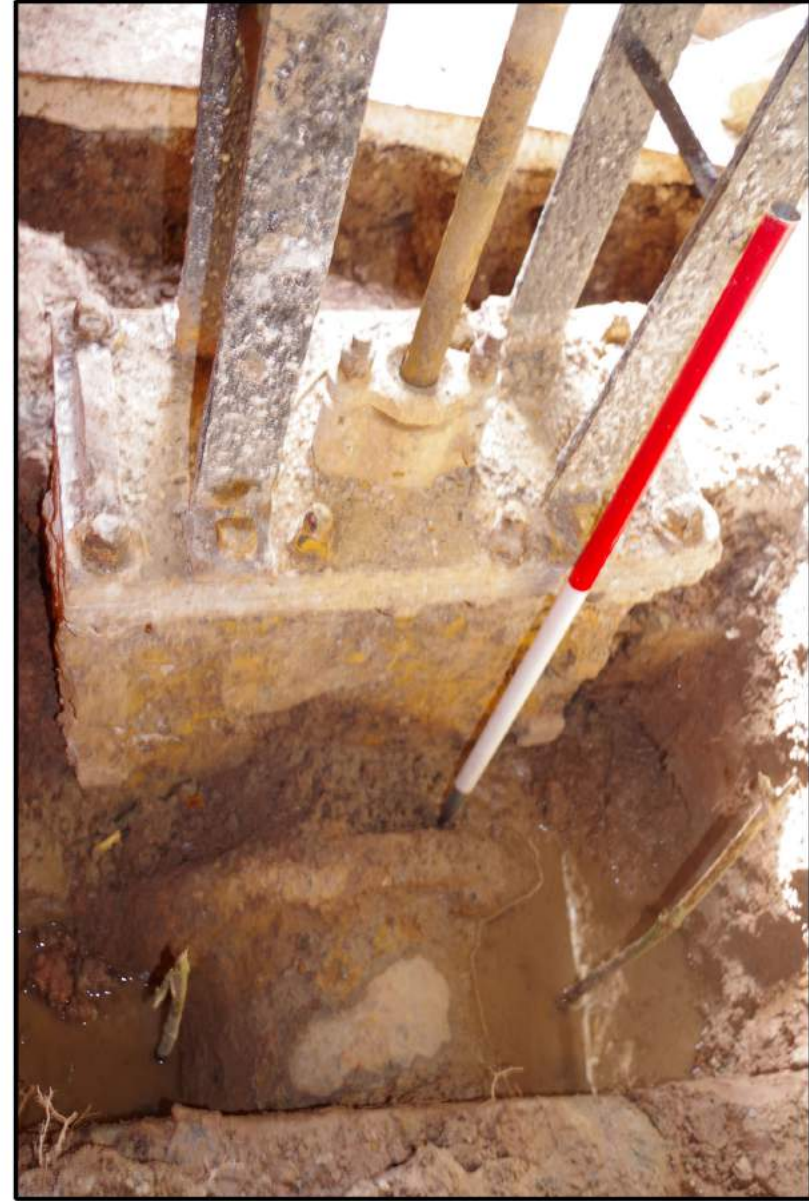
Fig 9: View of the valve base and pipe
