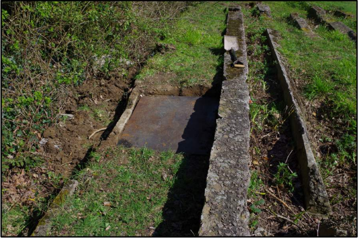
Fig 8: Access shaft covered by steel plate
