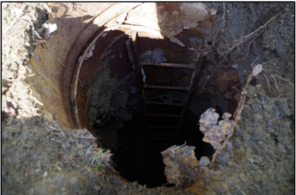
Fig 7: Interior of access shaft
