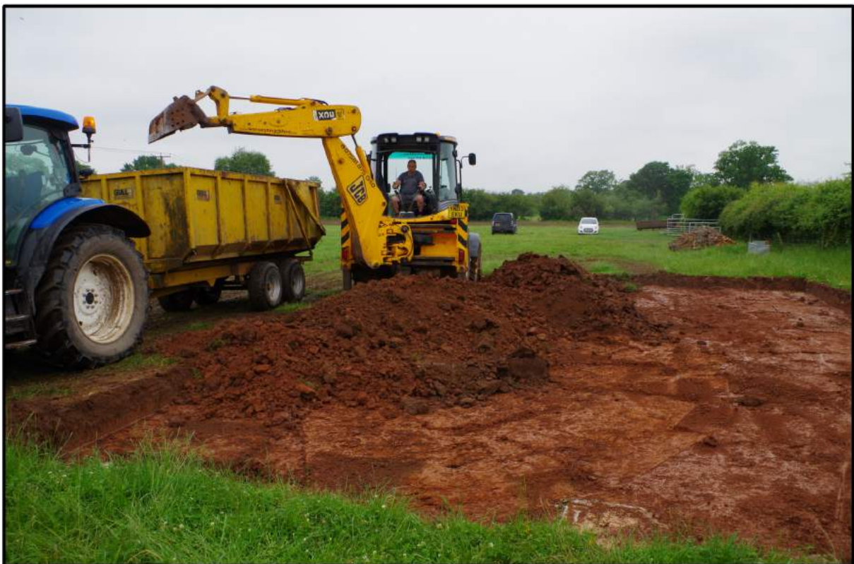
Fig 5: Stripping of footprint of building for floor slab
