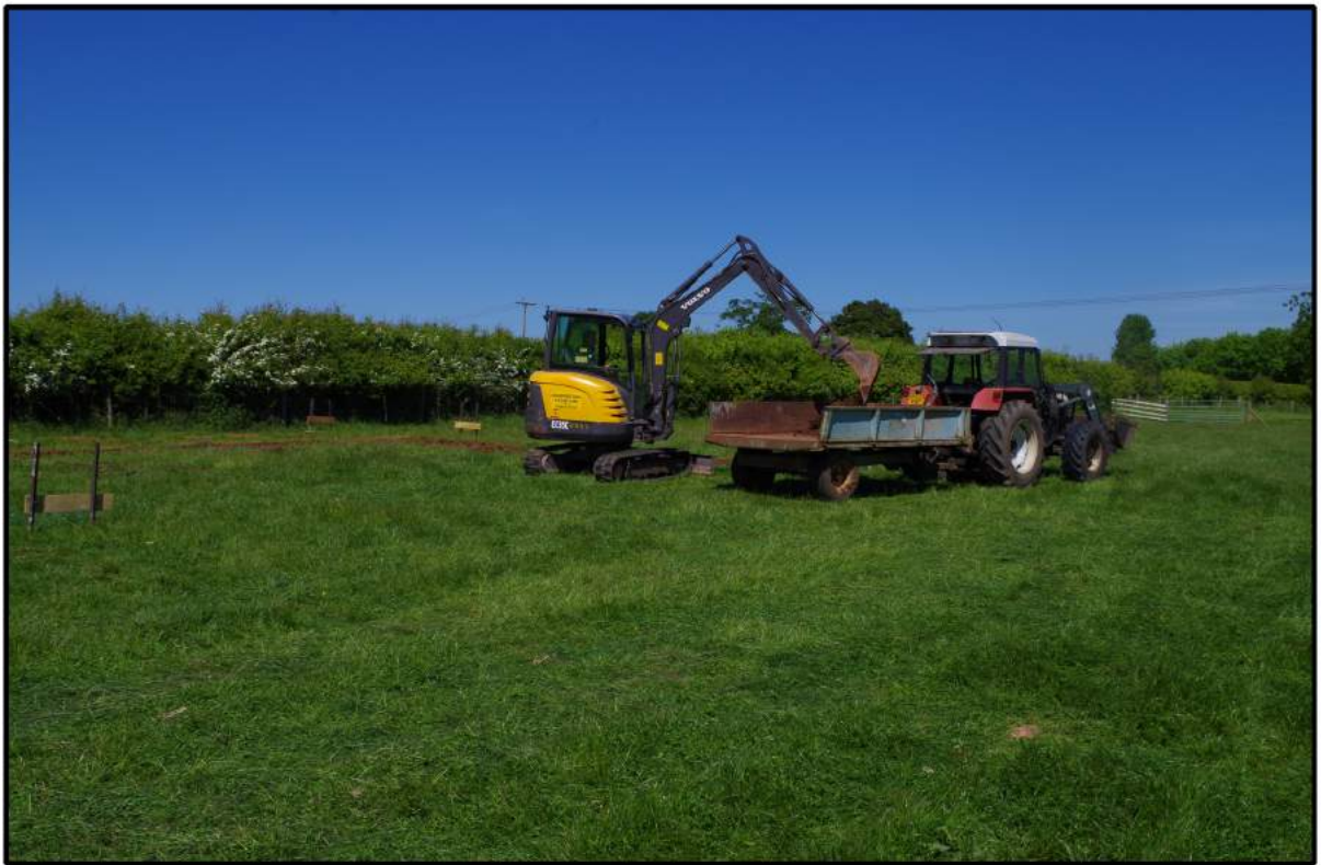
Fig 4: General view of site
