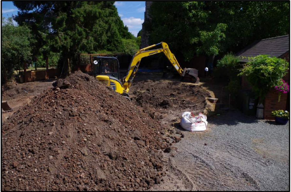
Fig 4: General view of area of ground reduction
