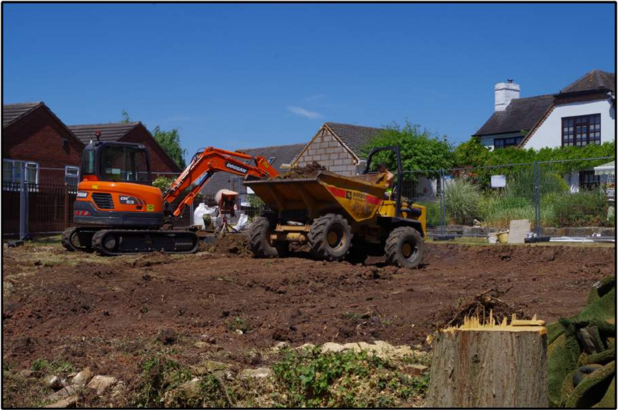
Fig 4: Stripping and ground reduction of area of house
