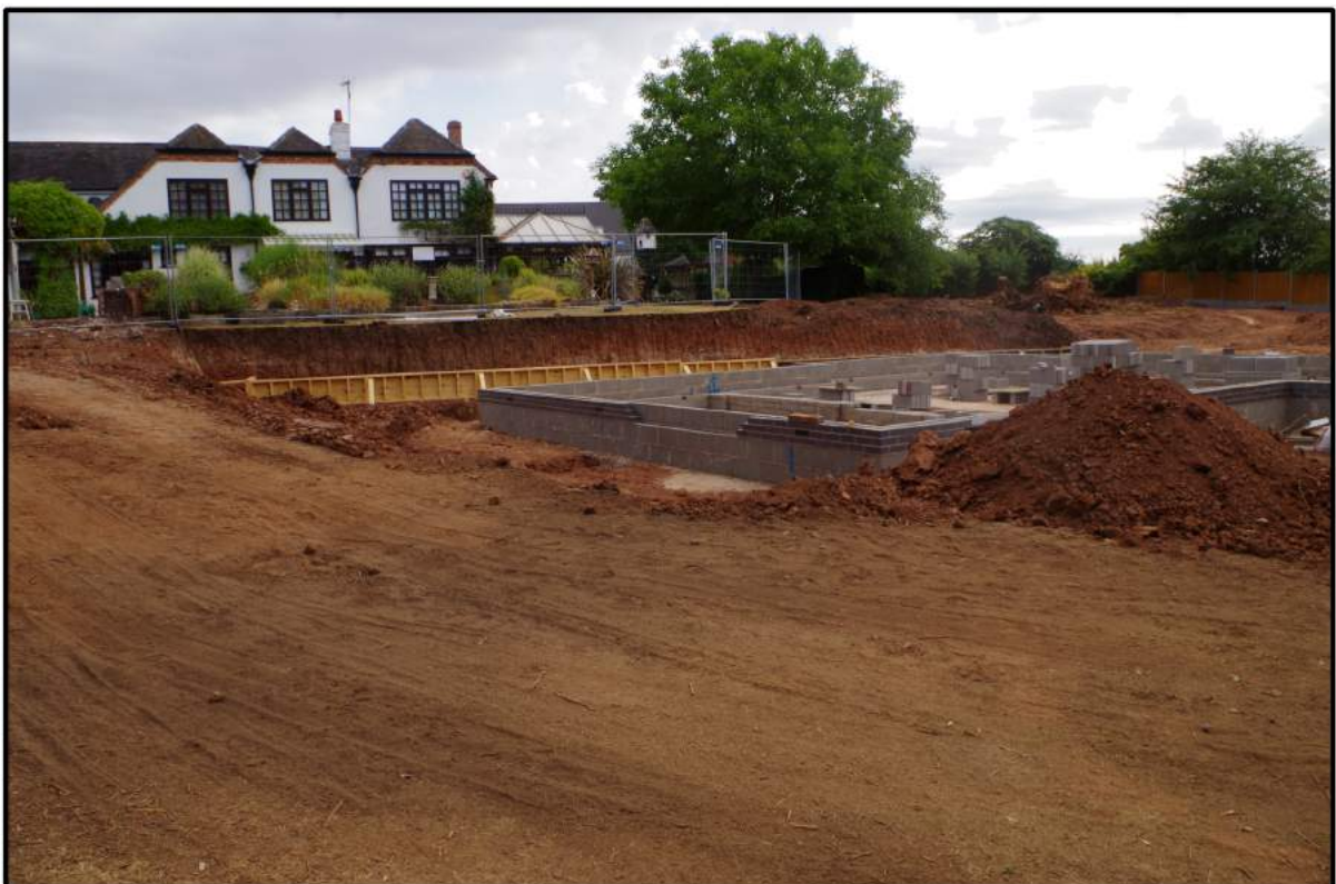
Fig 5: Full extent of ground reduction
