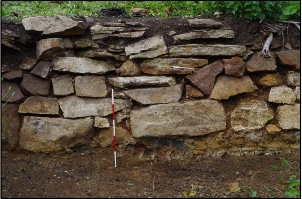
Fig 4: Example of canal side towpath walling at Hillmorton, Oxford Canal (Cook 2017)
