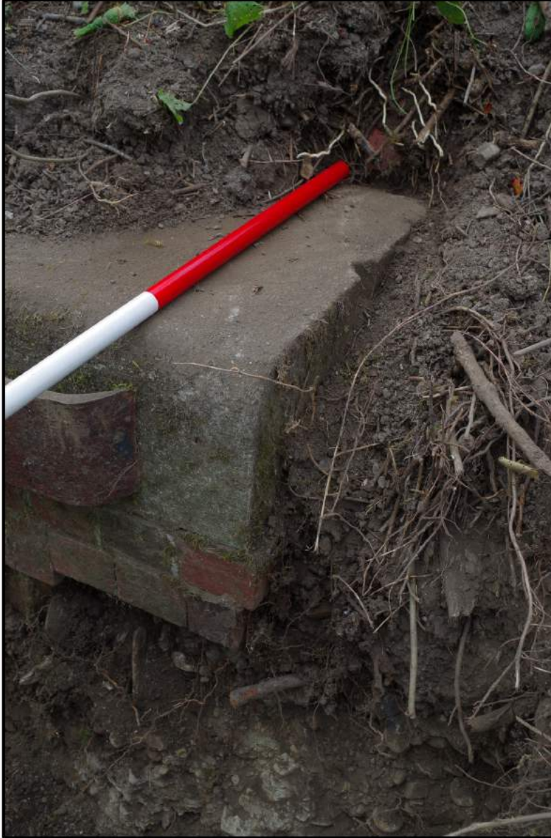
Fig 3.4: Detail of the Bridge 85 offside forebay wall; coping
