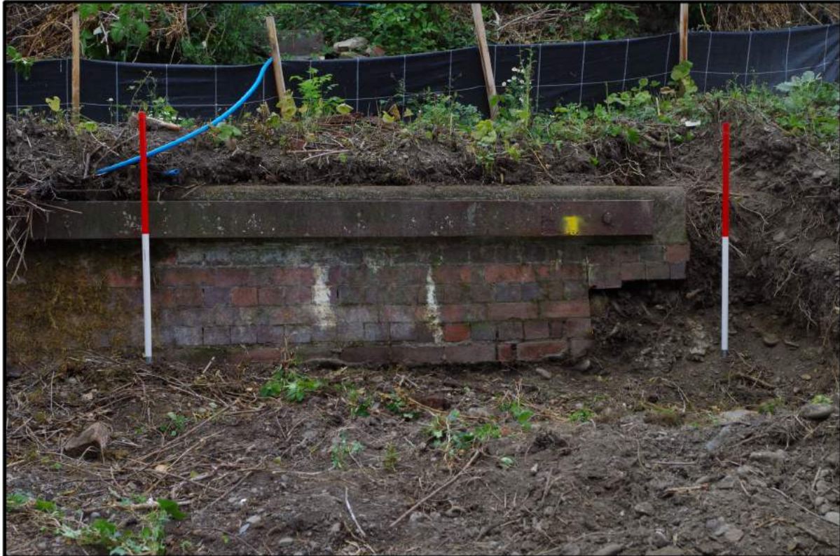
Fig 3.3: View of the offside Bridge 85 forebay wall
