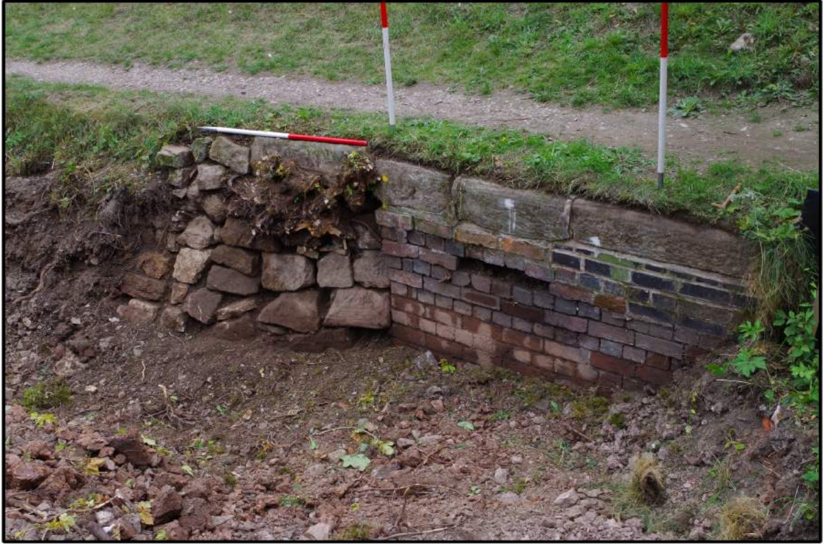
Fig 3.2: View of the nearside towpath retaining wall and Bridge 85 forebay wall
