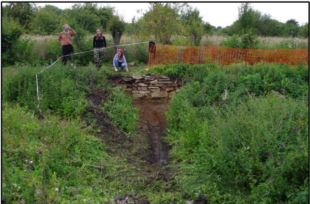
Fig 7: Area of rubble stone towpath walling, Grand Union Canal, Hillmorton
