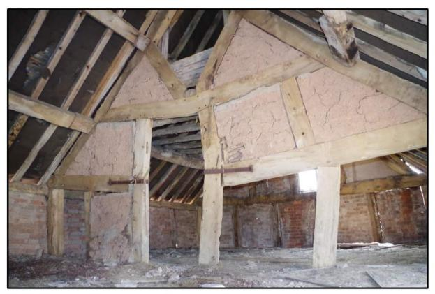
Fig 16: Phase 1 hay loft showing closed truss with wattle and daub panels
