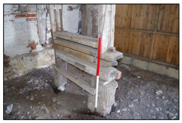
Fig 19: Phase 4 oast house; ground floor showing lower part of hop press
