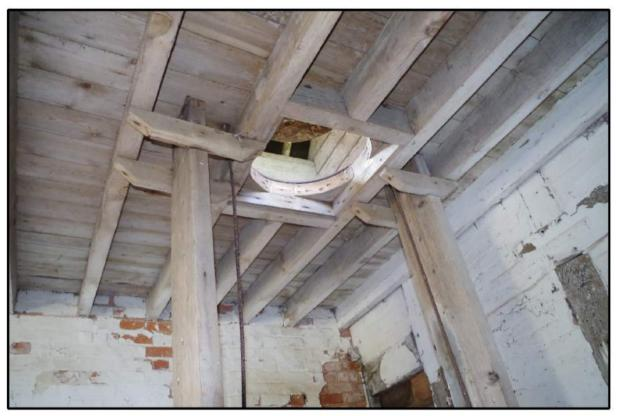
Fig 21: Phase 4 oast house; ground floor showing arrangement of hop pocket hole
