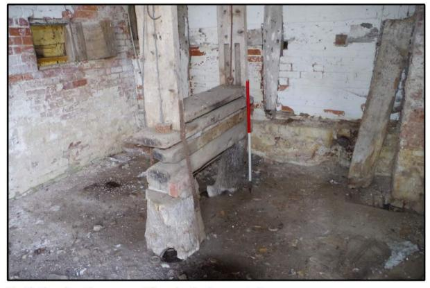
Fig 20: Phase 4 oast house; ground floor showing lower part of hop press
