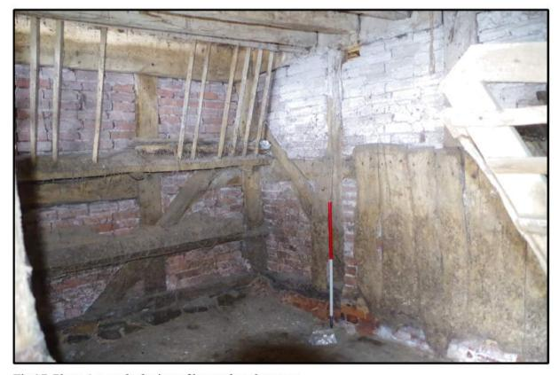
Fig 27: Phase 1 cow shed; view of hay rack and manger
