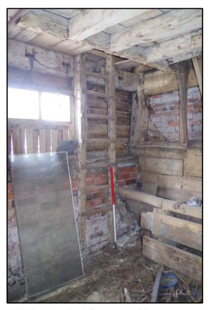
Fig 28: Phase 1 cow shed; ladder access to hayloft
