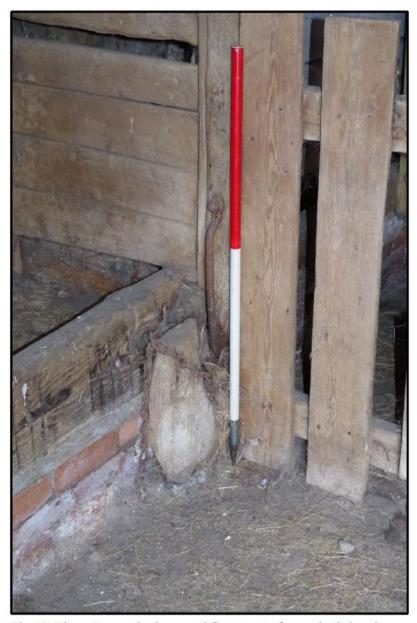
Fig 23: Phase 1 cow shed; ground floor, part of cow shed showing restraining bar and chain
