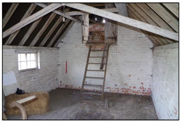
Fig 14: Phase 4 oast house; first floor, hop sorting and bagging floor; showing stair to hop drying floor
