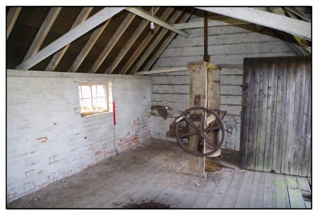
Fig 9: Phase 4 Oast house; first floor, hop sorting and bagging floor; showing upper part of hop press
