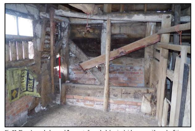
Fig 22: Phase 1 cow shed; ground floor, part of cow shed showing brick manger with wooden fittings
