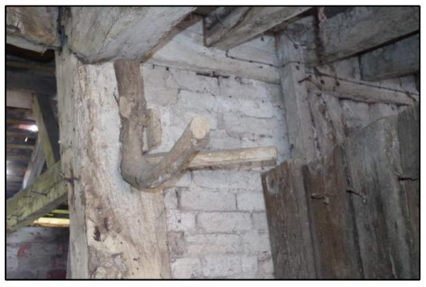
Fig 29: Harness hook improvised from forked branch
