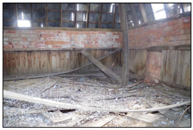
Fig 8: Phase 4 Oast house; first floor, hop drying floor; showing wooden panelling around lower part of walls
