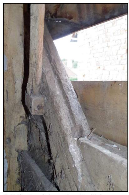
Fig 34: Phase 1 cow shed; grooves for wattle and daub
