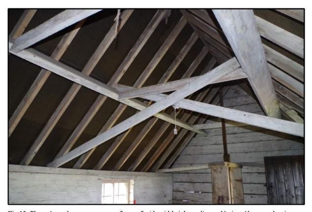
Fig 13: Phase 4 oast house; common rafter roof with mid-height purlins and 'scissor' braces, clasping a 'collar' brace between them
