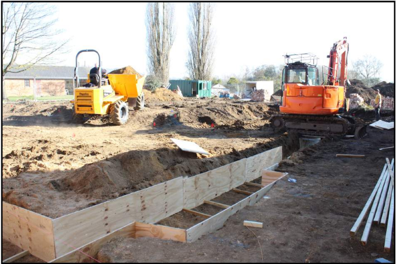
Fig 6: View of site from north-west showing shuttering to trenches
