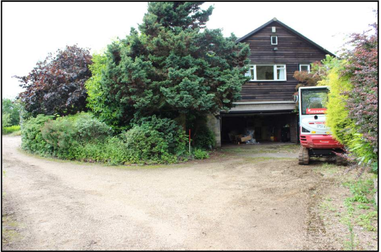
Fig 6: View of existing building looking south, showing excavation for subterranean garage
