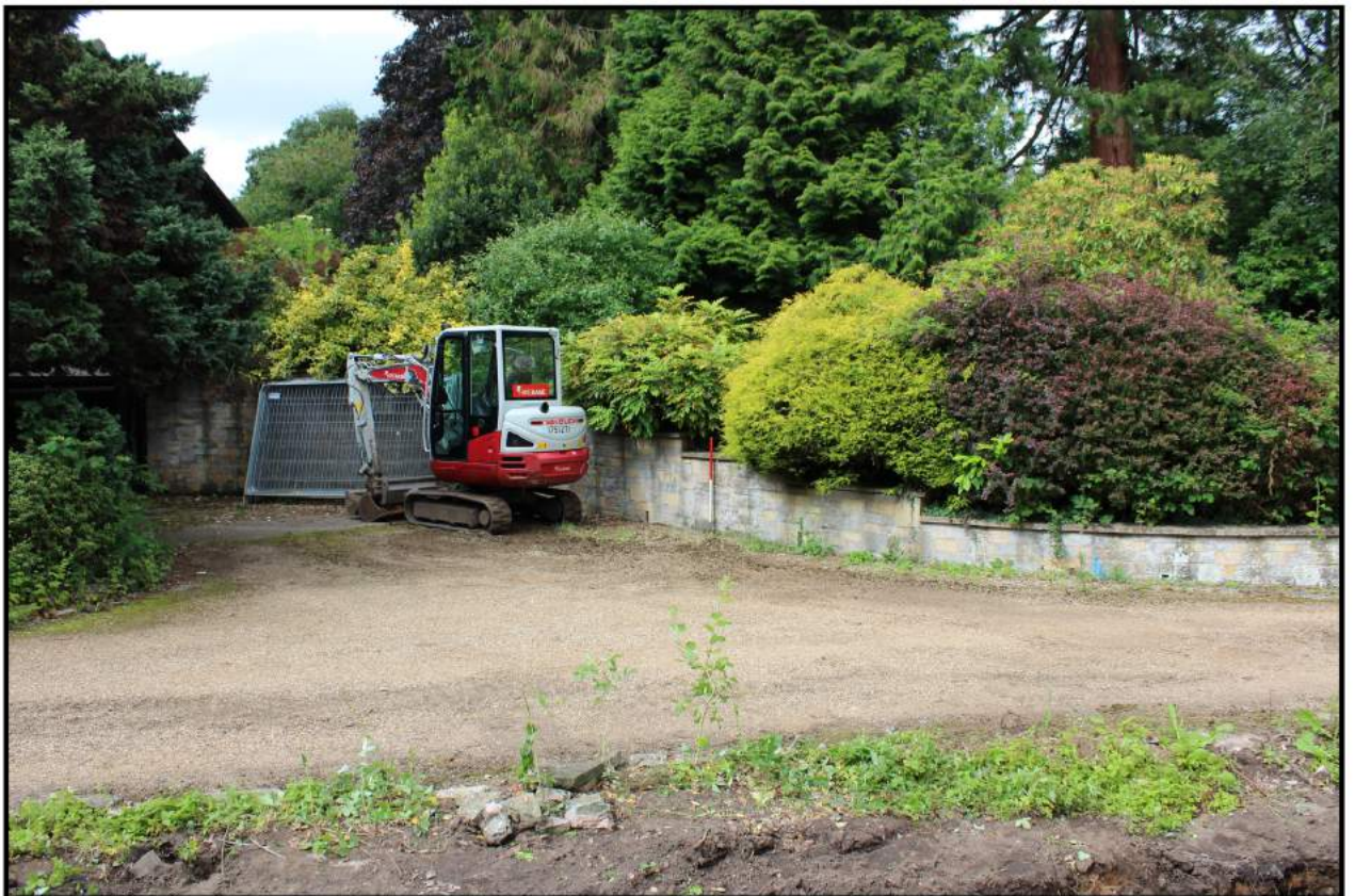
Fig 7: View of existing building looking west, showing excavation for subterranean garage
