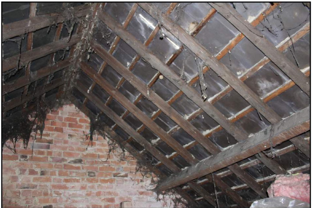
Fig 37: Roof space showing common rafter roof
