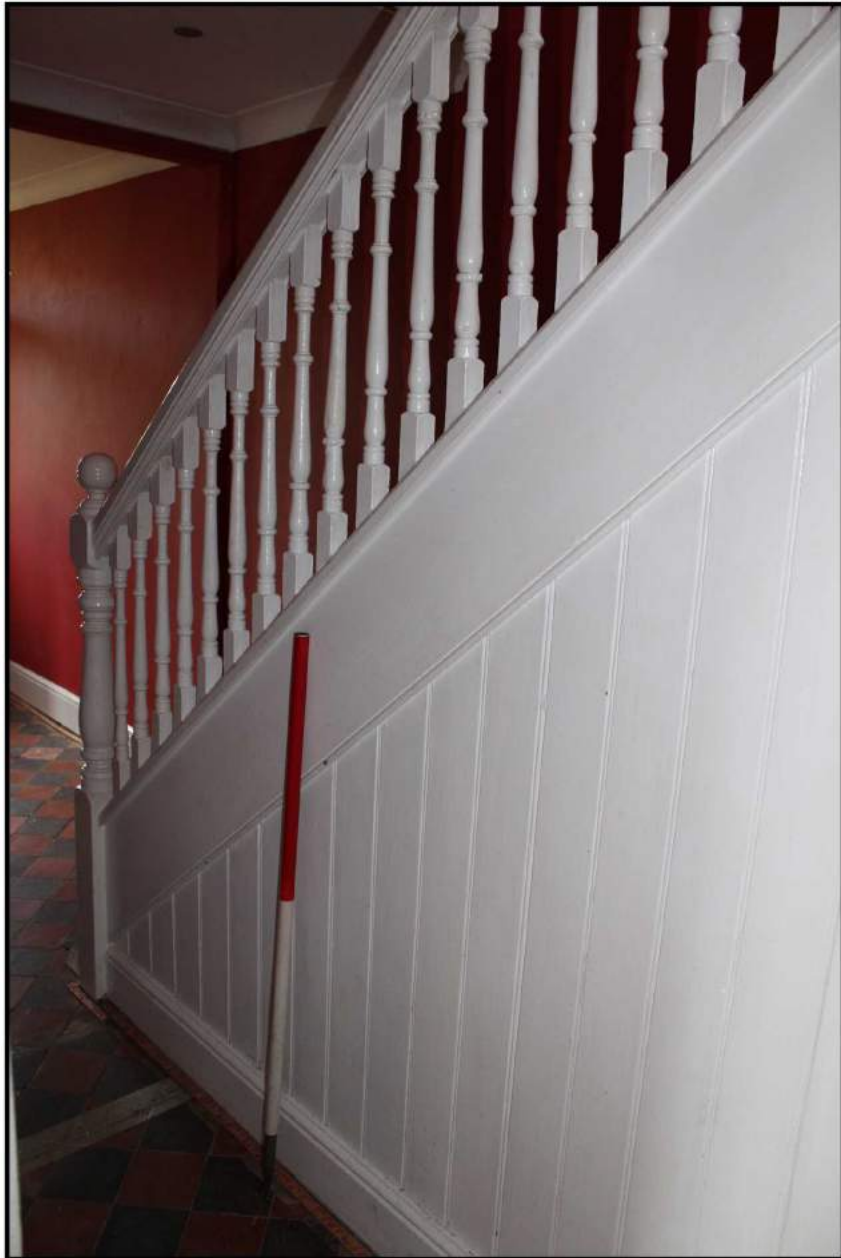
Fig 24: Room 1; detail of staircase
