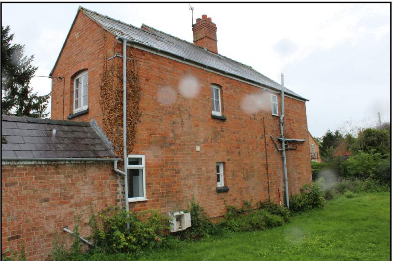
Fig 12: West elevation; south end
