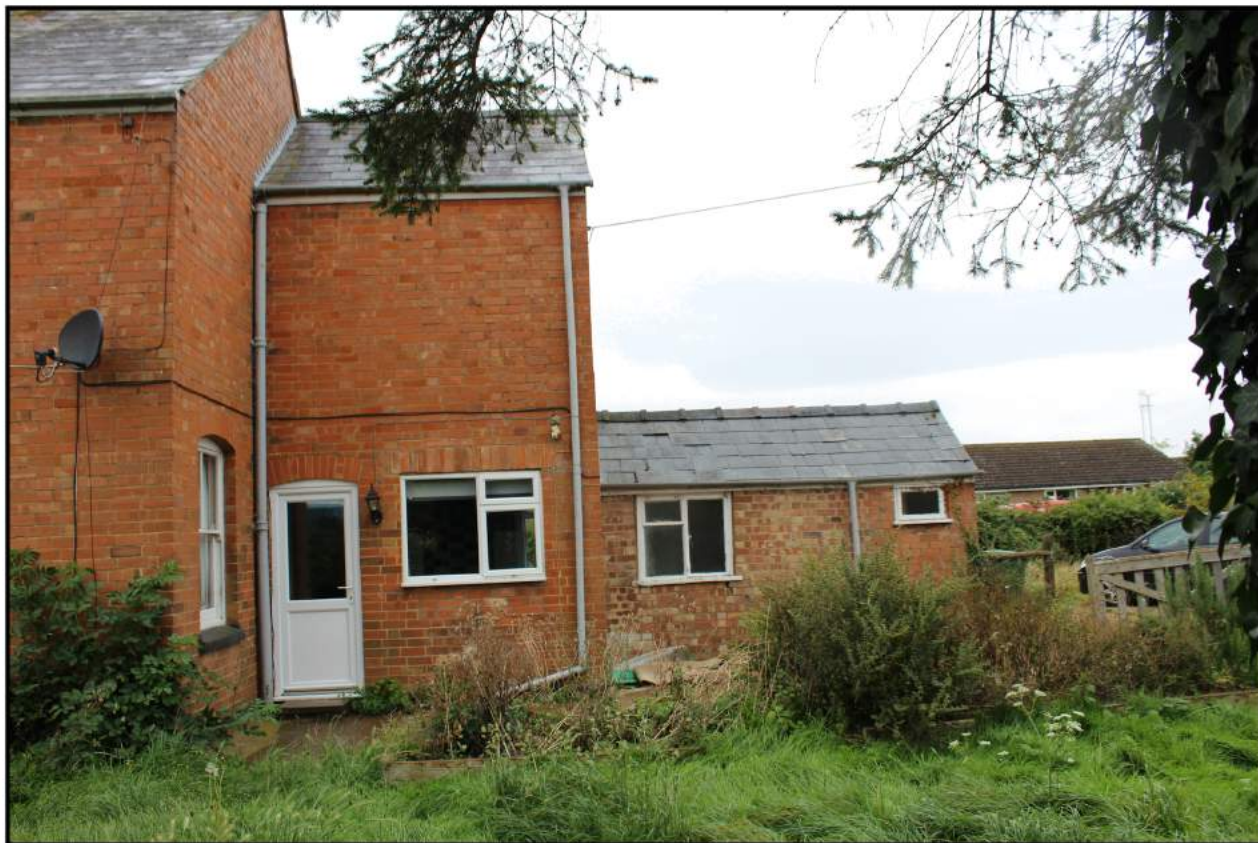
Fig 8: East elevation; north end
