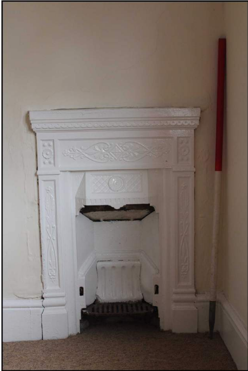
Fig 28: Room 12; third bedroom; detail of fireplace
