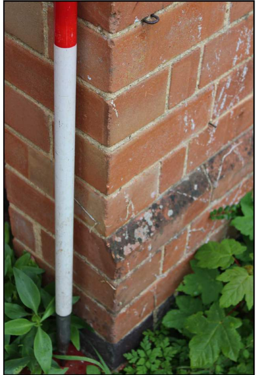
Fig 5: South elevation; detail of battered brick course
