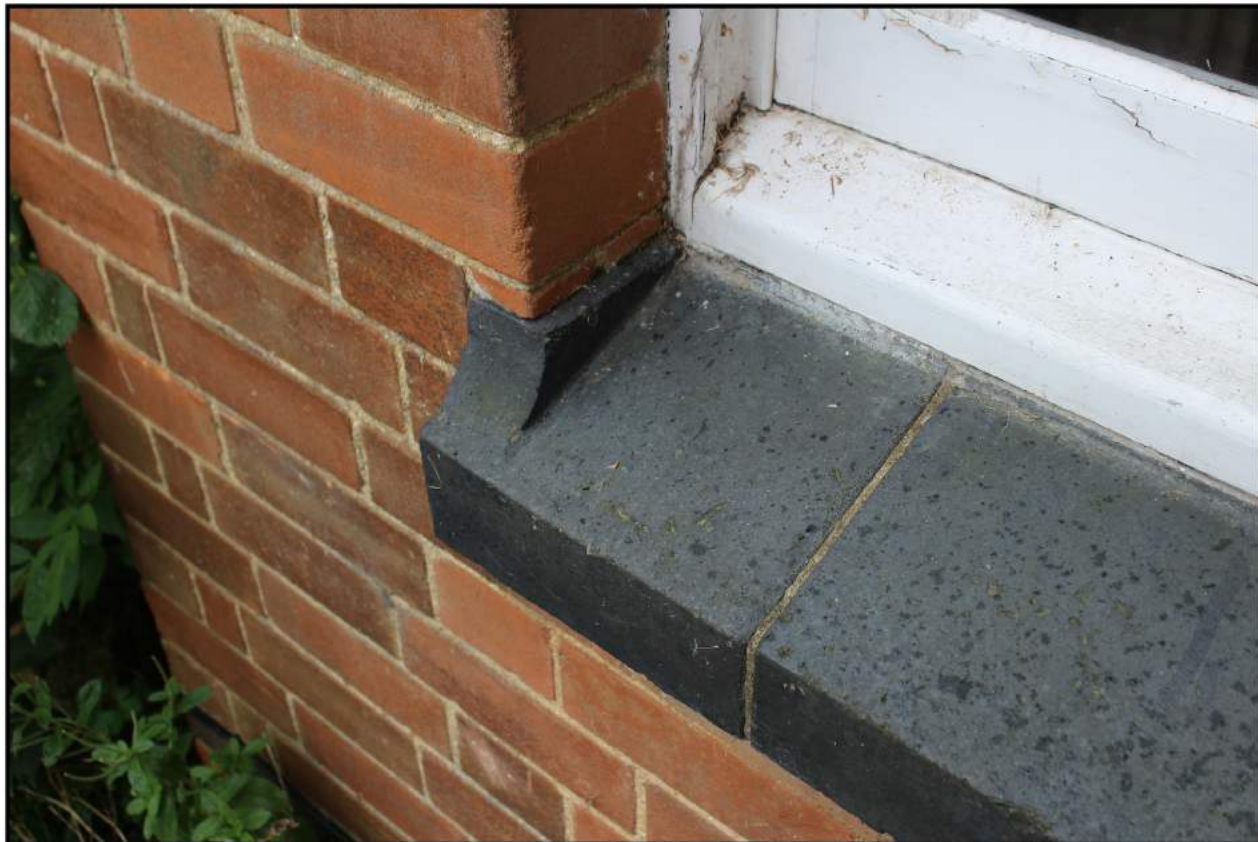
Fig 9: North elevation; detail of mounded blue brick cill
