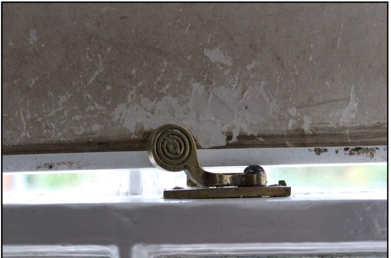
Fig 21: Room 3; dining room, detail of window catch
