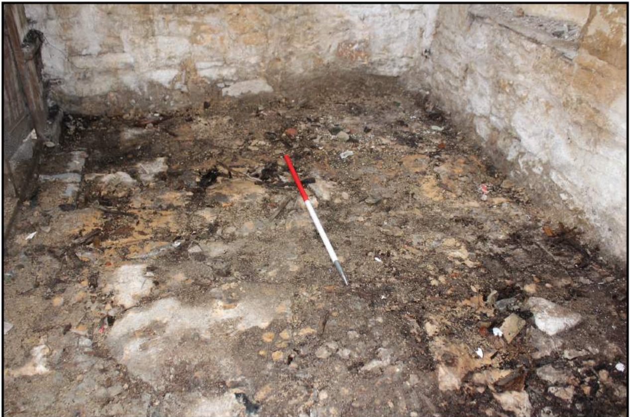
Fig 14: Interior, south-west end; showing stone floor
