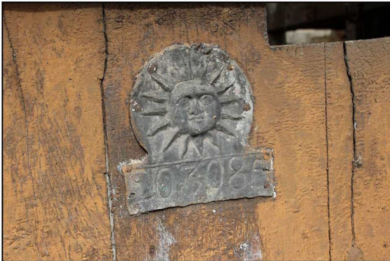
Fig 10: South-east elevation; showing Sun Fire Office plaque
