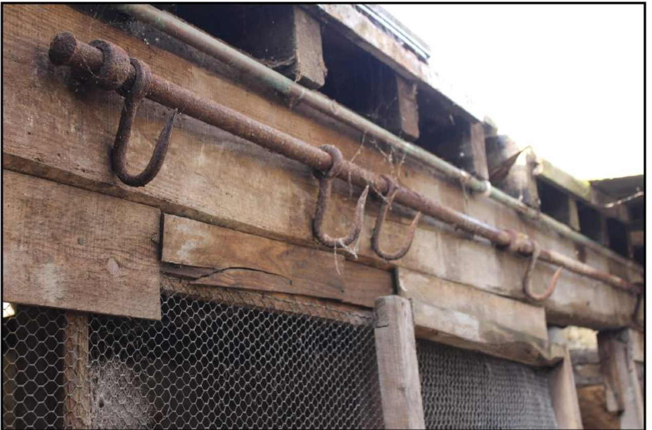
Fig 18: Interior, cross-passage; showing row of butcher's hooks
