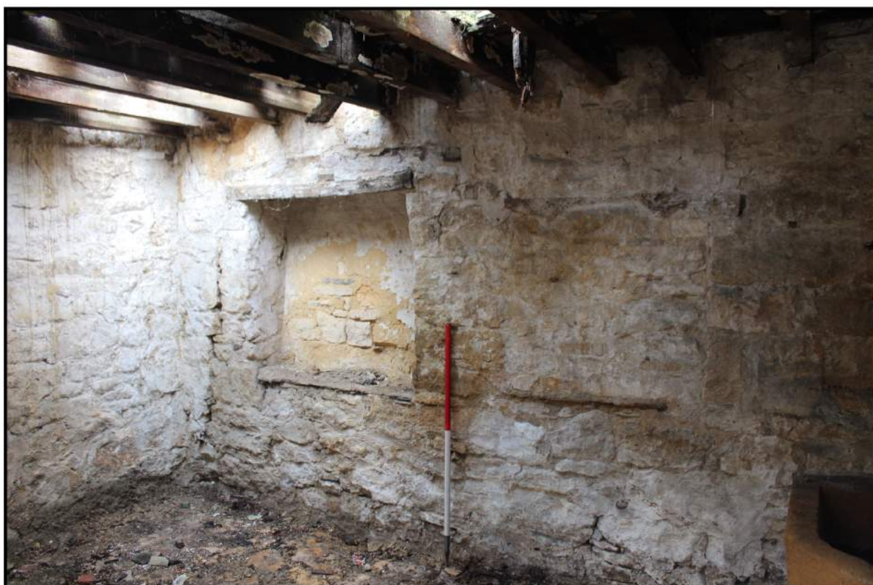
Fig 11: Interior, south-west end; showing two blocked windows
