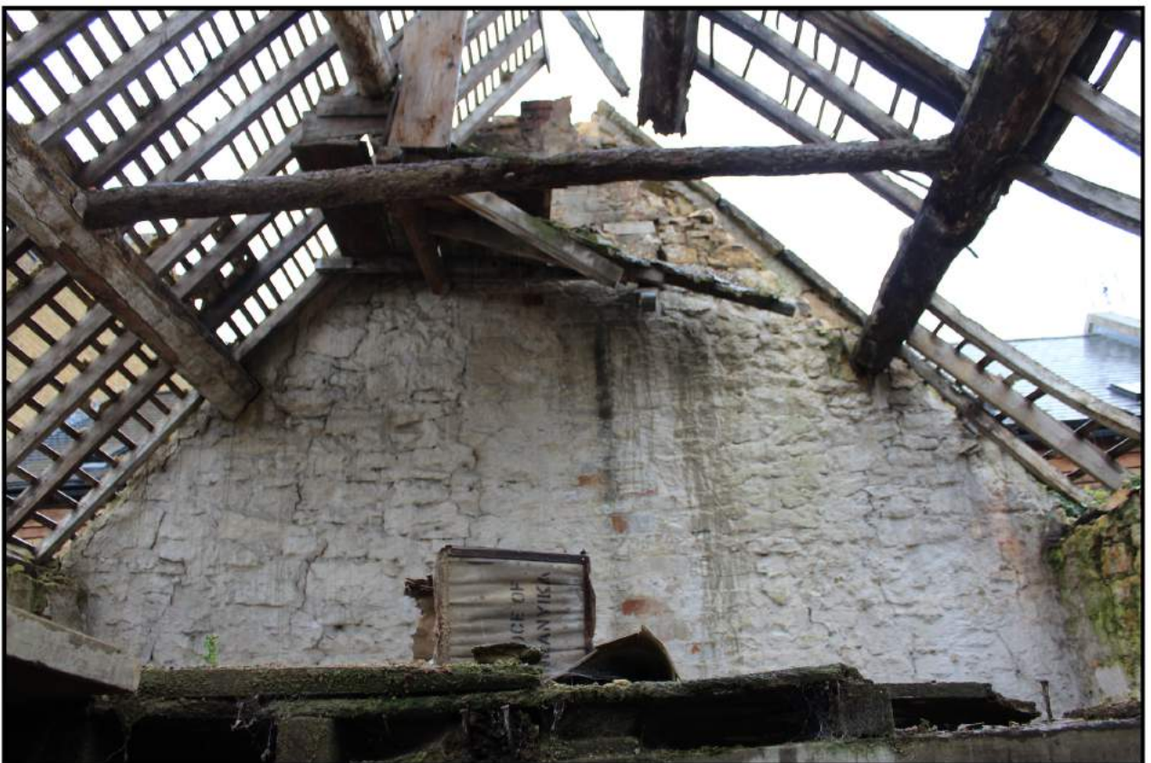
Fig 22: First floor, north-east gable wall
