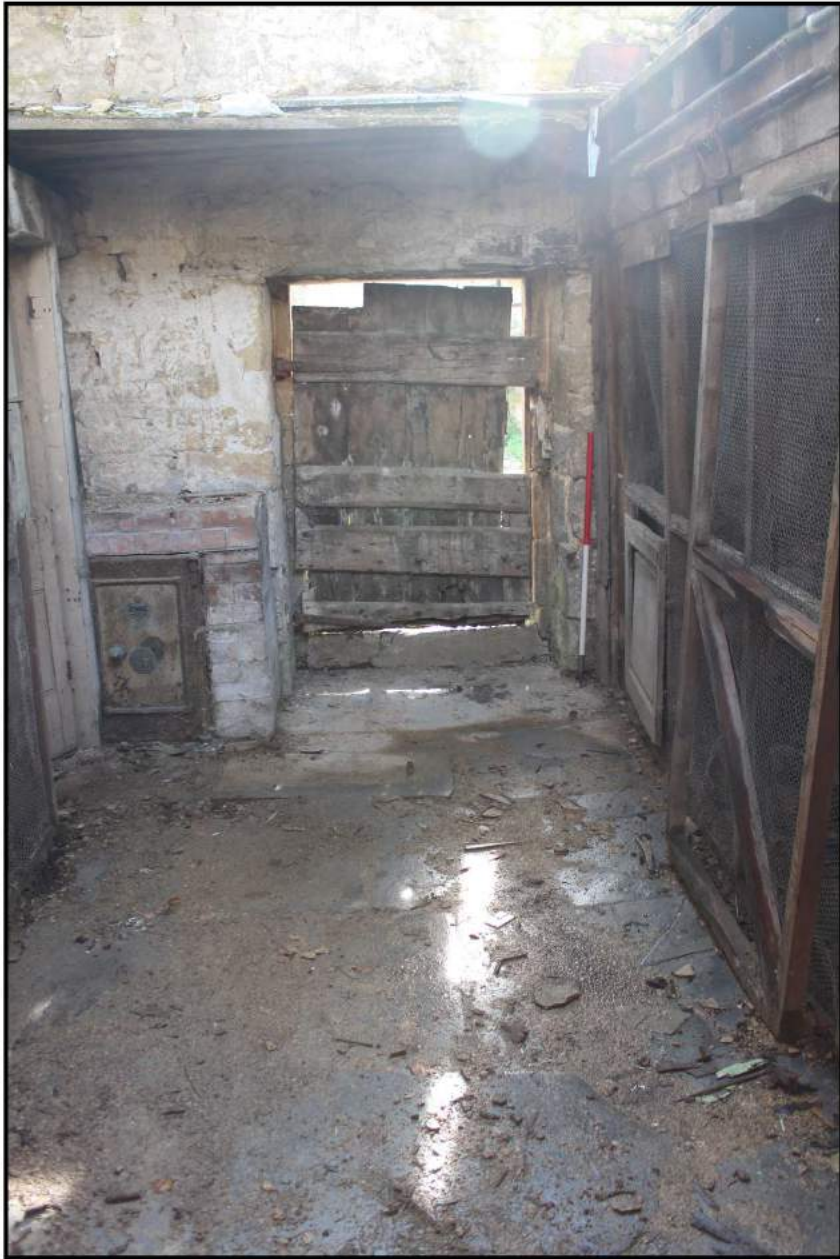
Fig 15: Interior; showing cross-passage, south end
