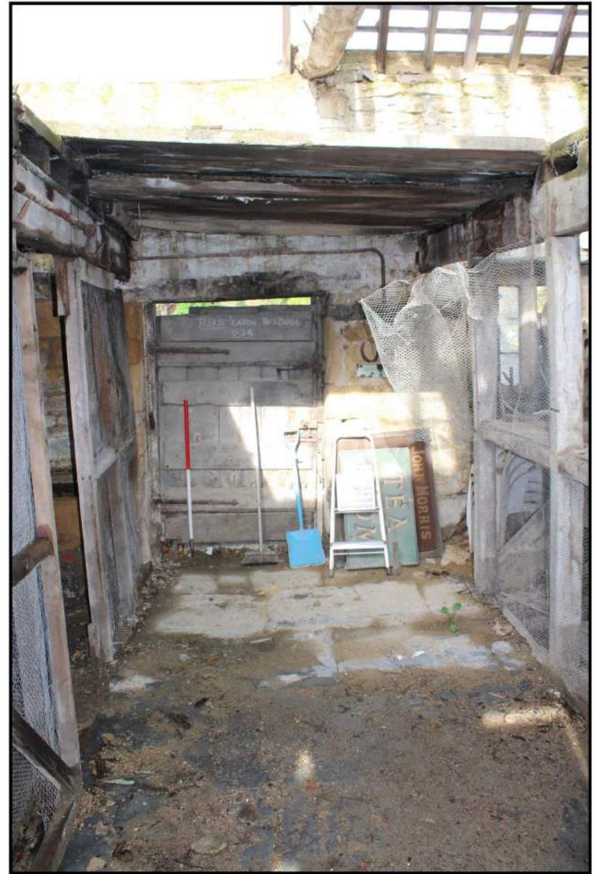
Fig 16: Interior; showing cross-passage, north end
