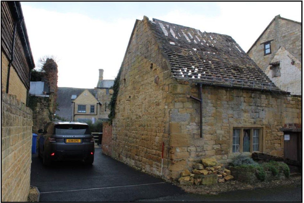
Fig 4: North-east and north-west elevations
