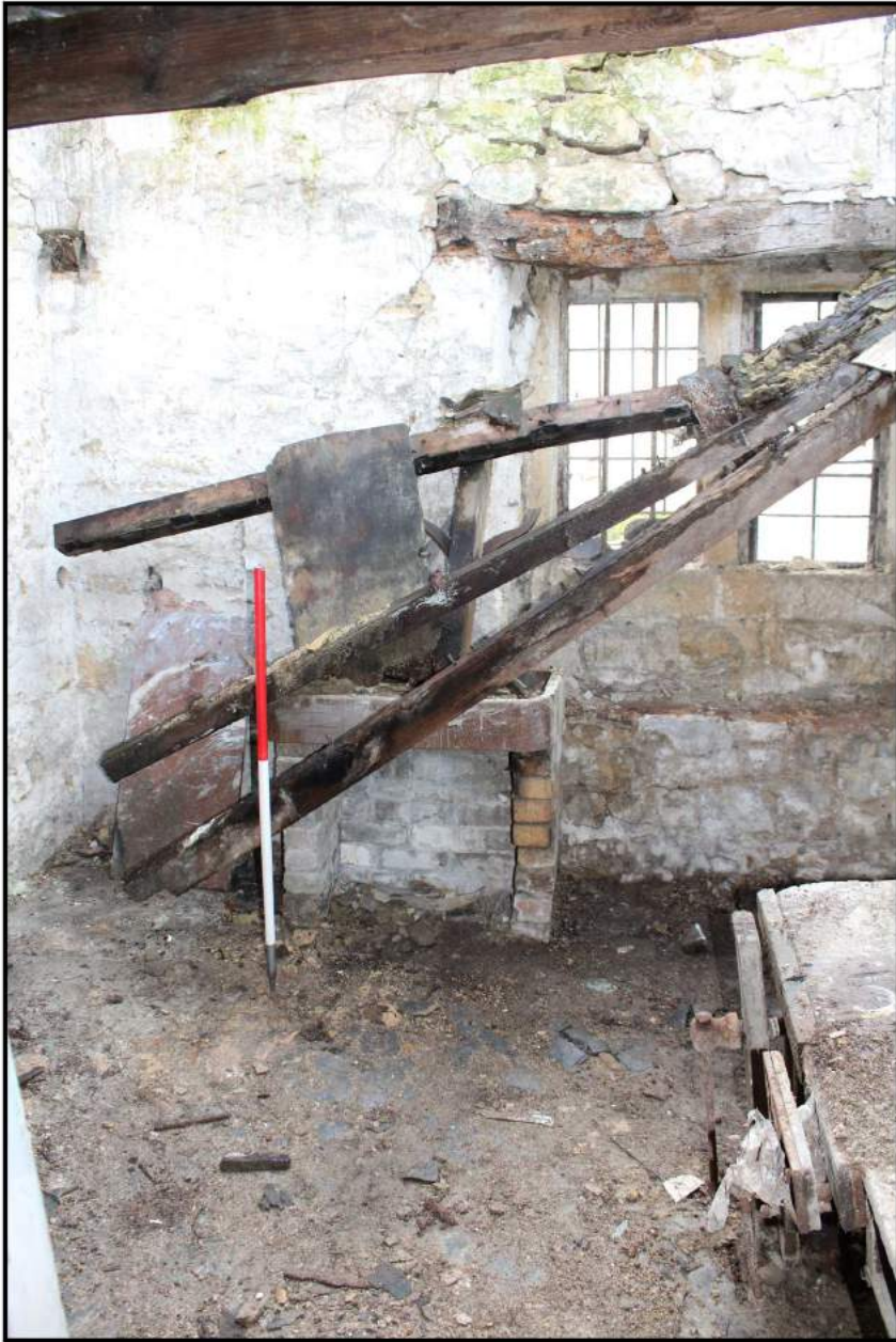
Fig 19: Interior, north-east end; showing sink
