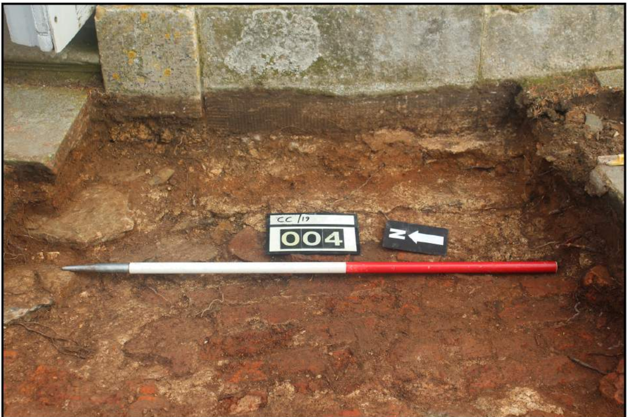
Fig 5: Triangular fillet of mortar (context 004) between the stone skin of the Rotunda (context 009) and the stepped foundation (context 008)
