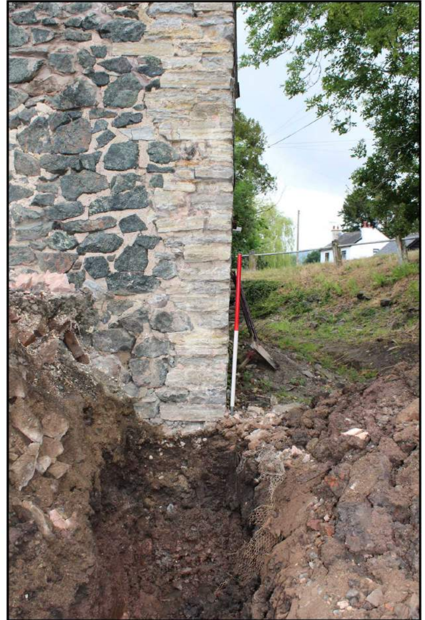
Fig 9: Northern footing trench and part of ditch adjacent to road
