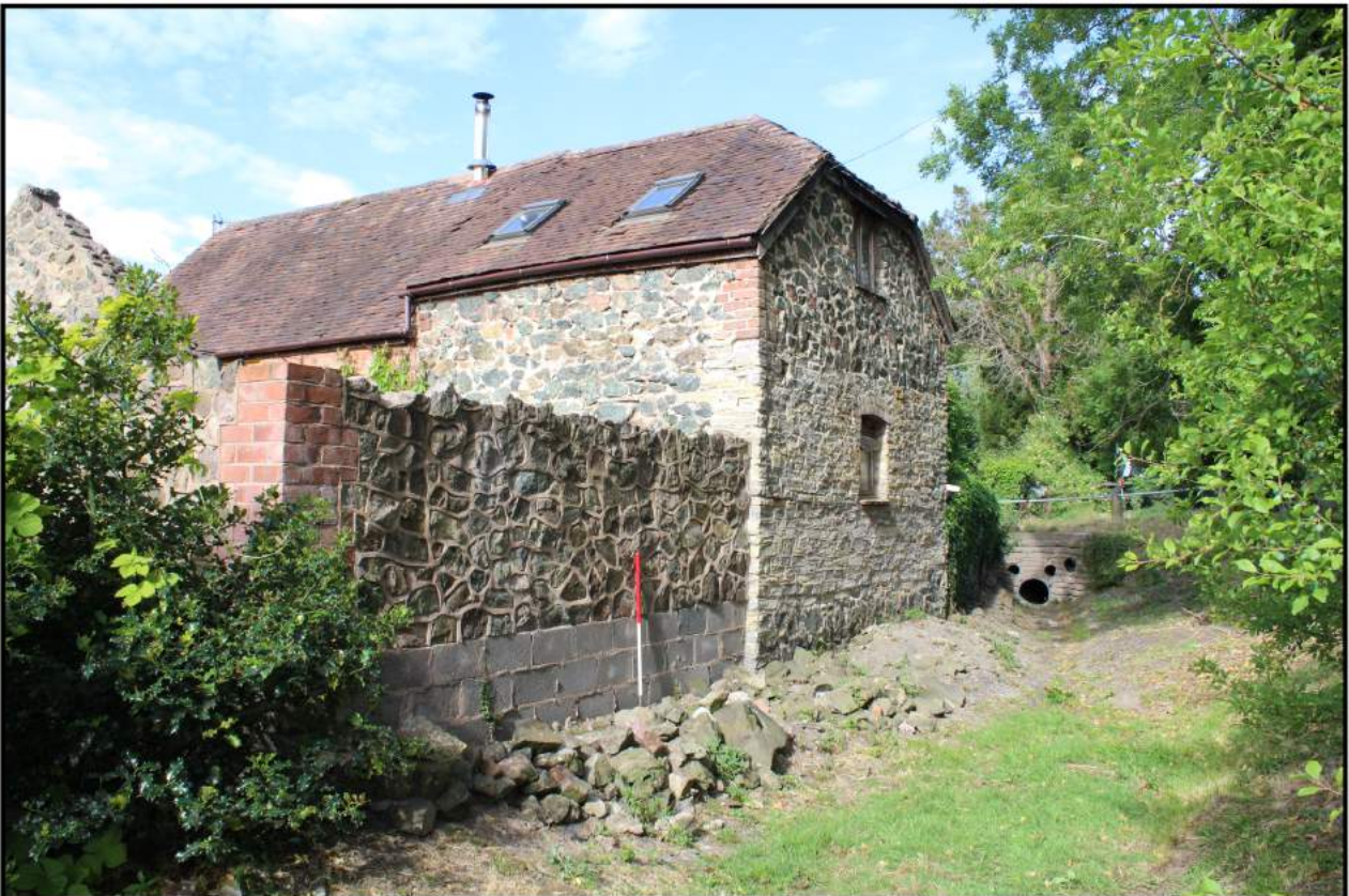
Fig 7: North elevation showing later block wall faced with random stone
