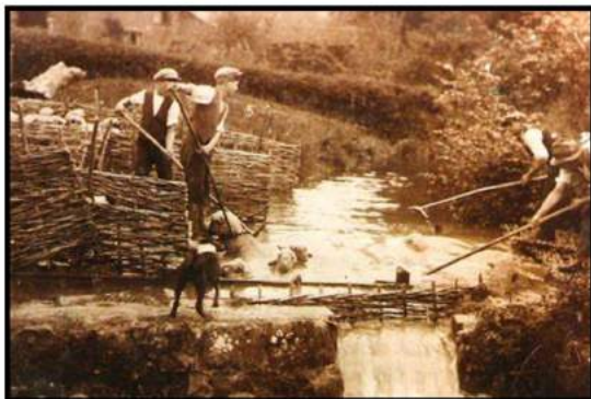
Fontmell Magma, south of Shaftesbury - sheepwash
