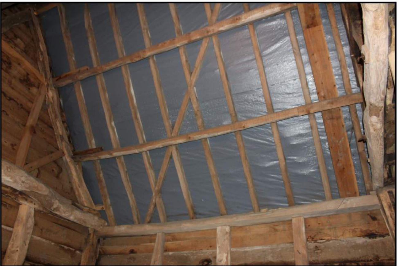
Fig 21: East corner of barn showing modern roof structure
