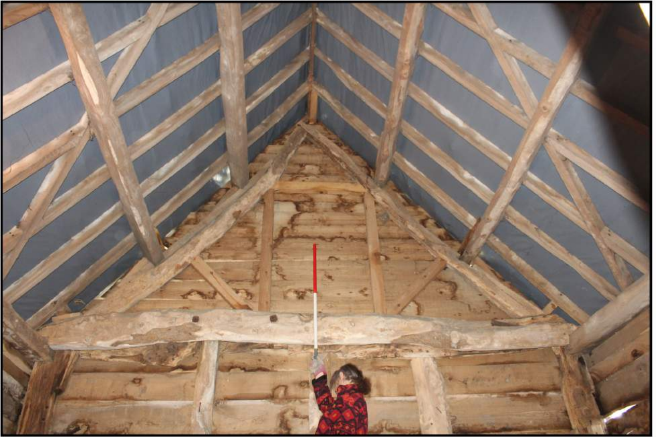
Fig 20: Upper part of truss 1
