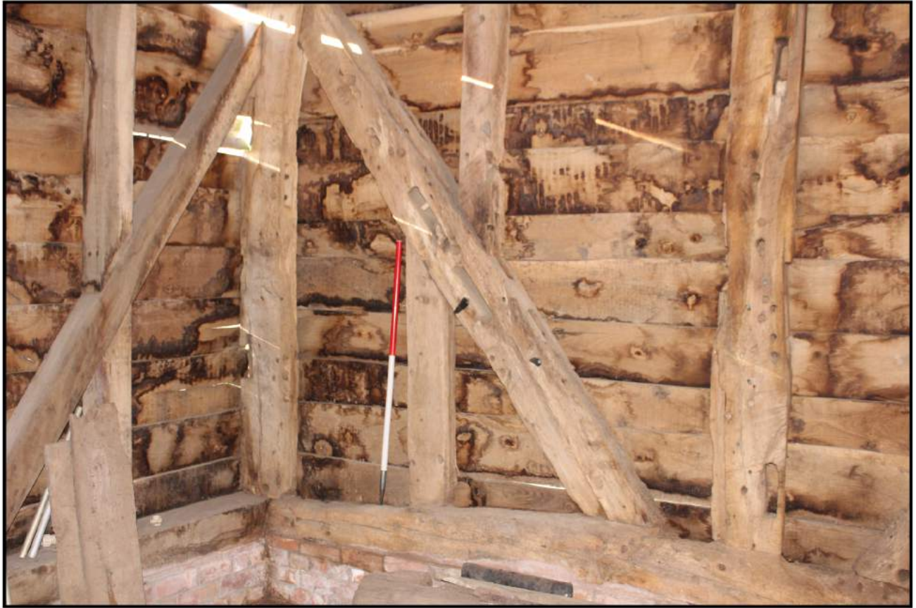
Fig 14: Detail of south corner of barn
