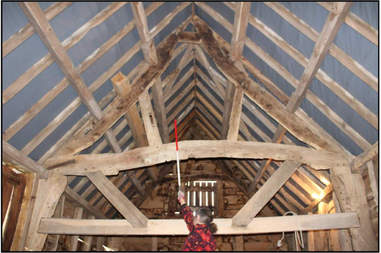
Fig 18: Upper part of truss 3
