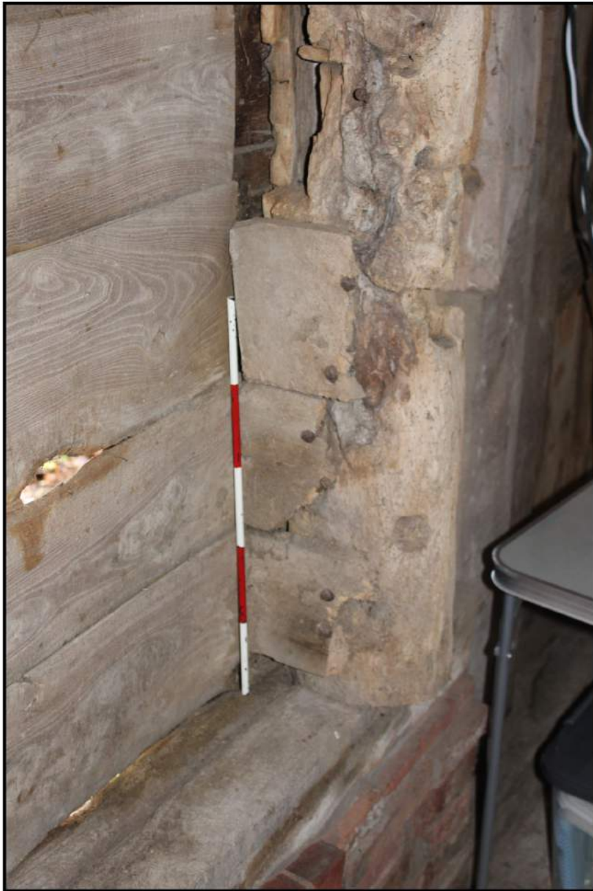
Fig 22: Barn interior; north-west elevation, south-west end, detail of possible cornhole
