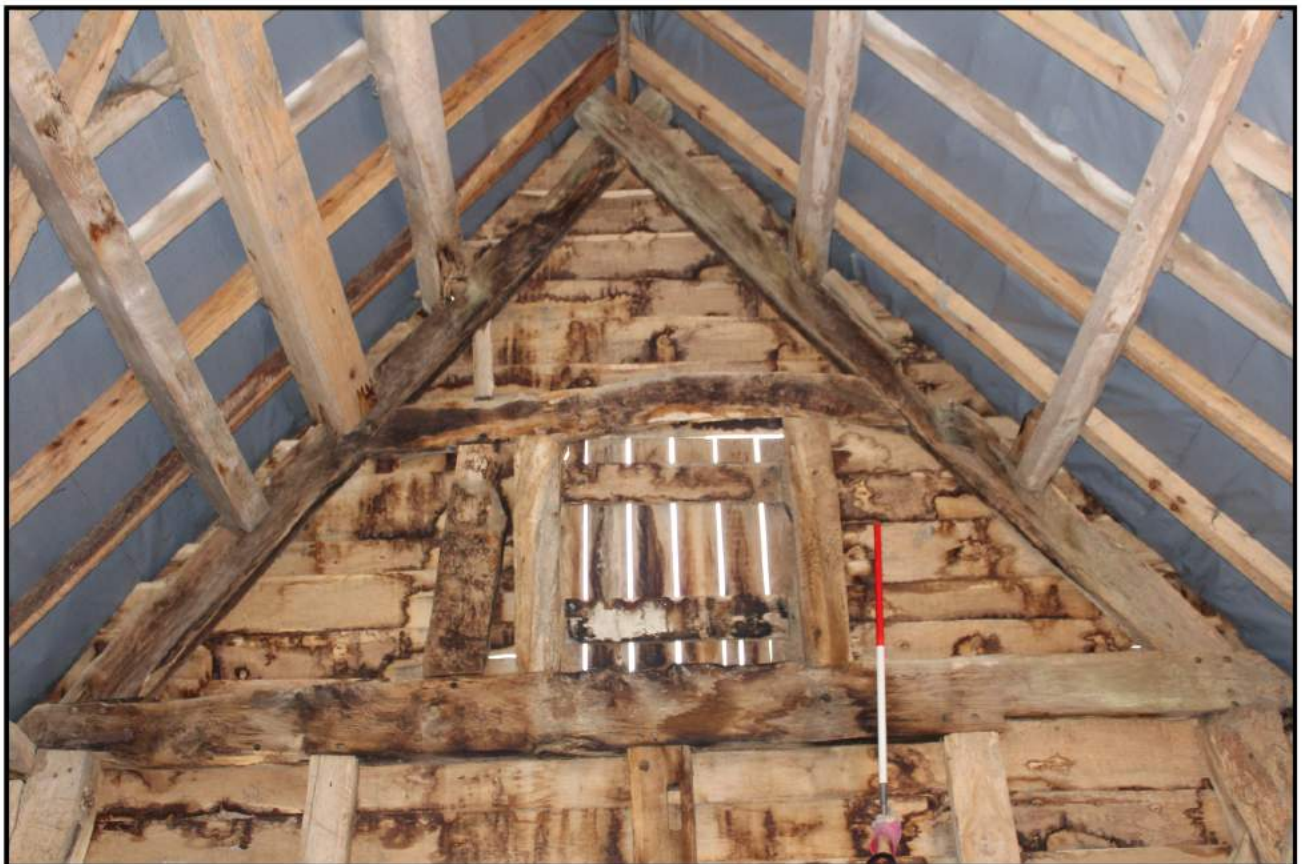
Fig 17: Upper part of truss 4
