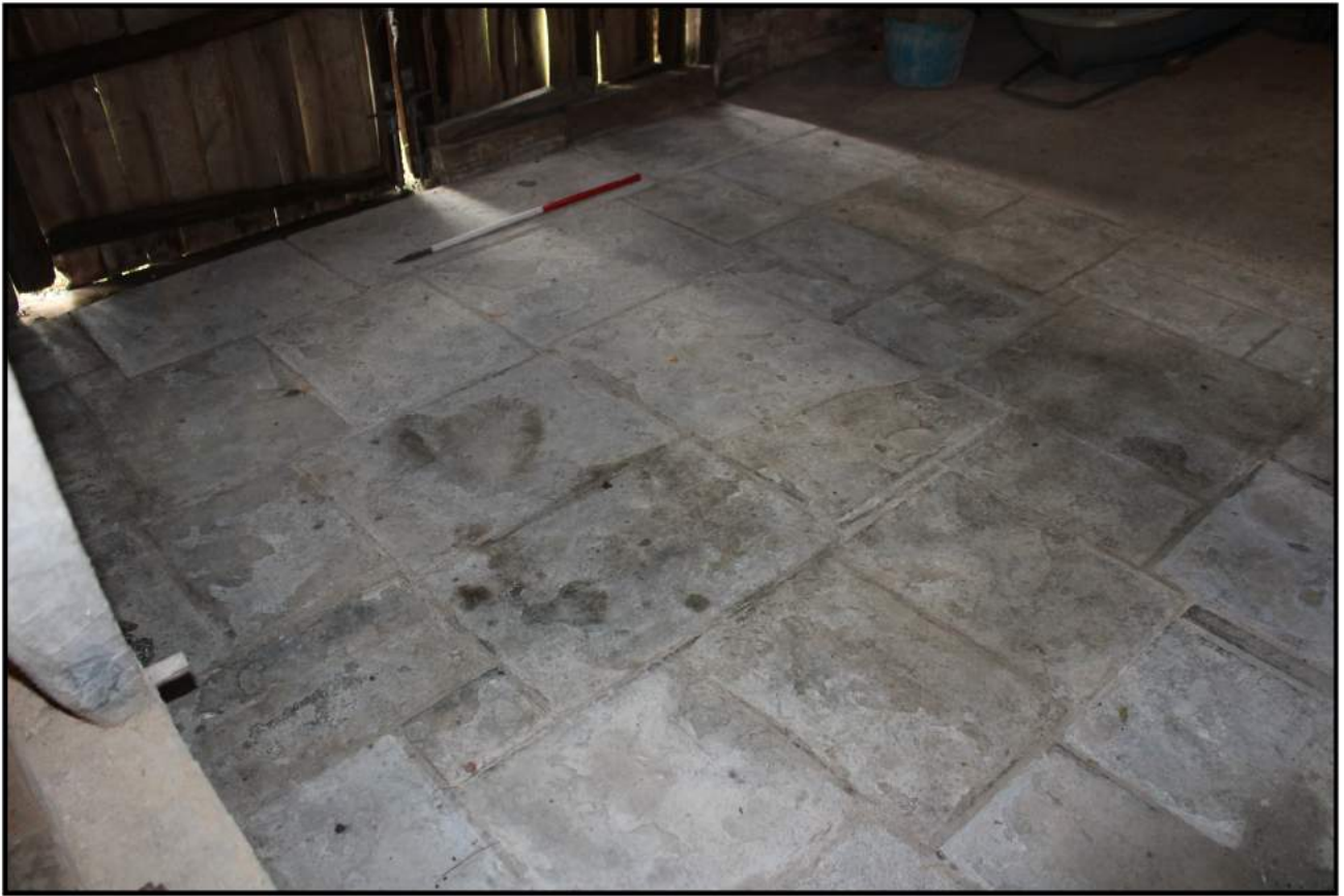
Fig 29: The threshing floor; relaid when the concrete floors were installed
