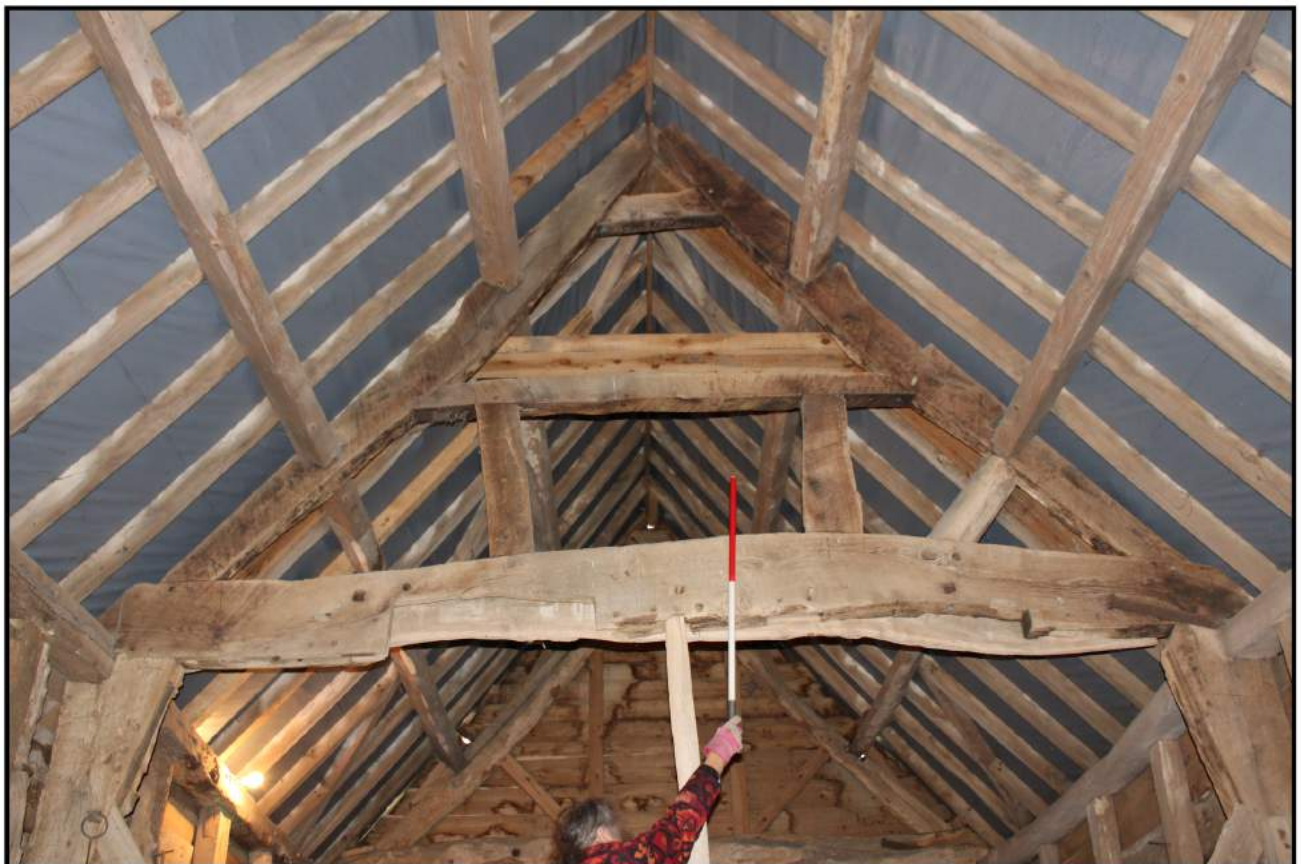
Fig 19: Upper part of truss 2
