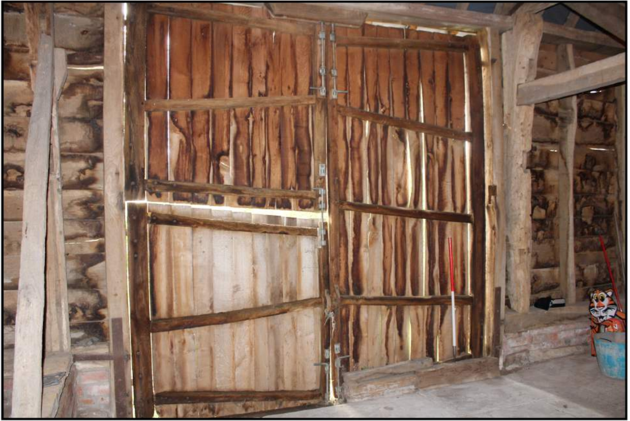
Fig 27: Barn interior; south-east elevation, detail of threshing floor doors
