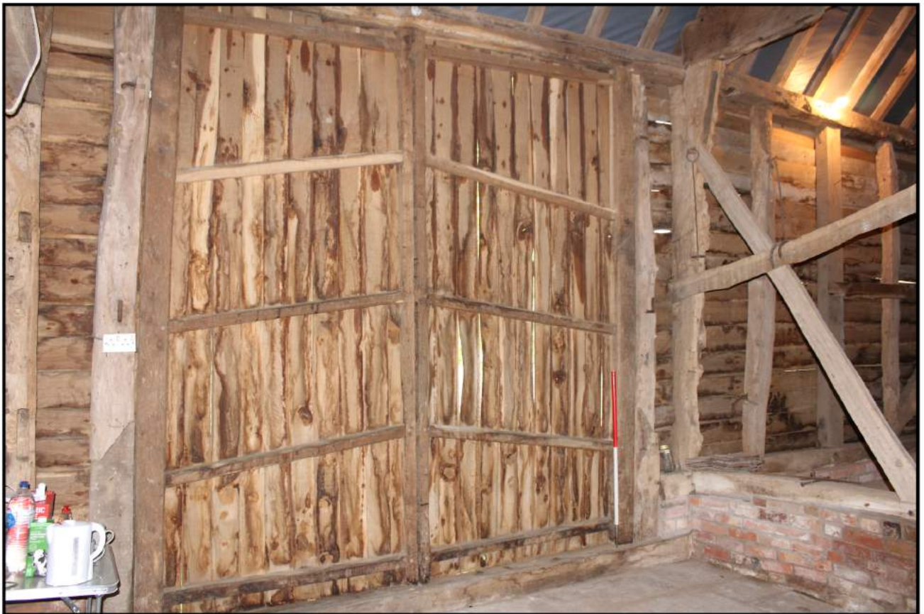
Fig 28: Barn interior; north-west elevation, detail of threshing floor doors
