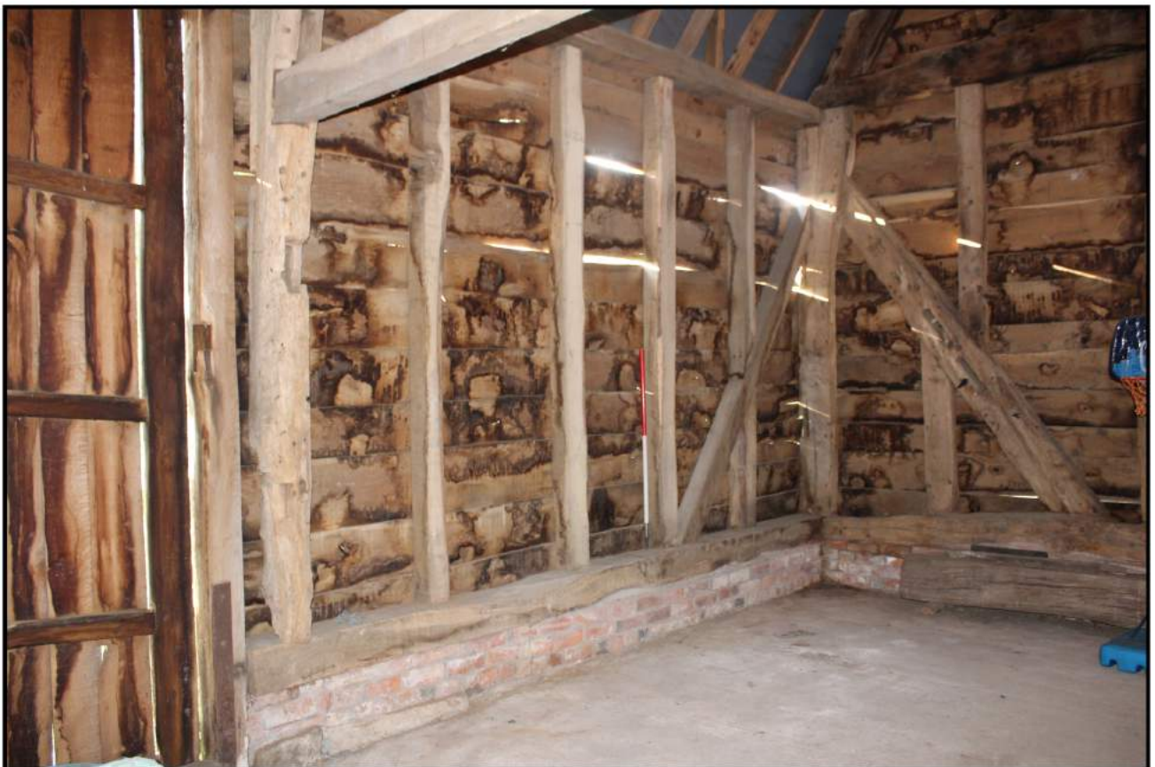
Fig 15: Barn interior; south-west elevation, south-west end
