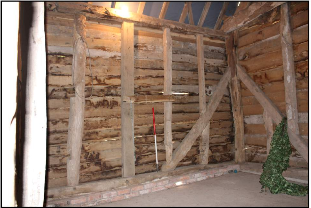
Fig 9: Barn interior; north-west elevation, north-east end
