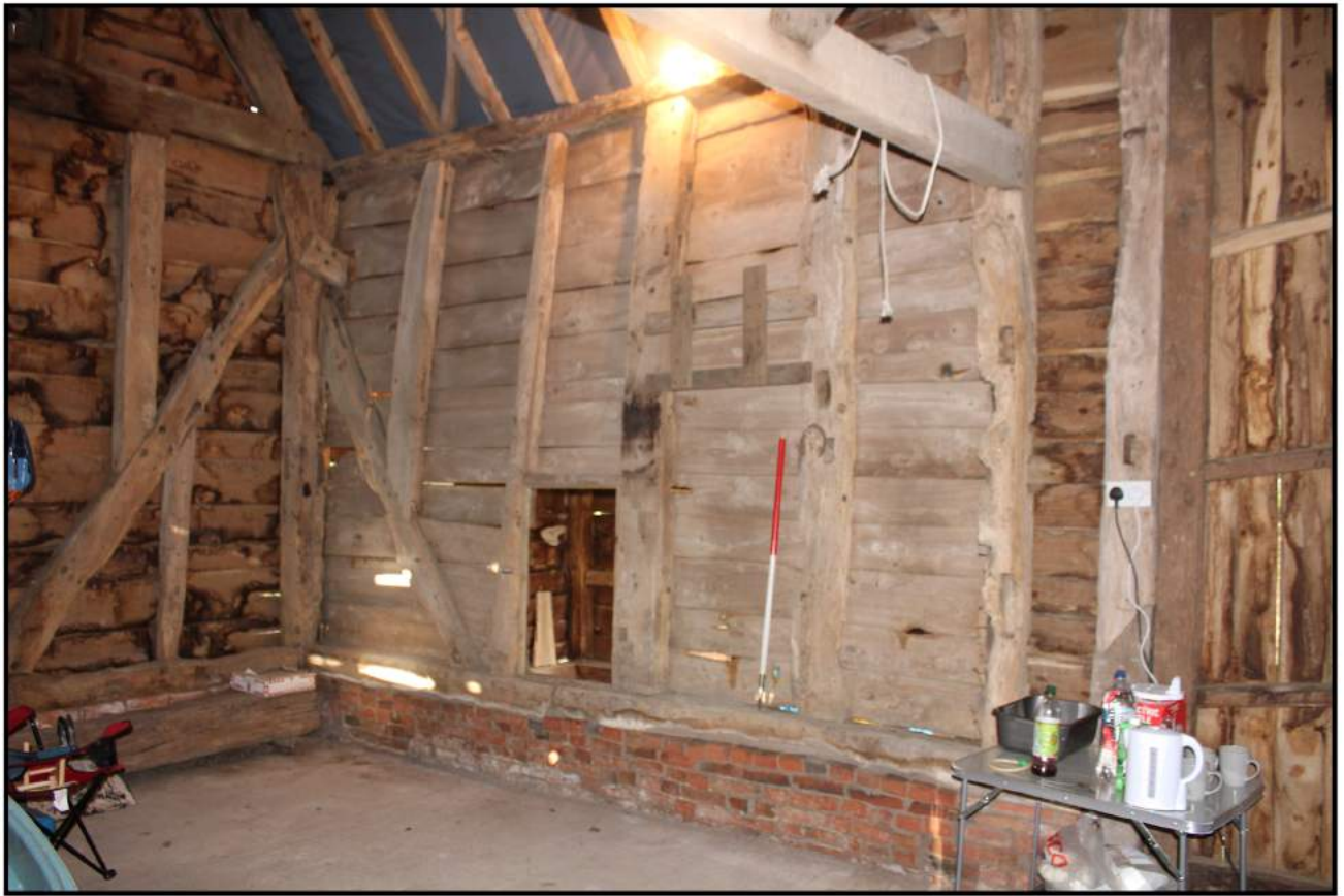
Fig 16: Interior of barn; north-west elevation, south-west end
