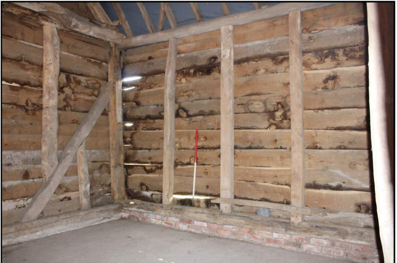
Fig 10: Barn interior; south-east elevation, north-east end
