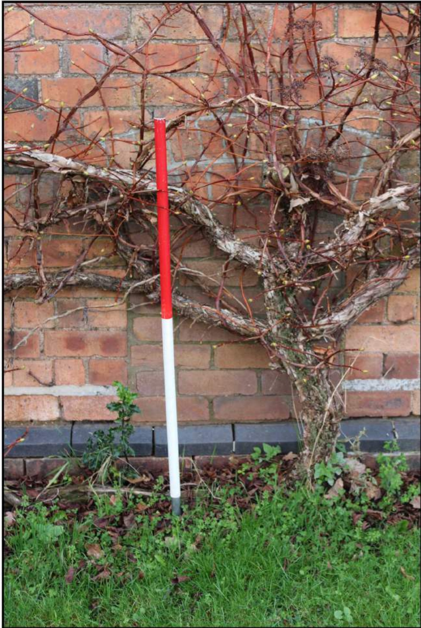
Fig 10: South-east elevation; detail of blocked opening
