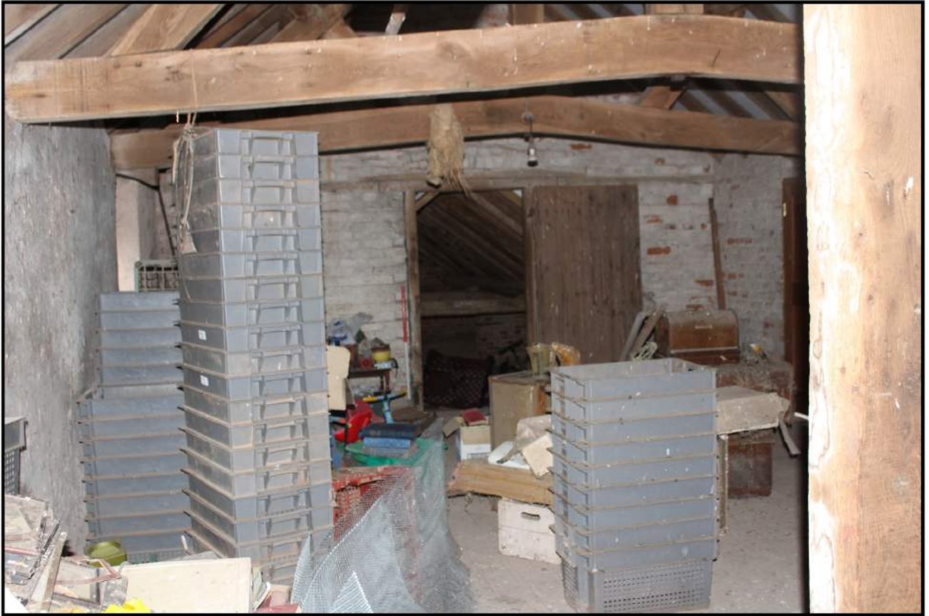
Fig 25: First floor looking towards hop drying area
