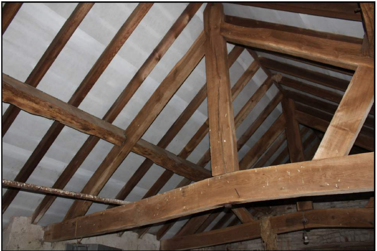
Fig 26: King post roof truss and purlin, showing modern common rafters
