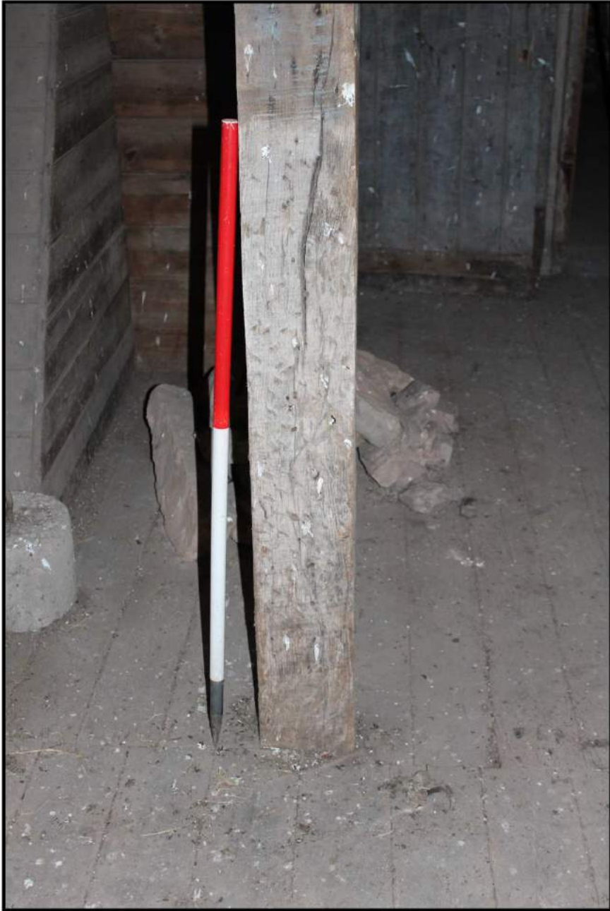
Fig 29: Pecking on lower part of post
