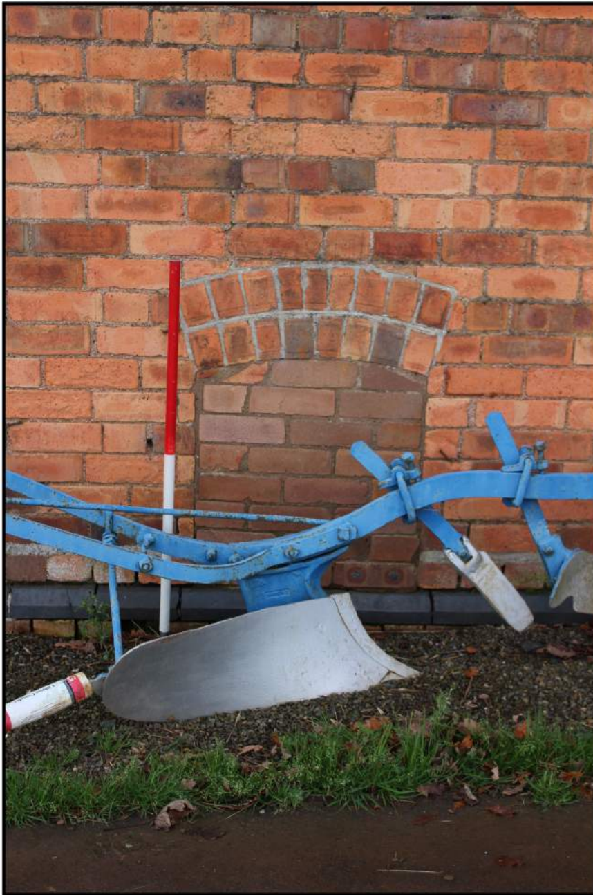
Fig 12: North-east elevation; detail of blocked opening
