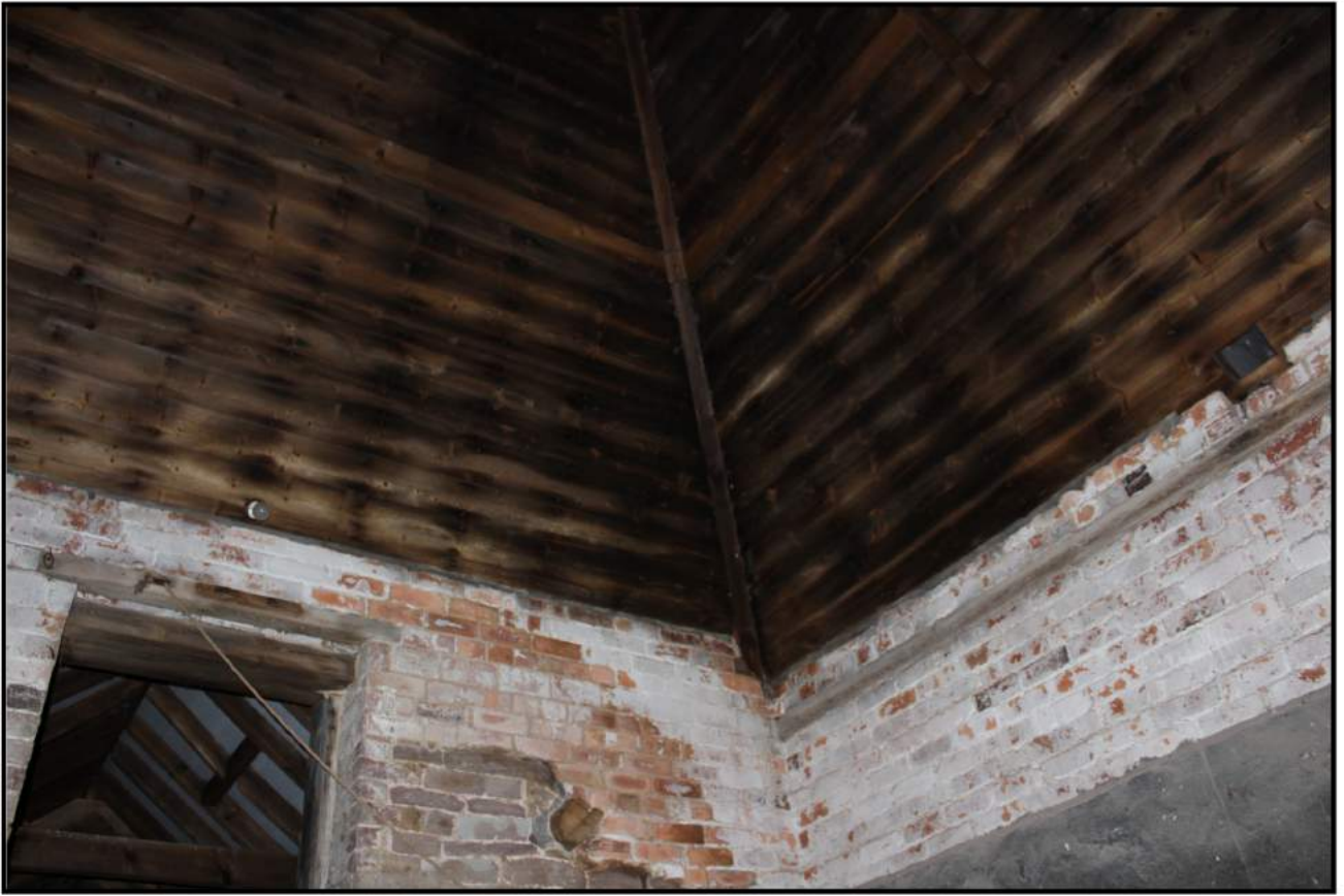
Fig 22: Interior of oast roof showing singed boards
