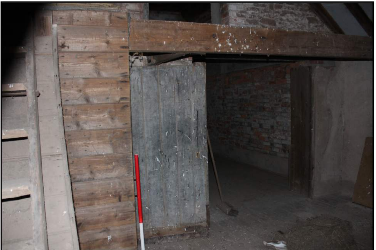
Fig 23: Platform providing access to drying floor door
