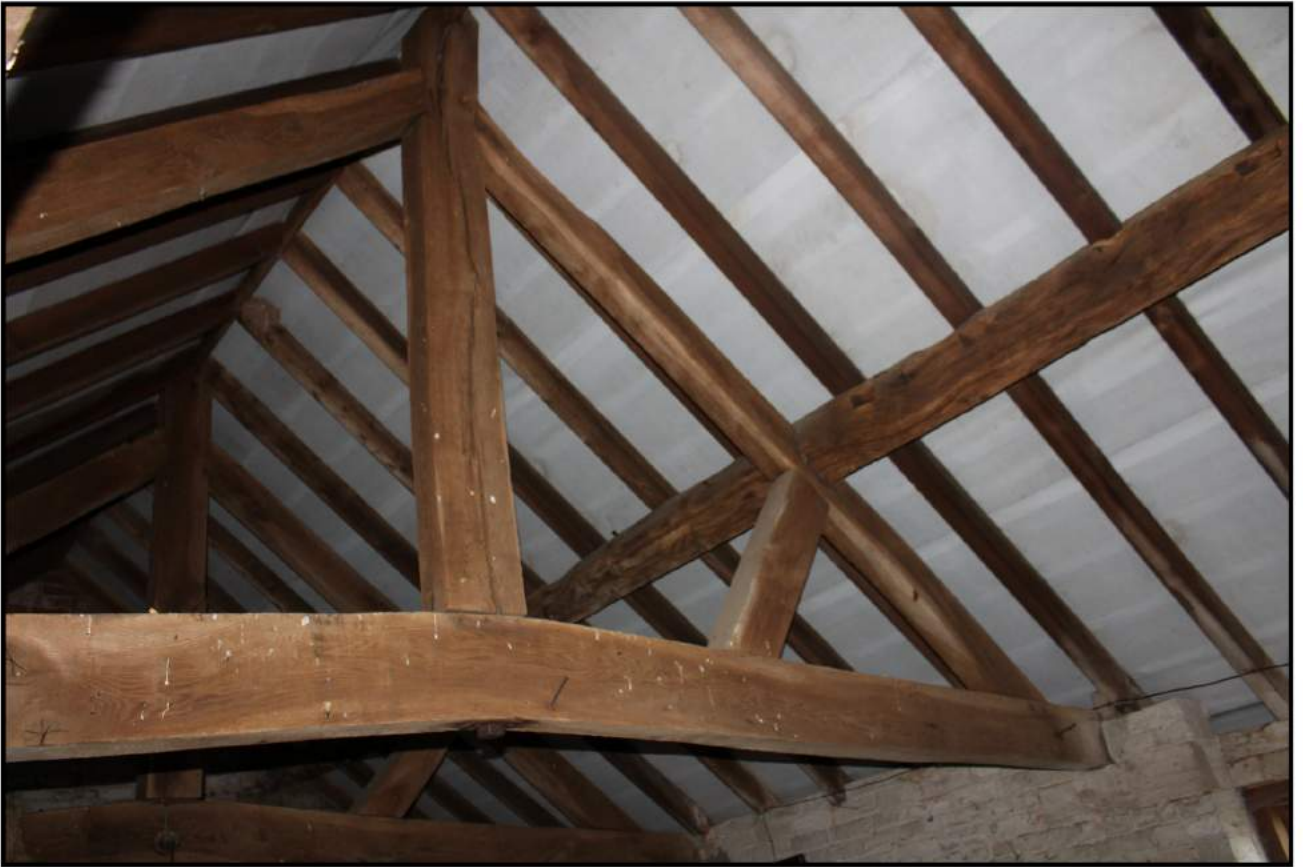
Fig 27: King post roof truss and purlin showing modern common rafters
