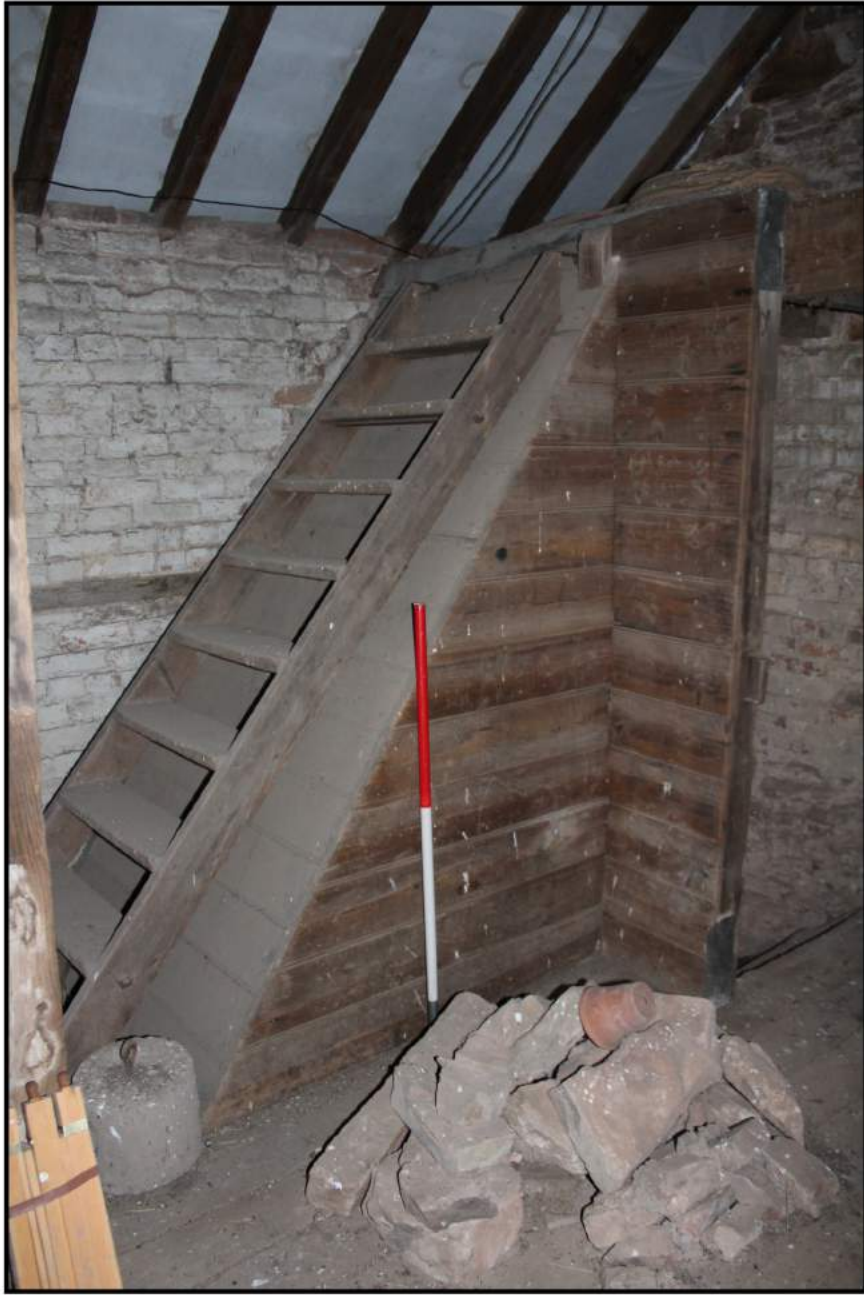
Fig 24: First floor, showing stairs to hop drying floor
