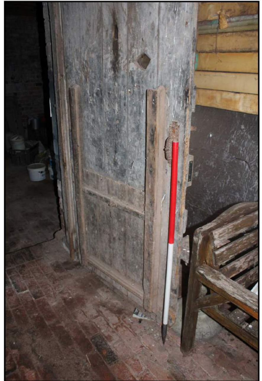
Fig 19: Ground floor, interior; showing door with sliding panel
