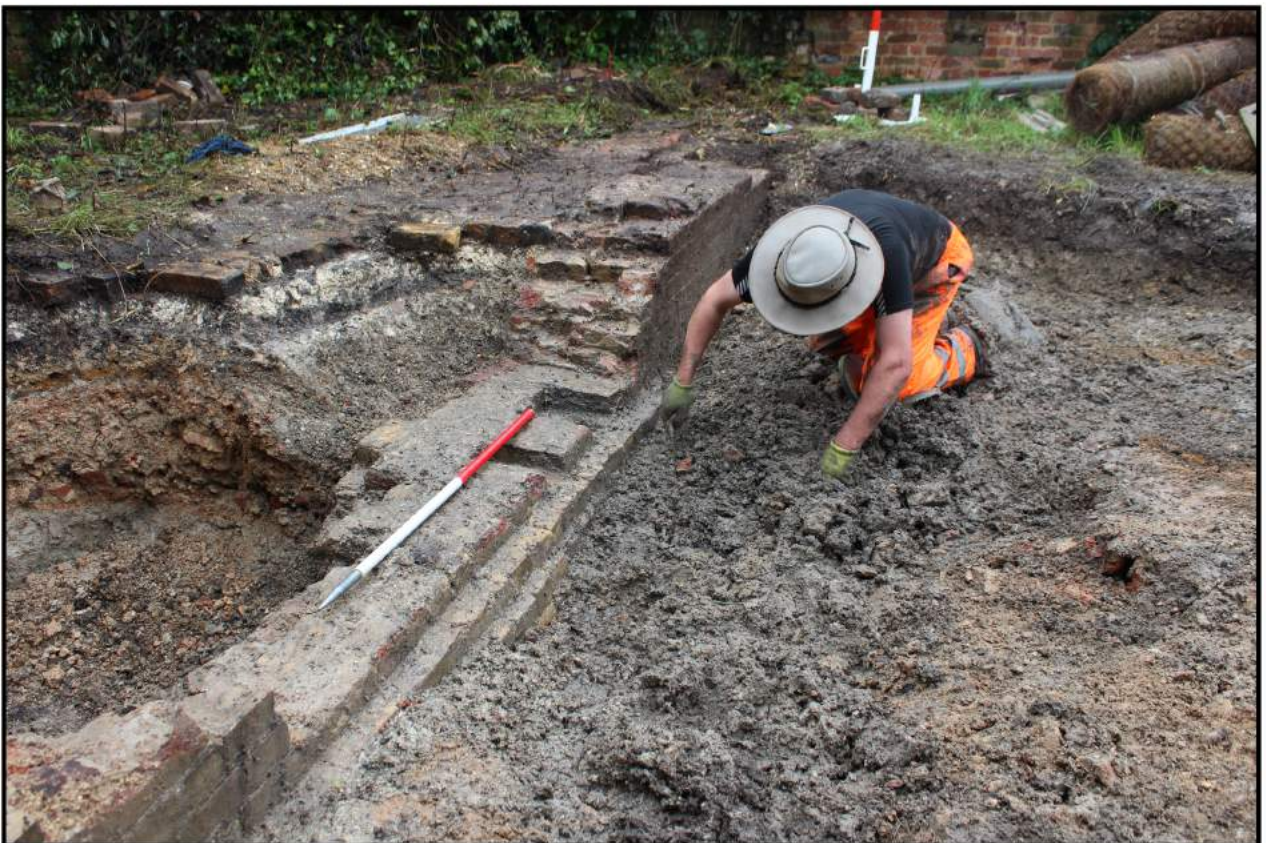
Fig 10: Existing wall, context 007 with stepped footing, context 010, probably same wall as shown on historic mapping, Figs 2.1 and 2.2, scale 1.0m
