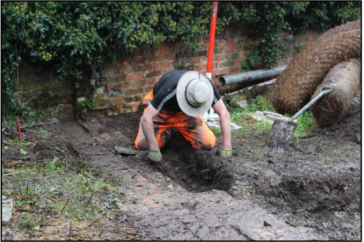
Fig 21: Existing wall, context 007 under excavation
