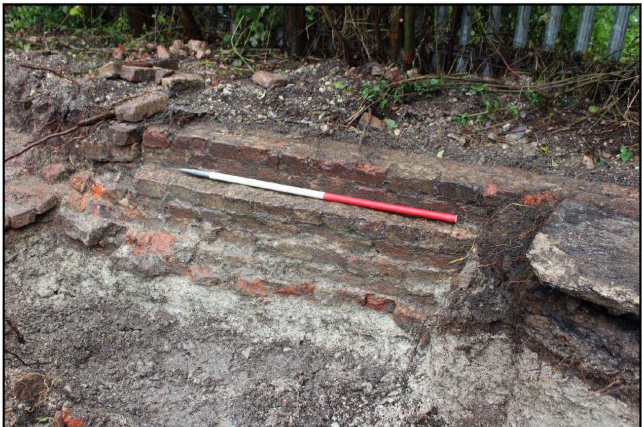
Fig 8: Existing wall; showing stepped footing, context 006, scale 1.0m
