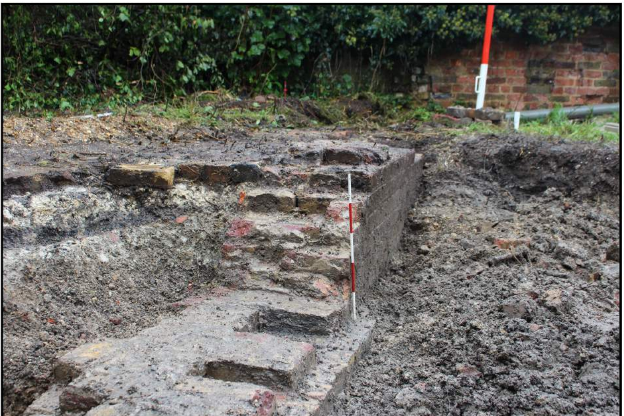
Fig 12: Existing wall; context 007, scale 0.5m
