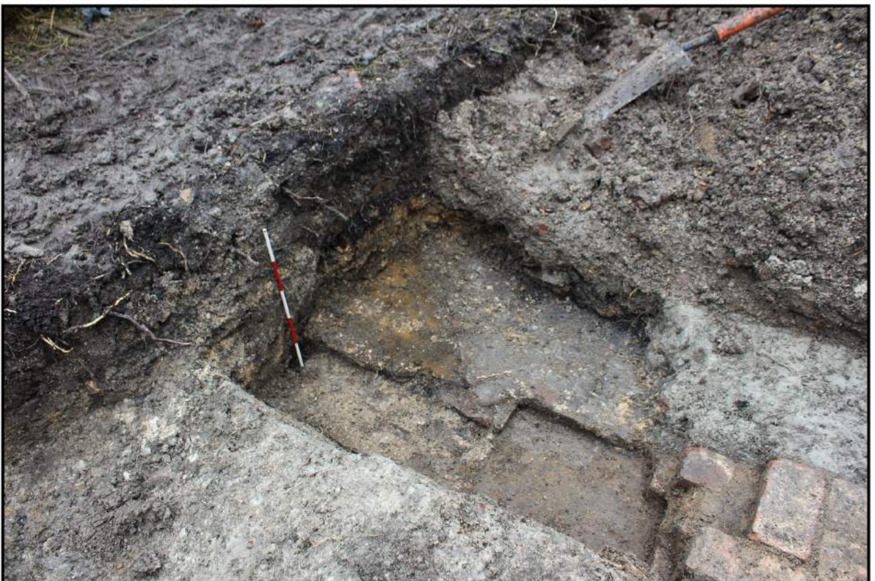
Fig 16: Existing wall, context 003, robbed wall, context 005 and robber trench, context 004; scale 0.5m
