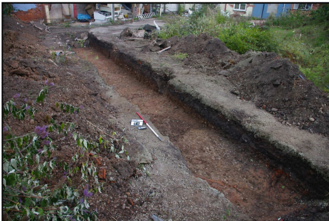
Fig 5: General view of Trench 1
