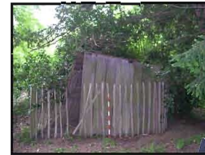
General view of privy
