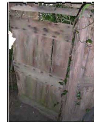
Detail of door
