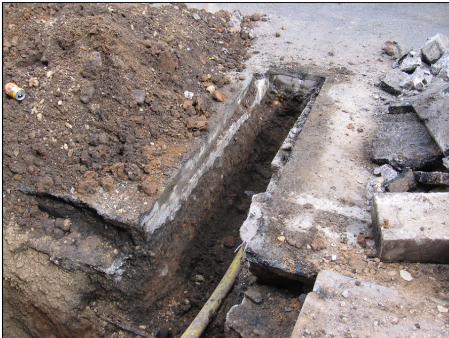
Plate 4 Trench at Section 21, looking north-east
