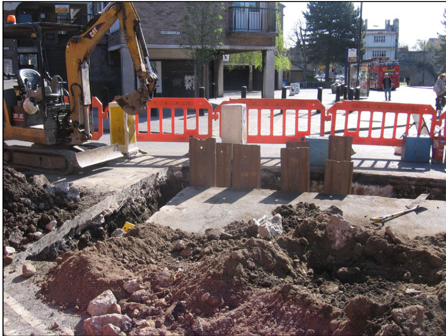
Plate 5 Trench at Section 22, looking east
