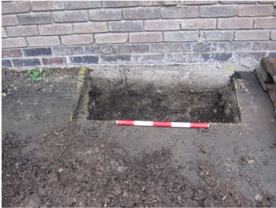
Plate 1 Test pit 1, looking north-west
