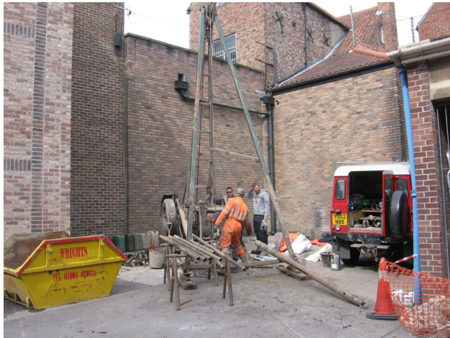
Plate 10 Borehole rig in position of borehole 2, looking west
