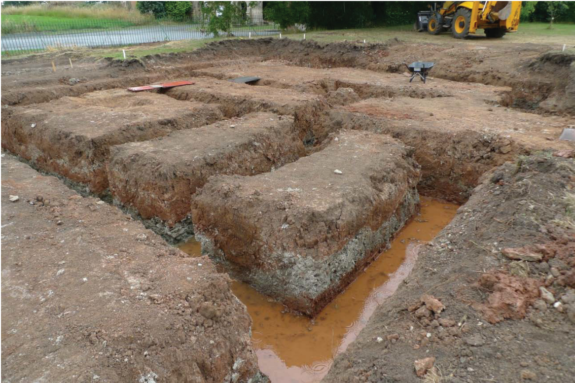
Plate 5 Foundation strip trenches looking towards the castle
