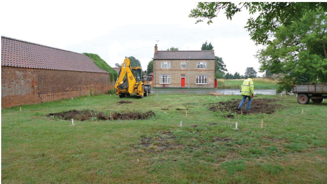
Plate 2 The site before groundworks began, looking south
