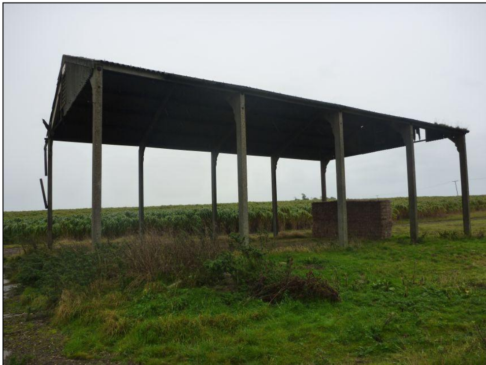
Plate 6 General view of the barn, looking south
